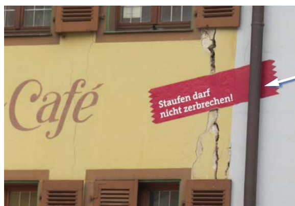
Figure 3: Damage to buildings in the historic town centre of Staufen im Breisgau.
