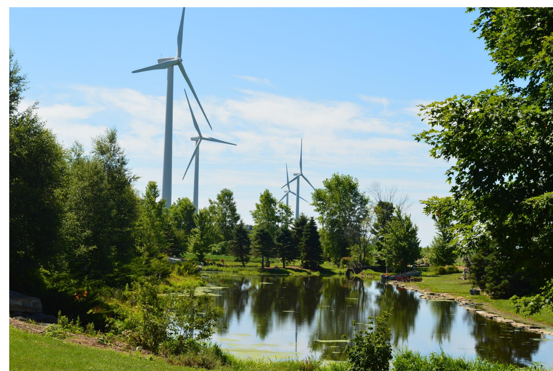
Wind turbines near Port Burwell, Ontario (Erie Shores Wind Farm)
