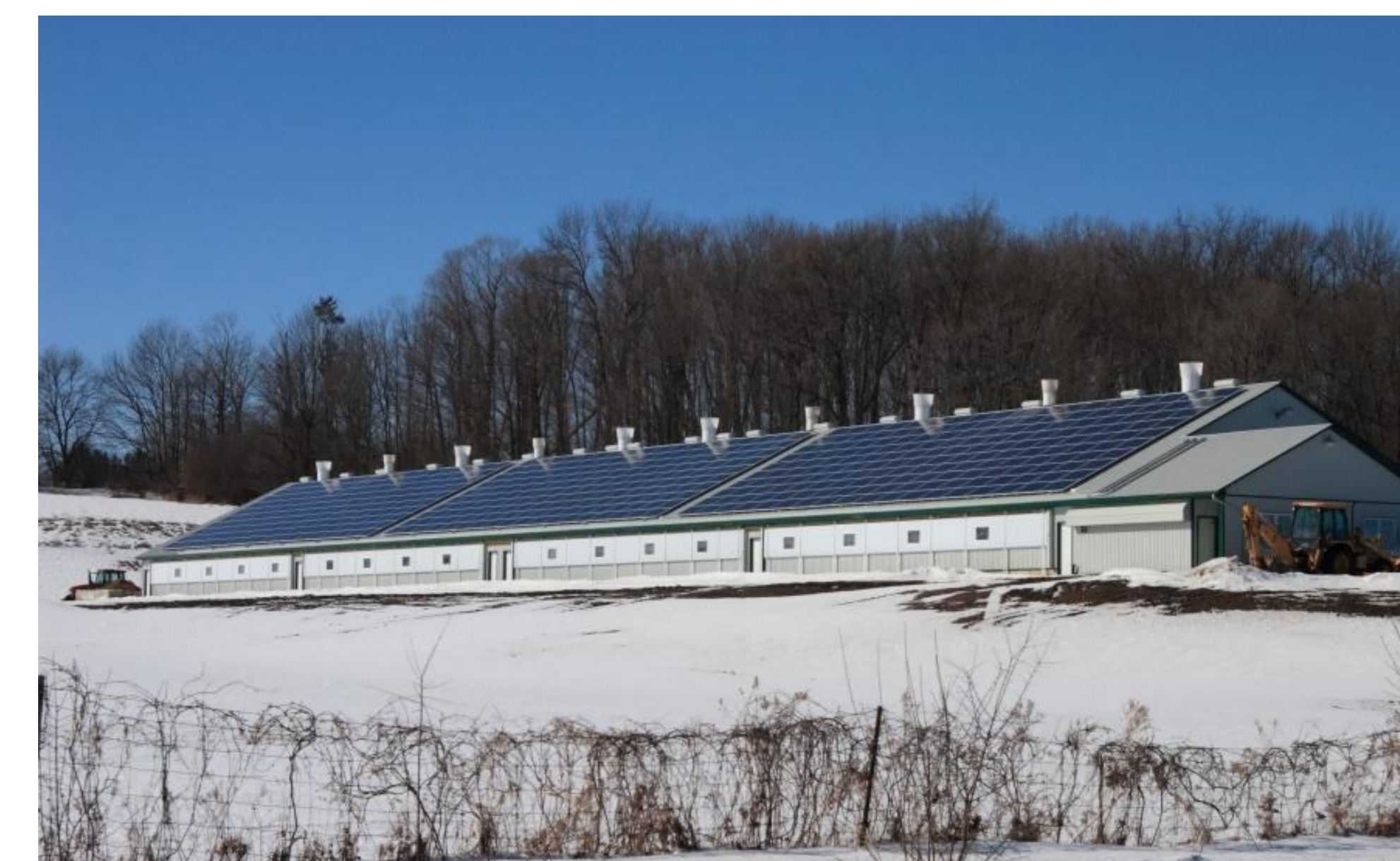
The Yorkshire Valley Barn Solar Project (Source: Generation Solar)
