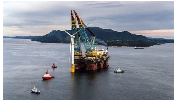
Figure 3d SSCV WTG installation (ref [12])
