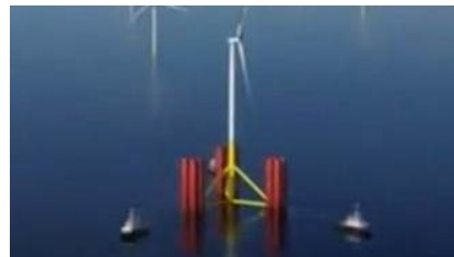
Figure 4a Temporary buoyancy on substructure at end of tow out (ref [14])
