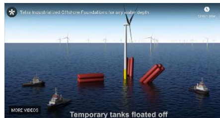
Figure 4b Temporary buoyancy on substructure removed after ballast down. (ref [14])
