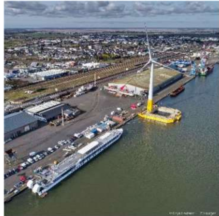
Fit Out Of Turbine
