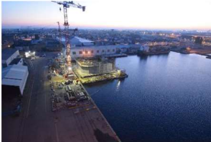
Concrete Substructure Built On Pontoon
