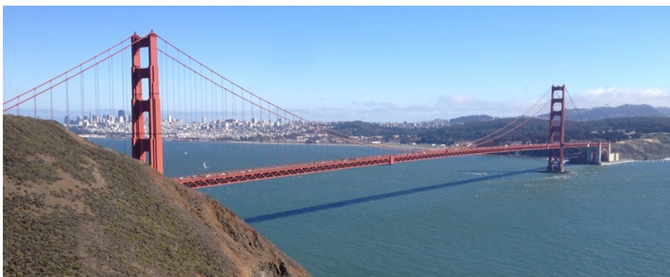
Figure 4 – Steel bridge era: Golden Gate Bridge, United States (1933)
