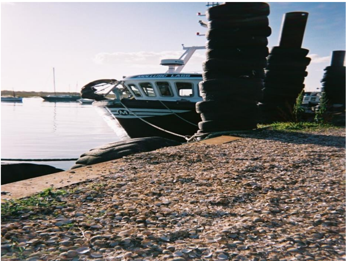
Photograph 13 Completed jetty constructions ( Shram )
