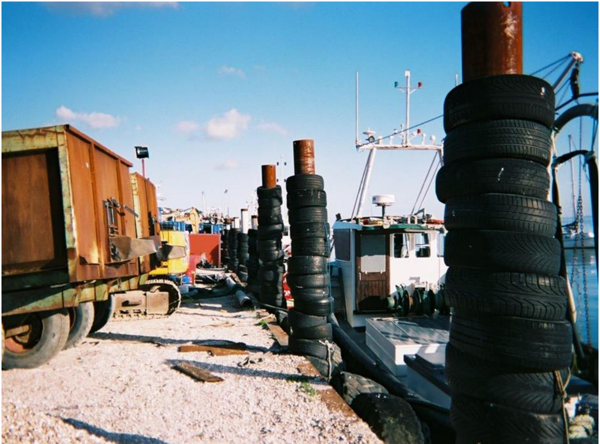
Photograph 12. Completed jetty constructions
