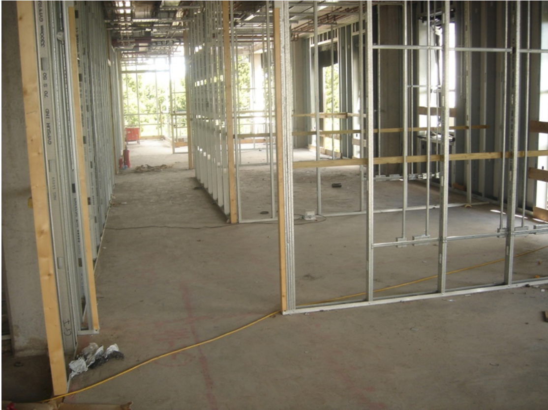
Figure 3: Framing system for internal partitions (Photos: A. Devin)
