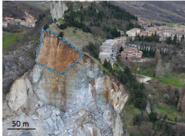
Fig. 4 View of the landslide area from the top, the dashed blue line highlights the discontinuities named SL2.1. Scale is indicative (Photo courtesy STB Romagna)
