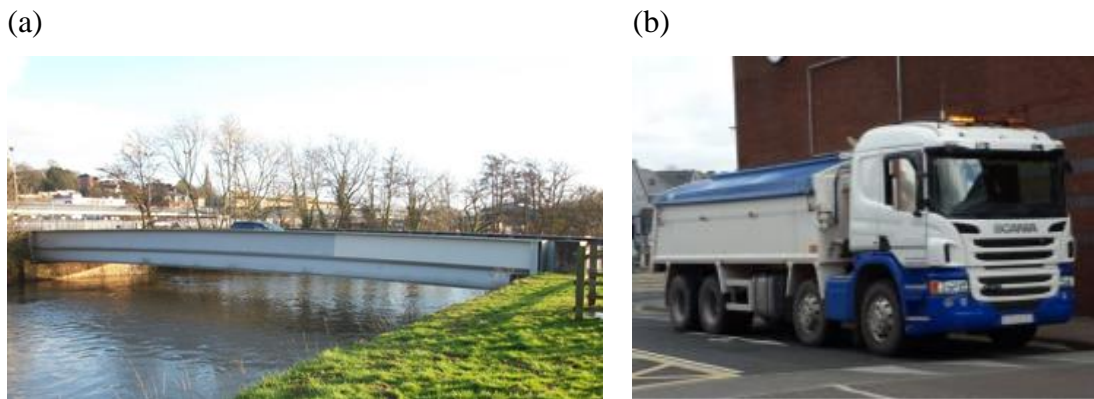
552 Fig. 9: (a) Bridge B elevation; (b) Test truck
