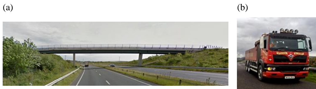
298 Fig. 3: (a) Bridge A elevation (3-span bridge); (b) Truck used in experiment
