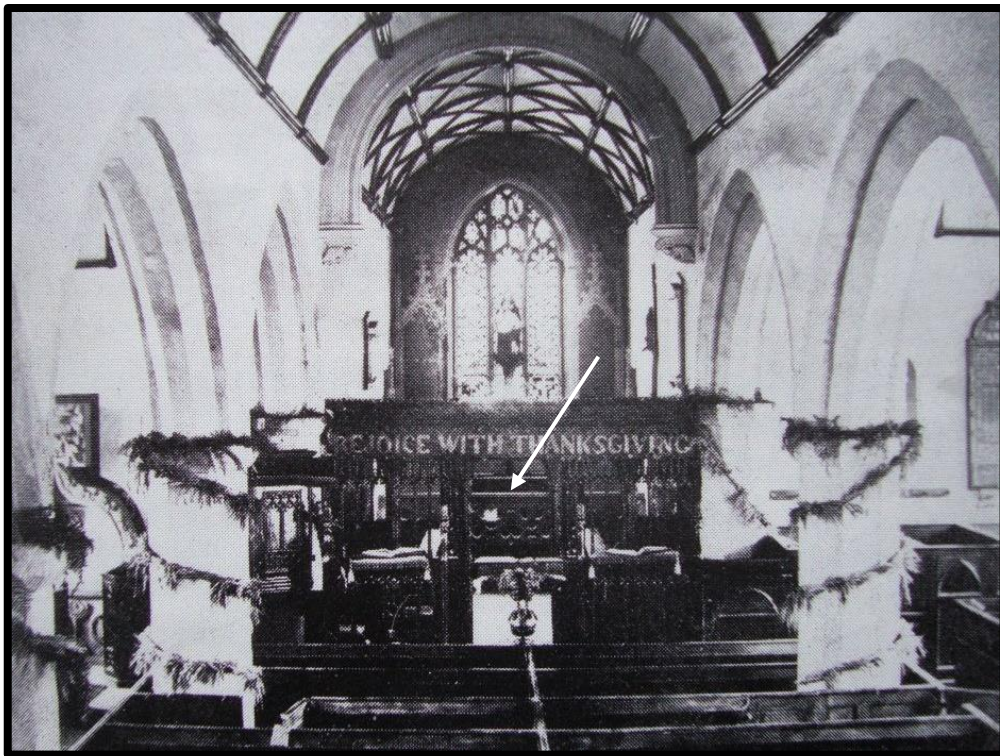
Fig. 245 The interior of Combeinteignhead church before the restoration of 1887, showing an old-fashioned interior with box pews, no central alley, and, remarkably, a stone altar rail (arrowed) crossing the entire sanctuary without interruption (photo in the anonymous Combeinteignhead church guide).
