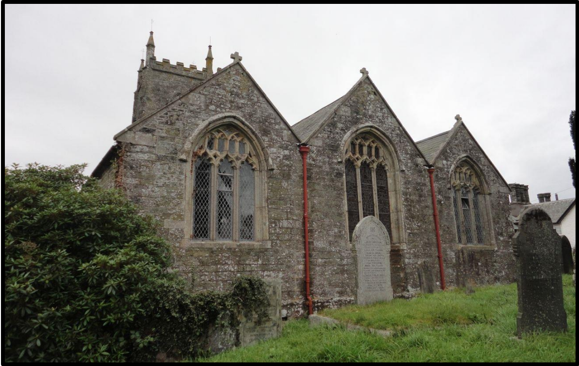
Fig. 238 The east end of the medieval church at Milton Abbot showing the absence of a distinct chancel (RWP Milton Abbot DSC09662).
