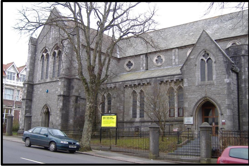
Fig 198 St Michael, Devonport (1843-5) by Benjamin Ferrey, Demolished 2007 (David King).
