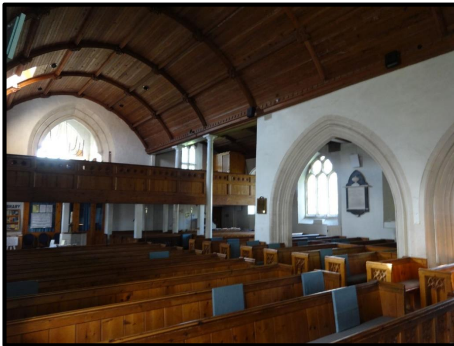
Fig. 152 The interior of the church at Seaton, showing the removal of the arcades and substitution of iron columns. Ashworth's proposal to reinstate the arcades was never carried out (RWP Seaton DSC02900).
