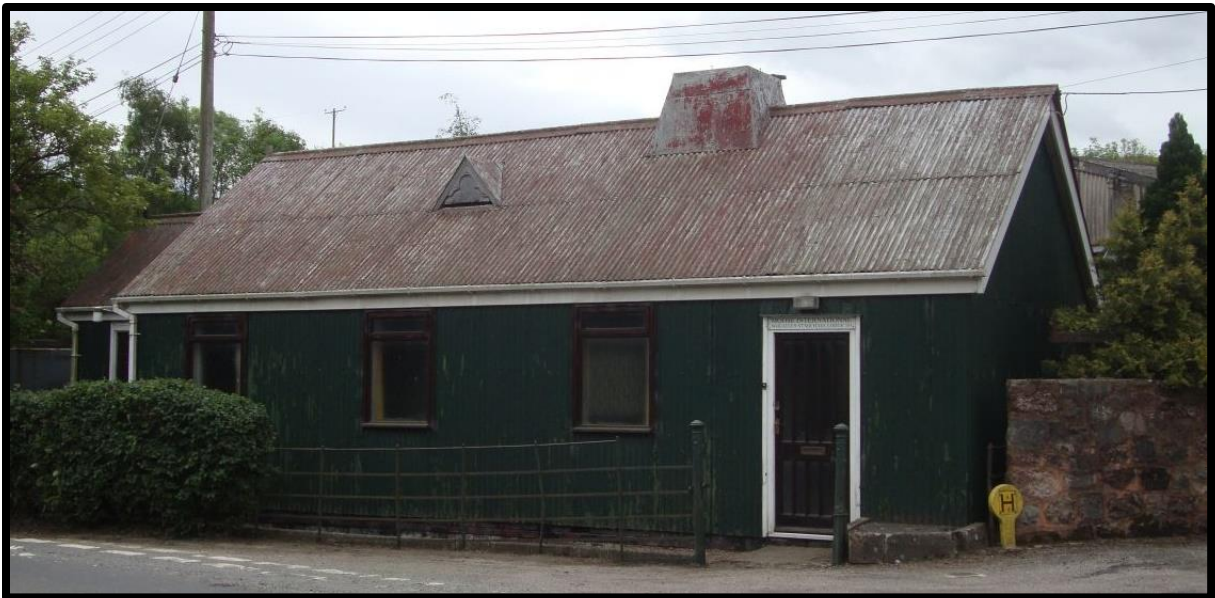
Fig. 22 The corrugated iron Mission Chapel at Wheatley in the parish of Alphington, Devon, the base of the spirelet remains on the roof (RWP Wheatley DSC04966).
