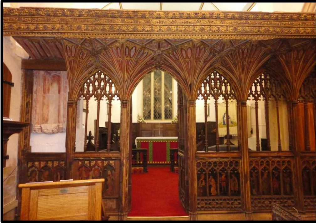
Fig 57 The rood Screen at Plymtree, showing the northern bay crudely adapted around an earlier image niche, suggesting that the screen was brought here in the 16th century, from elsewhere (RWP Plymtree DSC09645).
