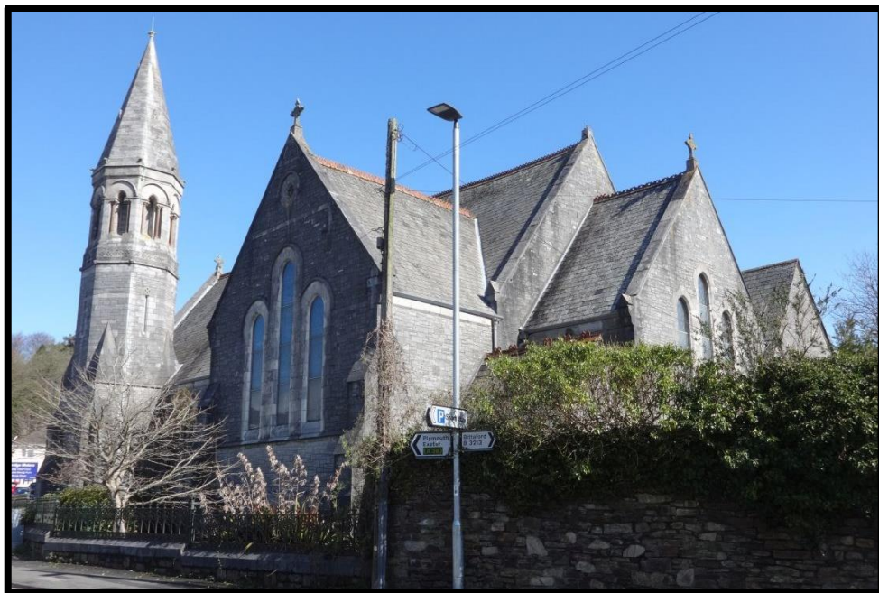
Fig. 162 The Methodist Church at Ivybridge (1874) by Norman & Hine, showing developed Gothic details and asymmetrical planning (RWP Ivybridge Methodist Church DSC093).
