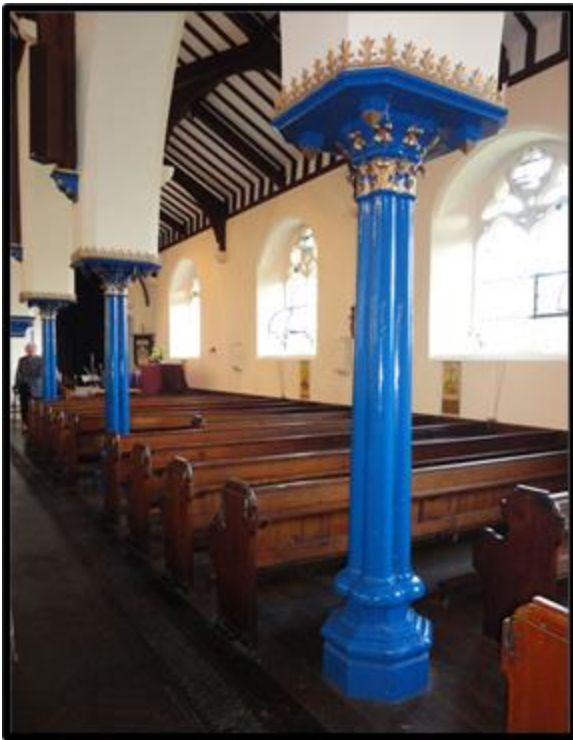
Fig. 209 The iron columns at Christchurch, Ellacombe (RWP Ellacombe; Torquay Christchurch DSC06226).
