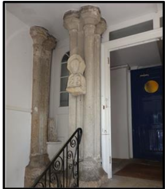
Fig. 75 Reused monolithic pillars from the medieval arcades at Stoke Damarel (RWP Devonport Stoke Damarel DSC00058).
