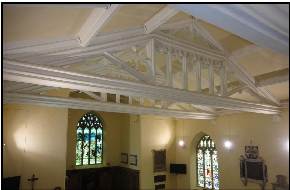
Fig. 87 Stoke Canon: the rebuilt church of 1835 showing the broad nave spanned by an un-archaeological Gothic queen-post roof but with carefully replicated perpendicular window tracery (RWP Stoke Canon DSC00230).
