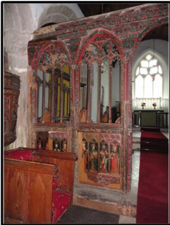
Fig. 302 The rood screen at Chivelstone, showing the damage following the loss of the rood loft and basic wear and tear (RWP Chivelstone DSC1842).
