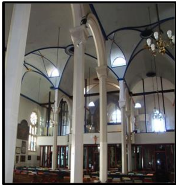
Fig. 99 The remarkably un-archaeological interior of St Michael's, with timber columns crowned with cushion capitals (RWP Teignmouth St Michael DSC00293).
