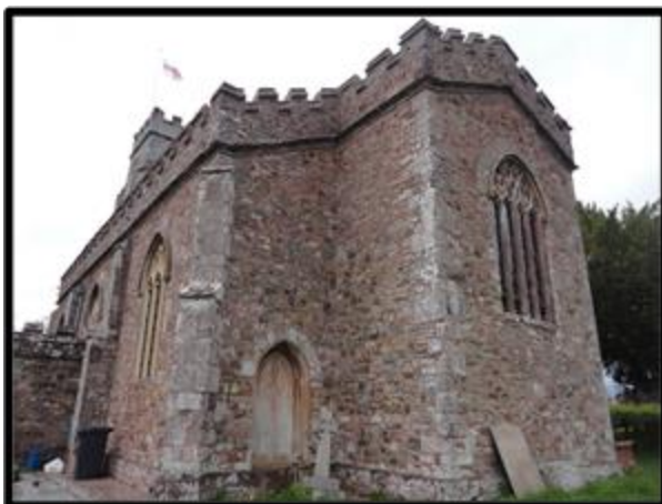
Fig. 169 The church at Stoke Canon from the east, showing relatively accurate details applied to an inappropriate bulk (RWP Stoke Canon DSC00142).
