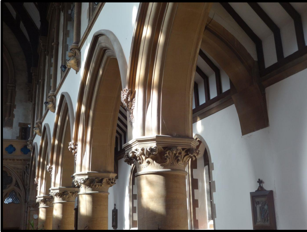
Fig. 205 Early French style 'Muscular Gothic' crocketed capitals at St Michael's Mount Dinham, Exeter (1864-8) by M. Rohde-Hawkins (RWP Exeter St Michael's DSC06722).
