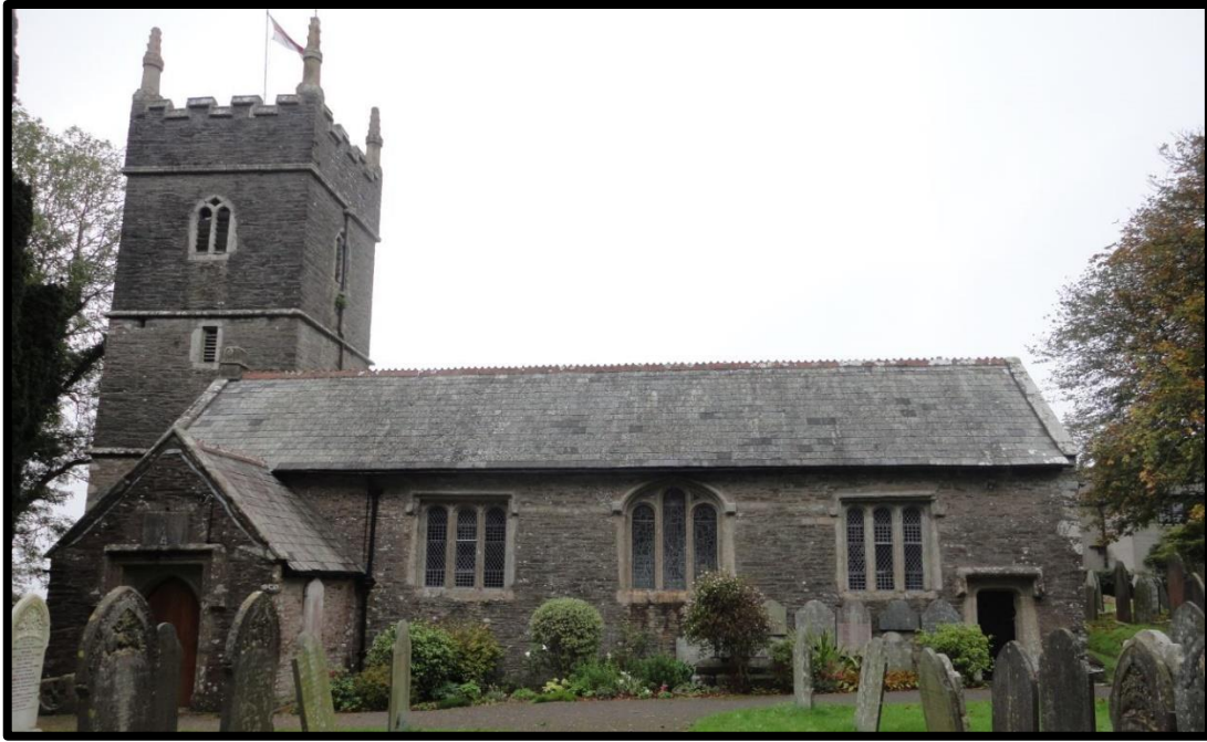
Fig. 55 The late 16th-century church at St Budeaux, near Plymouth, showing the south aisle. The church has three equal aisles, with doorways at all four corners (RWP St Budeaux DSC09510).
