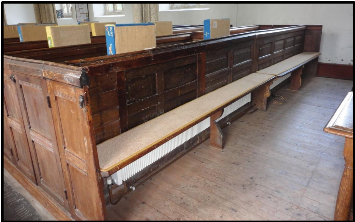
Fig. 311 Reused sections of box pews at Halwell, now partially removed, incorporating joinery of at least three periods. (RWP Halwell DSC04642).
