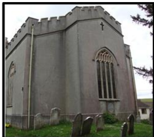
Fig. 170 The church at Ide from the east, showing perpendicular tracery mixed with Georgian false ashlar-work (RWP Ide DSC04798).
