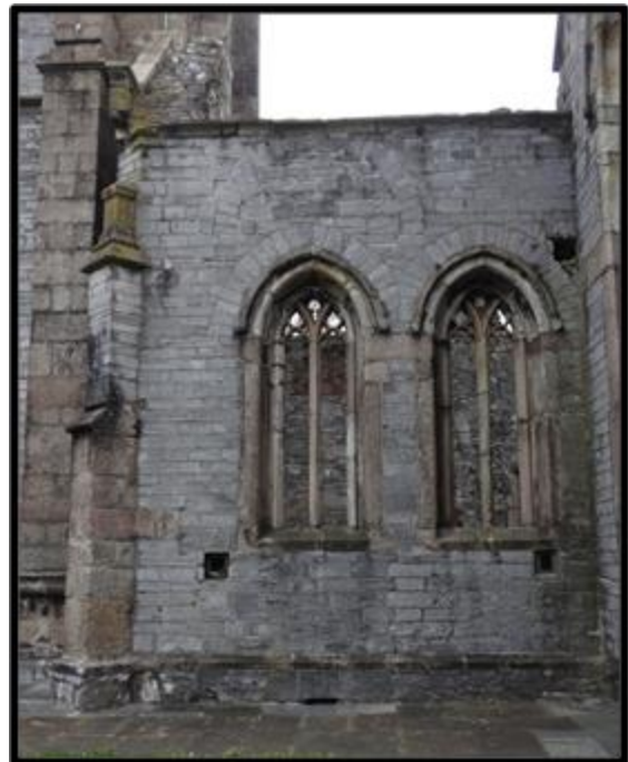
Fig. 61 Anomalous round-headed arch in the south-western part of the nave at Charles, Plymouth, possibly for an earlier fenestration scheme (RWP Plymouth; Charles DSC06764).
