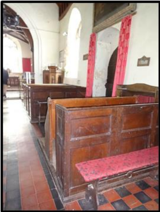
Fig 251 A democratised interior; the removal of box pew doors at Stockleigh English to cheaply create open benches (RWP Stockleigh English DSC01977).
