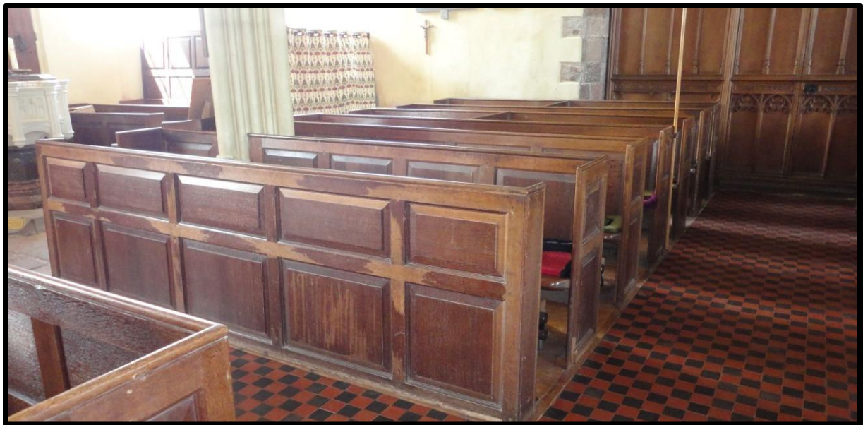
Fig. 13 Reset box pew material at Cheriton Fitzpaine, retained for use as open benches following the restoration of 1883-5 by James Crocker of Exeter (RWP Cheriton Fitzpaine DSC04679).
