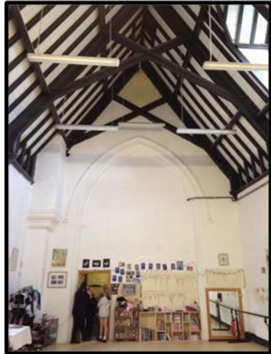
Fig. 230 The school-chapel built for St Peter’s parish, Plymouth (1862), by Roger Elliott (later The Good Shepherd) showing the chancel arch (RWP Stonehouse The Good Shepherd DSC08894).
