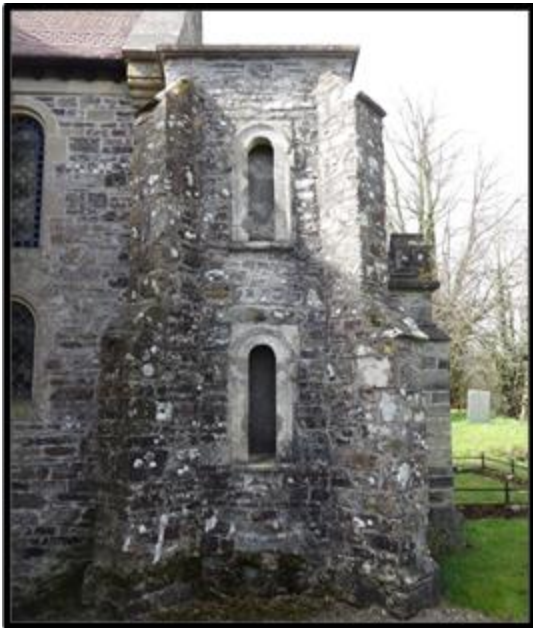
Fig 80 Part of the church at Filleigh (1732) showing one of the former towers of the false façade (RWP Filleigh DSC00355).
