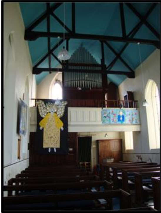
Fig 295 The singing gallery at Chudleigh Knighton, complete with organ (RWP Chudleigh Knighton DSC02487).
