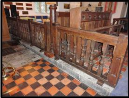
Fig 249 The 17th-century altar rails at Horwood reconfigured as a chancel screen (RWP Horwood DSC03936).
