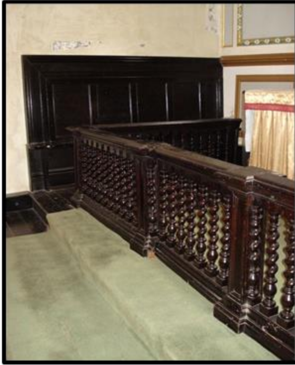
Fig 119 Communicants benches and rails of the late 17th century at St Martin, Exeter (RWP Exeter; St Martin DSC03365).
