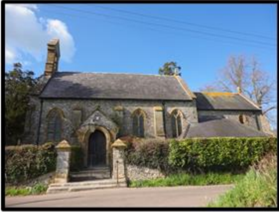
Fig. 222 The small rural church of All Saints, Axminster (1840), by Benjamin Ferrey (RWP All Saints DSC09405).
