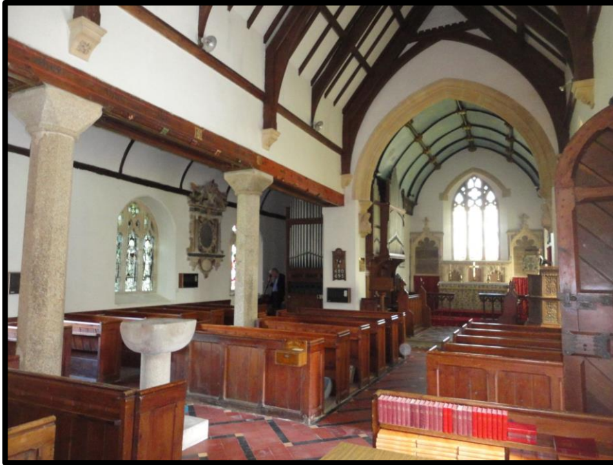
Fig. 151 The interior of the church at Alverdiscott, showing the replacement of the arcades (RWP Alverdiscott DSC09035).
