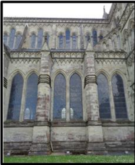
Fig. 181 Salisbury Cathedral, detail of the aisles (RWP Salisbury DSC01651).
