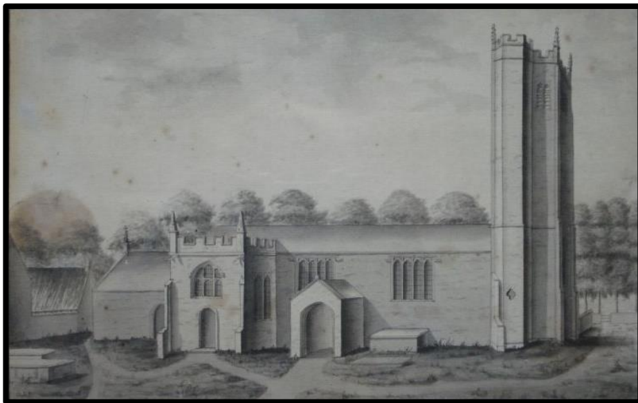
Fig 58 The north side of St Thomas' Church by Exeter before early 19th-century alterations, showing 17th-century Gothic details (Anonymous drawing dated 1765, possibly by Matthew Blackmore?, now held in the Church vestry at St Thomas'; RWP Exeter St Thomas, DSC00308).
