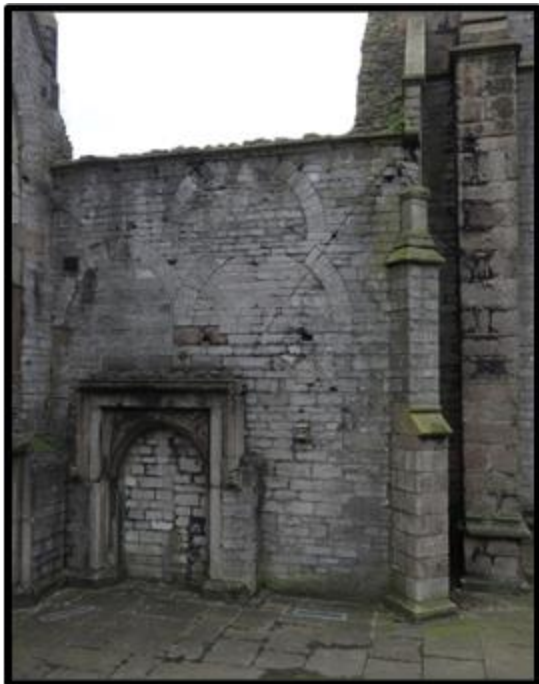
Fig. 60 Anomalous round-headed arches in the north-western part of the nave at Charles, Plymouth, possibly for an earlier fenestration scheme (RWP Plymouth; Charles DSC06747).
