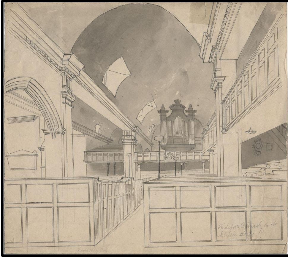
Fig 14 The interior of Bideford Church in c.1865, drawn by Edward Ashworth before rebuilding, showing the impact of inserting additional galleries within a medieval structure (SWHC WSL P&D 05509).
