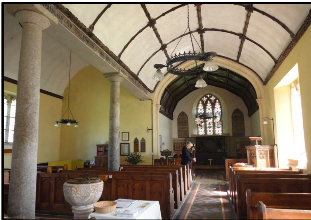
Fig. 150 The interior of the church at Highampton, showing the replacement of the arcades in the Georgian period to create an auditory space (RWP Highampton DSC05488).
