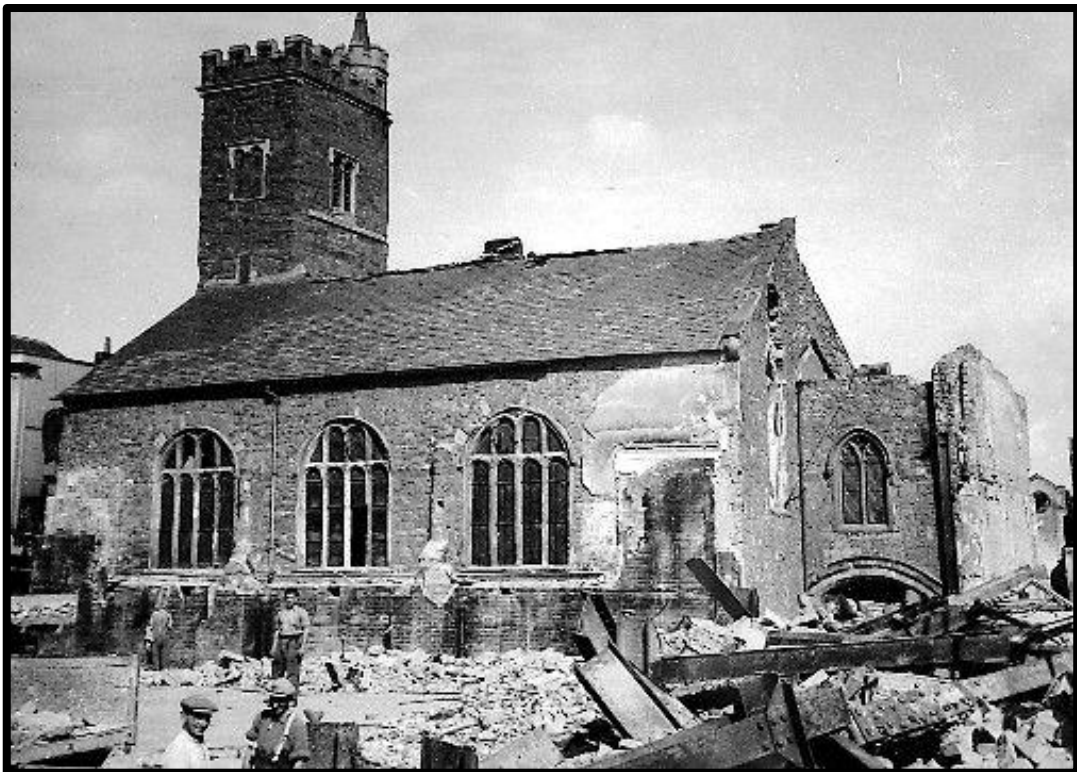
Fig. 70 The south side of St Stephen after the blitz, showing the 17th-century window tracery, now removed (EA War-cat-500).
