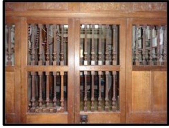
Fig. 250 18th-century altar rails reused in the tower screen at Dartington (RWP Dartington DSC05718).
