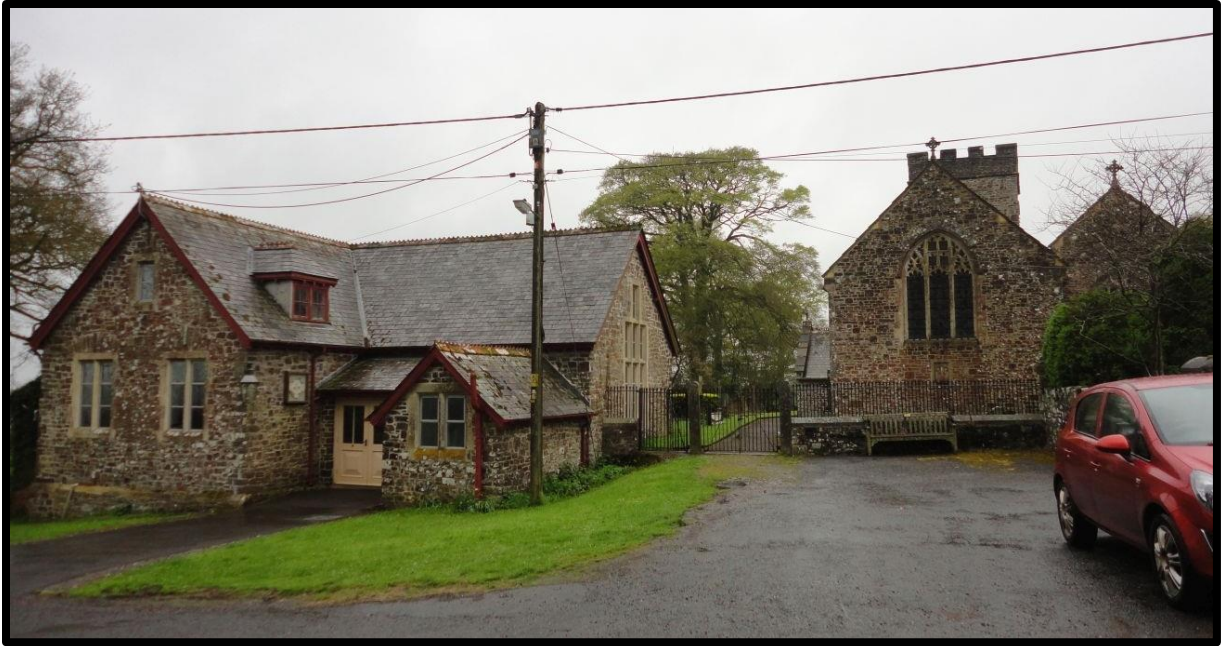
Fig. 21 Rose Ash, Devon; the proximity of the ancient parish church and the schools. Two school buildings survive, both adjoining entrances to the churchyard. The National School founded in 1848 was later succeeded by a Board School in 1877, but proximity to the church clearly remained important (RWP Rose Ash DSC04450).
