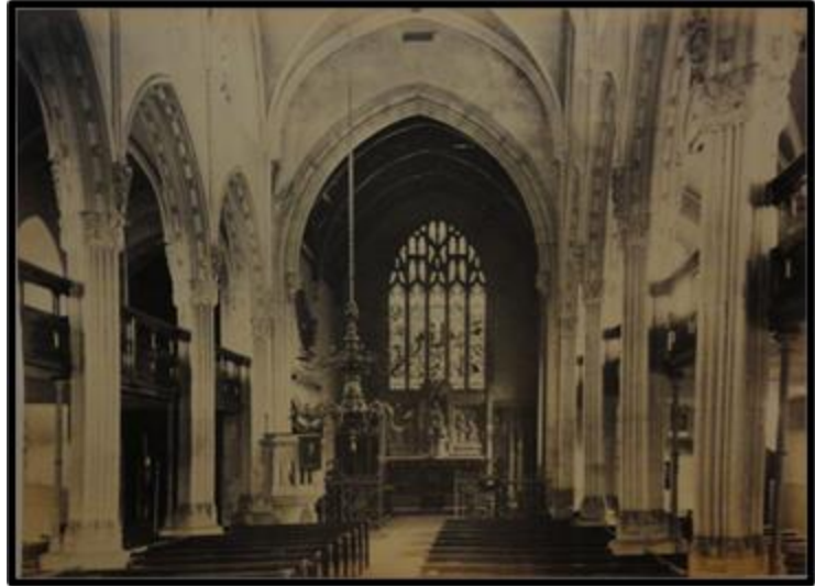
Fig 105 The interior of St Sidwell before its destruction in 1942, showing the reused medieval arcades and the careful accommodation of the galleries as subordinate to them. The chancel is a later addition (D&EI 1870 ROG).
