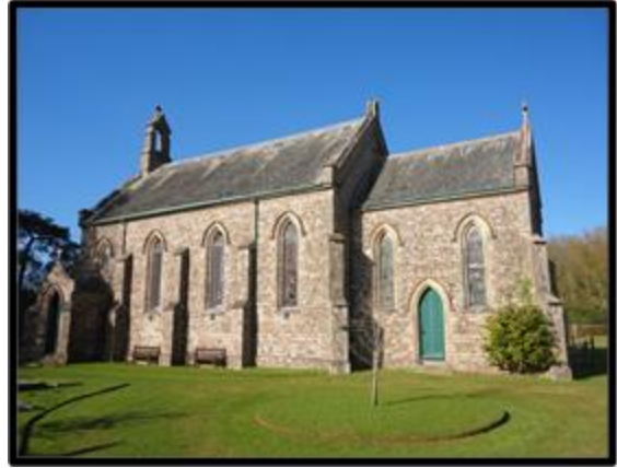
Fig. 223 The similar and very early church at Escot (1837) by Henry Roberts (RWP Escot DSC09097).
