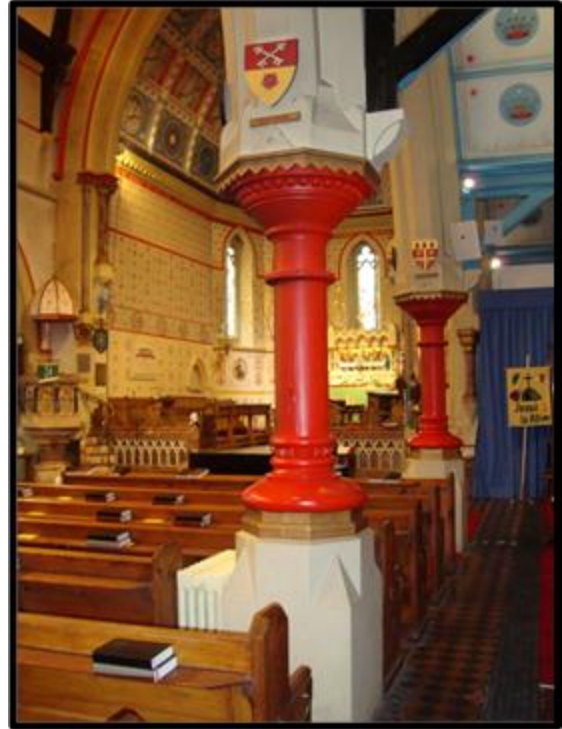
Fig. 208 The iron columns at St Luke, Torquay (RWP Torquay St Luke DSC08616).
