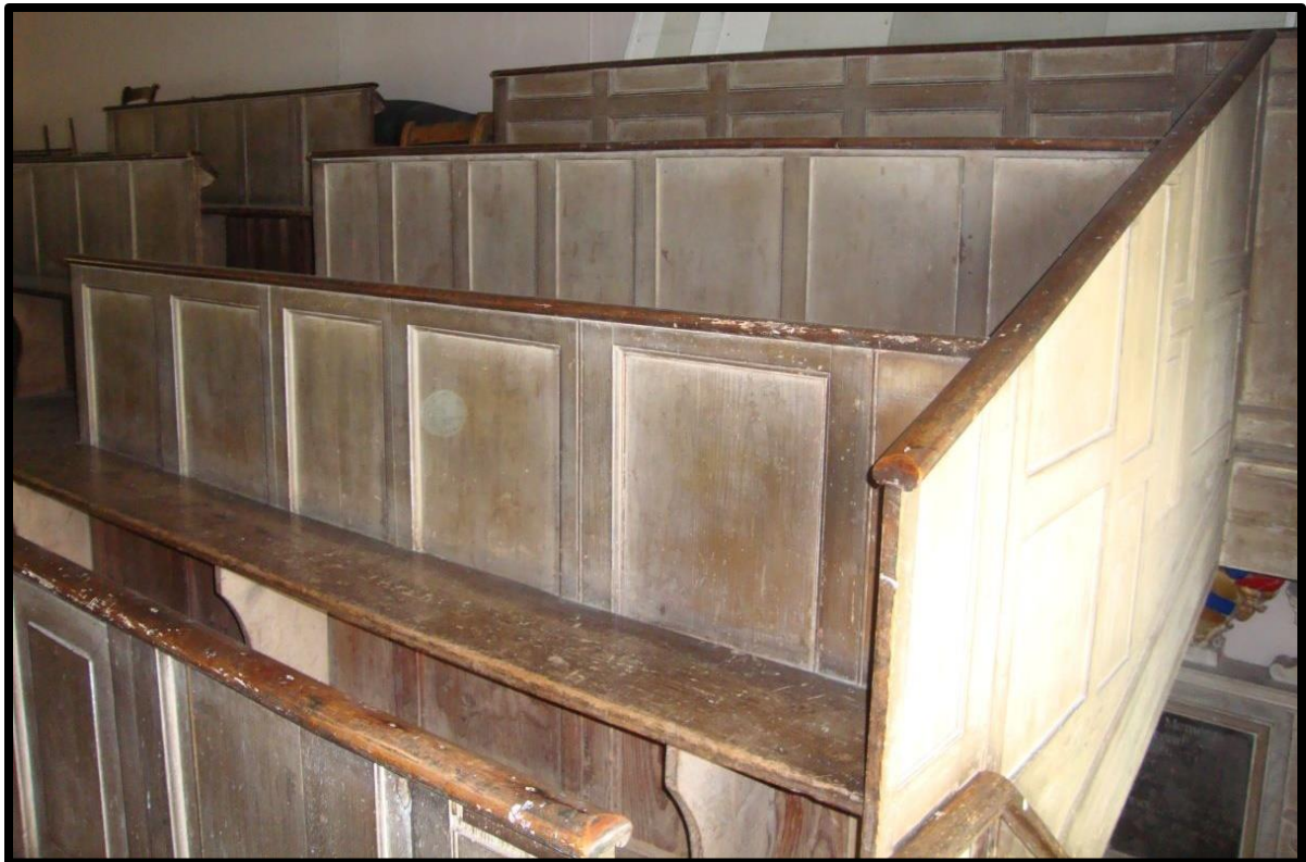
Fig. 147 The remains of reused box pews in the gallery at Ide, incorporating raised-fielded (foreground) large-fielded and smaller-fielded panels, reused from a complex interior with many phases of Georgian intervention (RWP Ide DSC04827)
