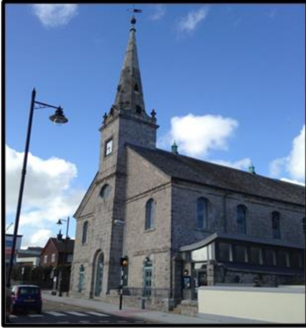
Fig 78 St Aubyn's Church , Devonport (1771) (RWP Devonport; St Aubyn 087).
