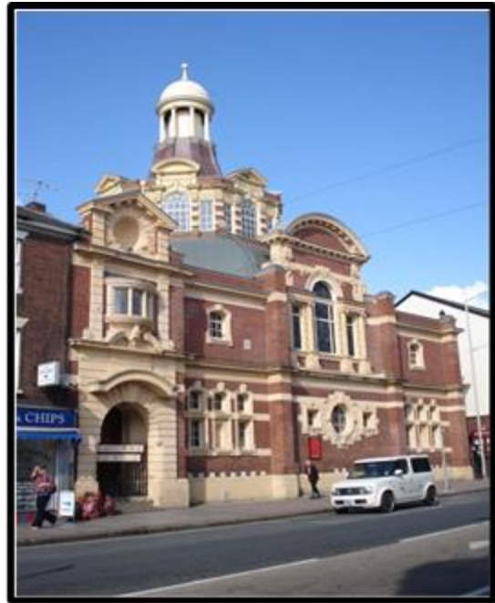
Fig 10 The Wesleyan Methodist Chapel in Sidwell Street, Exeter (Frederick Commin, 1905), built in reinforced concrete on the 'Cottancin System' in the Roman Baroque style (RWP Exeter St Sidwell's Methodist DSC03210).
