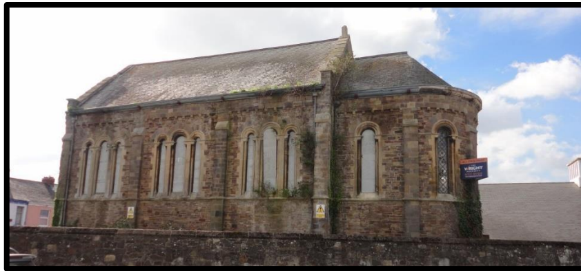
Fig.176 The Immaculate Conception RC Chapel at Barnstaple (1842-5) An accomplished essay in Romanesque, whoever its architect (RWP Barnstaple Immaculate Conception DSC01720).
