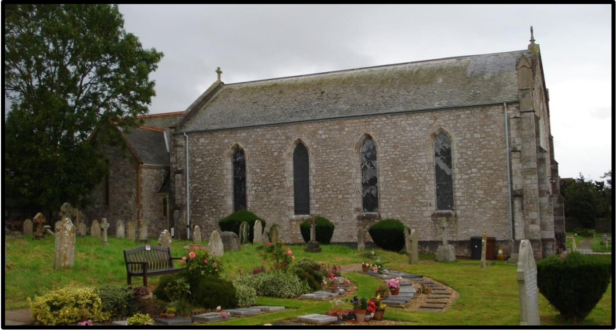
Fig. 17 The simple pre-ecclesiological Gothic church at Countess Wear (1838), designed by Henry Lloyd in the 'lancet style' showing the most basic form of a Gothic-revival church. The cupola for the bell has been removed, the chancel (left) is a later addition (RWP Exeter Countess Wear DSC00325).
