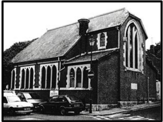
Fig. 237 St Matthias school-chapel at Amity Place, Plymouth (1891), by D. Bellamy, shortly before its demolition in 1996 (Author, EA Archives 1996).
