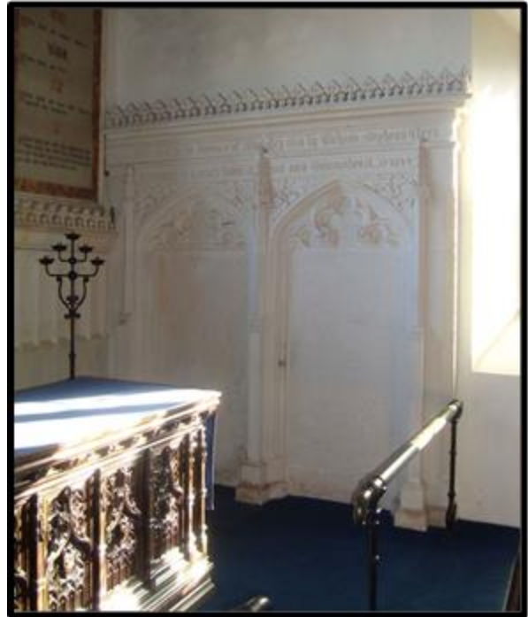
Fig 292 The Sedilia at Holcombe Burnell (RWP Holcombe Burnell ).
