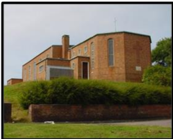
Fig. 35 St Aidan, Ernesettle, Plymouth (now demolished), a post-war suburban church in the monumental tradition (David King collection).
