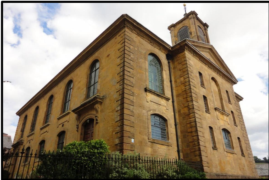
Fig. 77 The church of St George at Tiverton by the London Architect John James (1714-33, showing the new classical form of church with a two-storey exterior reflecting internal galleries (RWP Tiverton: St George DSC03267).
