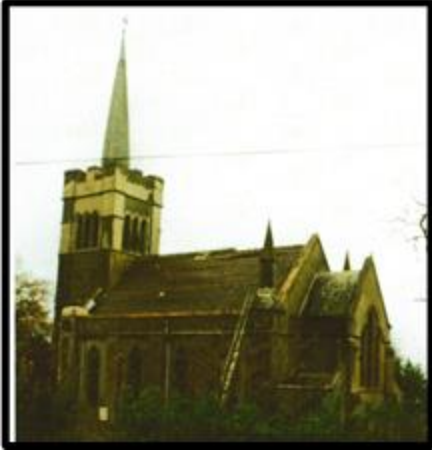
Fig. 179 All Saints Blackborough (1837-8), by John Hayward photographed by P. Lee before demolition in 1994.
