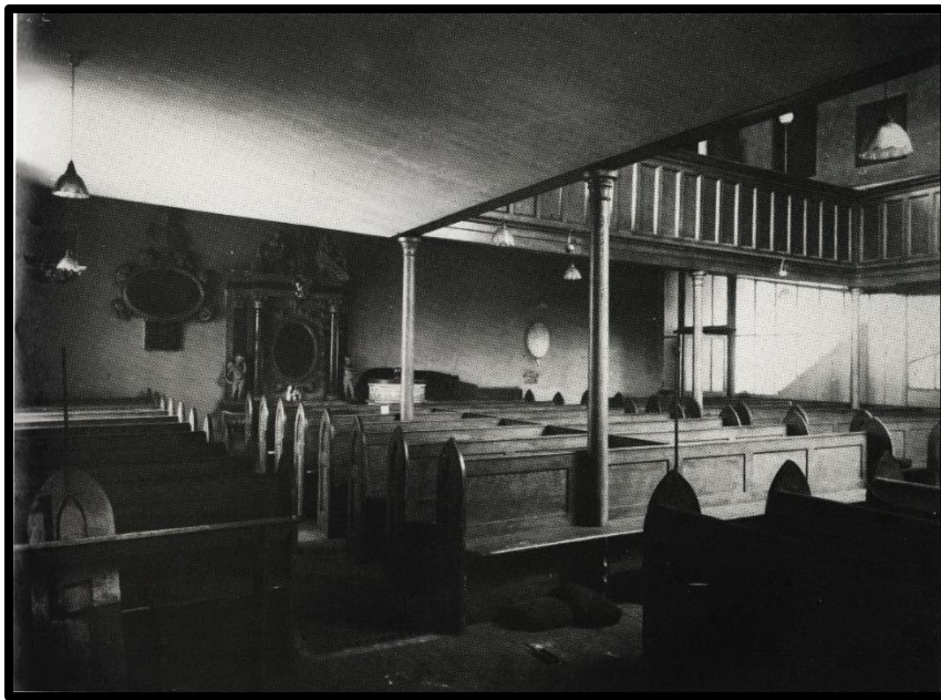
Fig. 189 The interior of St John's on Fore Street Hill, Exeter, re-ordered in 1843 to accommodate the congregation of St George the Martyr (demolished for road widening). St John's had two storeys of galleries and seems almost a deliberate rejection of ecclesiastical principles (EA Topographical Print Files, Fore Street, St John).
