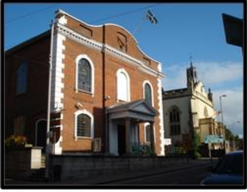
Fig 7 George's Meeting, Exeter (1760) built for a Presbyterian congregation. The rectangular form was characteristic of buildings of all denominations (RWP Exeter, George's Meeting DSC03304).
