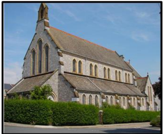
Fig. 204 St Barnabas, Stoke (1885) by J. P. St Aubyn. Demolished 2002 for a housing development (David King).
