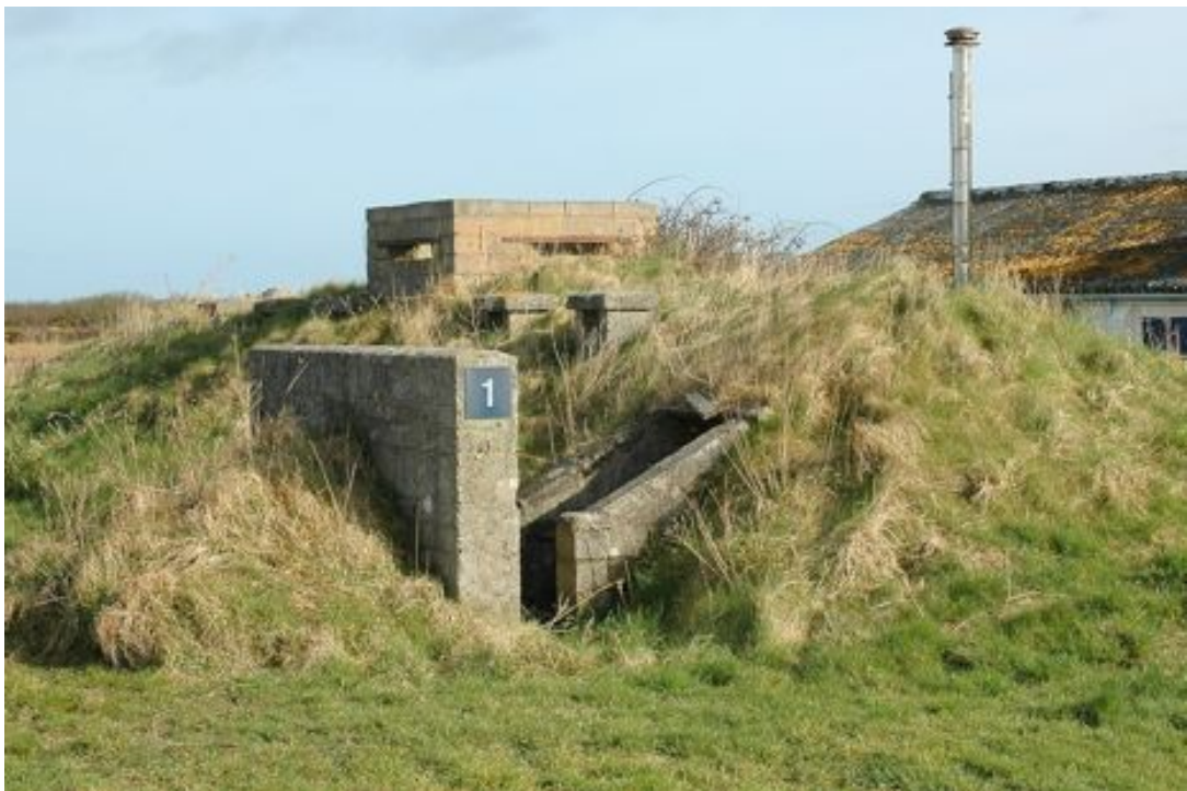
Figure 12: Air Raid Shelter at RAF Portreath - note the intact brick escape tower at the far end (Photo: Richard E Flagg)
