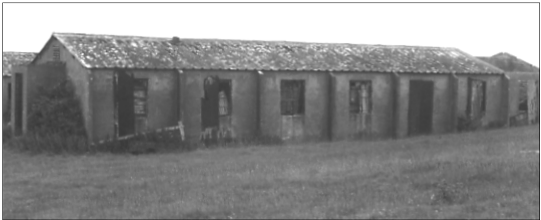
Figure 10: Extant RAF Regiment Barrack Building- RAF Scarlett (Photo: Manx Heritage Foundation)
