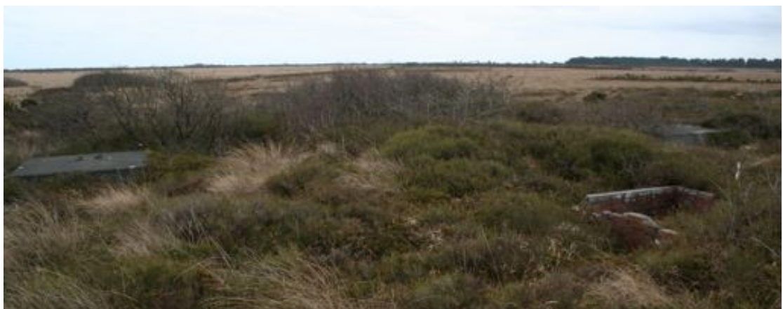
Figure 27: Receiver Aerial Bases seen at ground level. Brick structure is the cable guide. (Photo: Benjamin Oldcorn)
