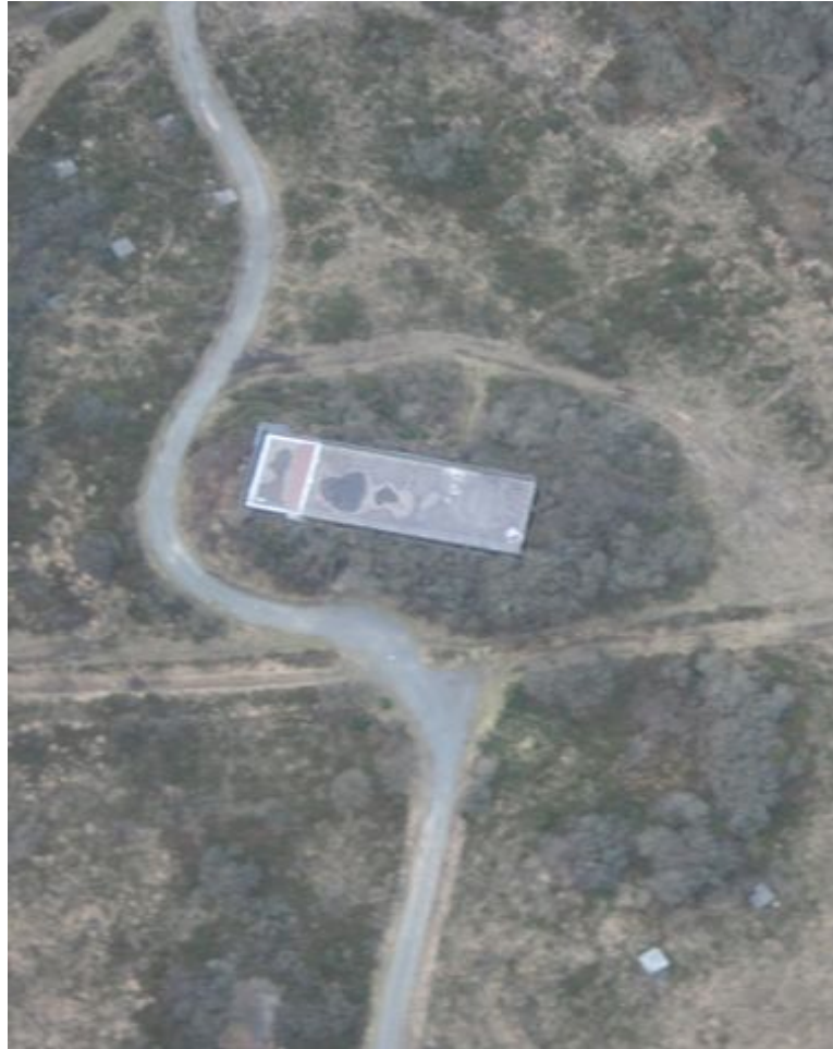
Figure 26: Receiver Aerial Bases visible adjacent to the Receiver Block (Photo: Benjamin Oldcorn)
