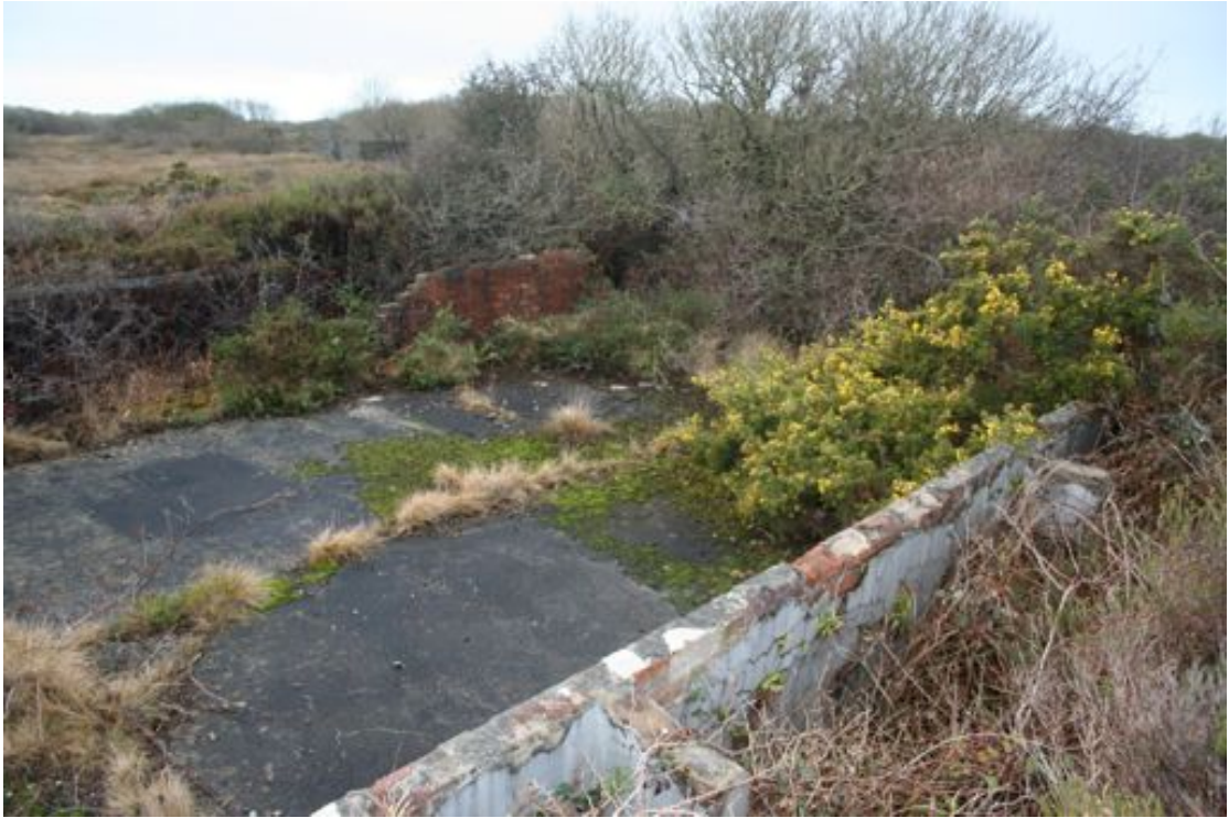
Figure 9: Overgrown portion of the Barrack Hut (Photo: Benjamin Oldcorn)
