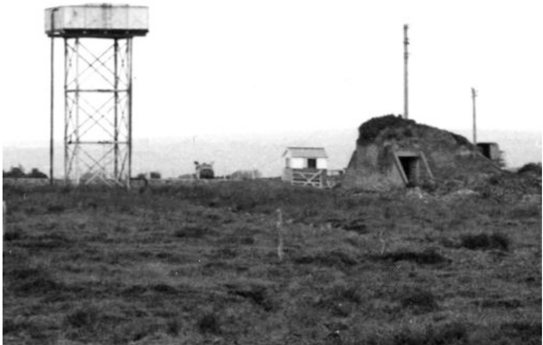
Figure 22: Water Tower (left) and CH Sub Station (right) (Photo: BT Archive)
