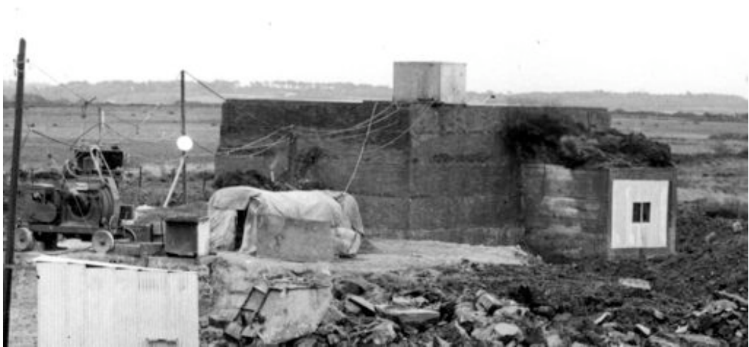
Figure 21: Standby Set House at Dry Tree (Photo: BT Archive)
