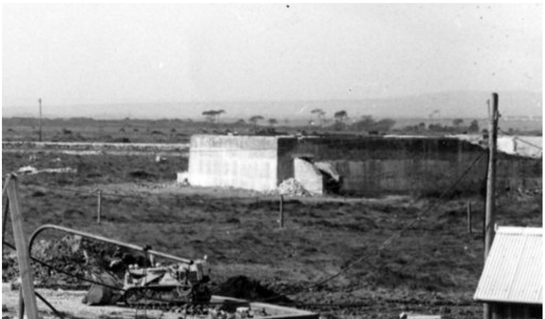
Figure 20: Intact Type B Transmitter at Dry Tree (Photo: BT Archive)
