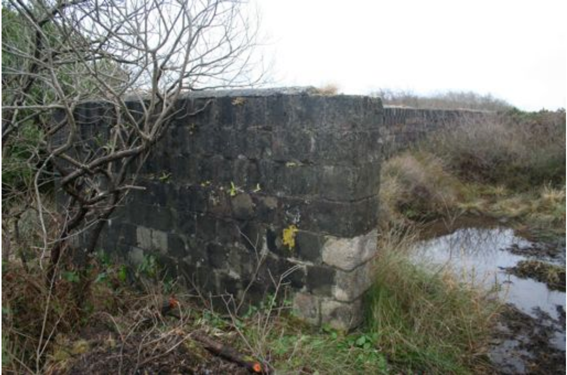
Figure 15: ICH Building at Dry Tree, Flooded. (Photo: Benjamin Oldcorn)
