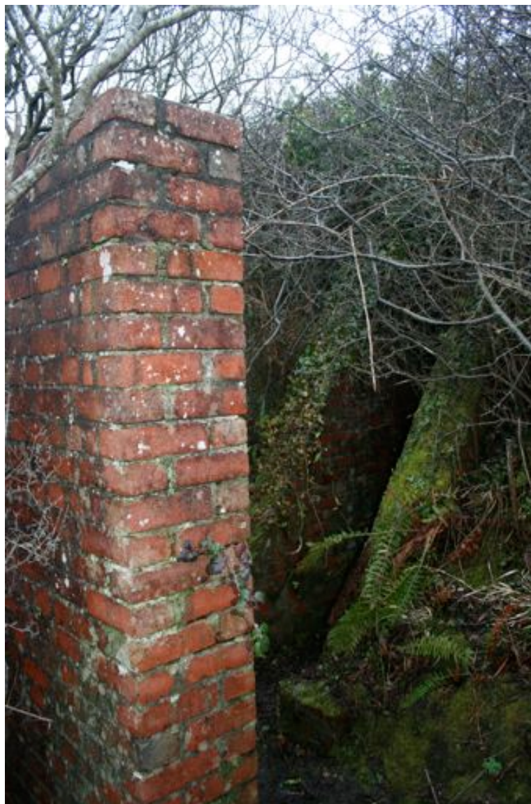
Figure 18: Second 'L' Shaped Building on Site (Photo: Benjamin Oldcorn)
