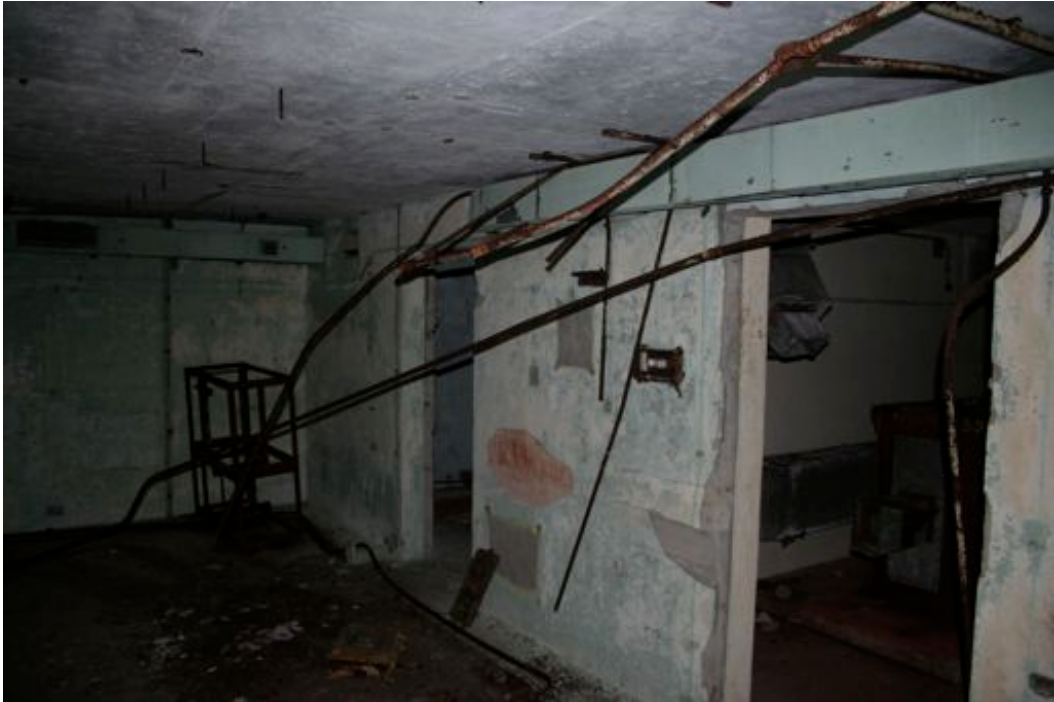
Figure 6: The Receiver Room of the Type C Building: air conditioning plant can be found intact through the doorway (Photo: Author)
