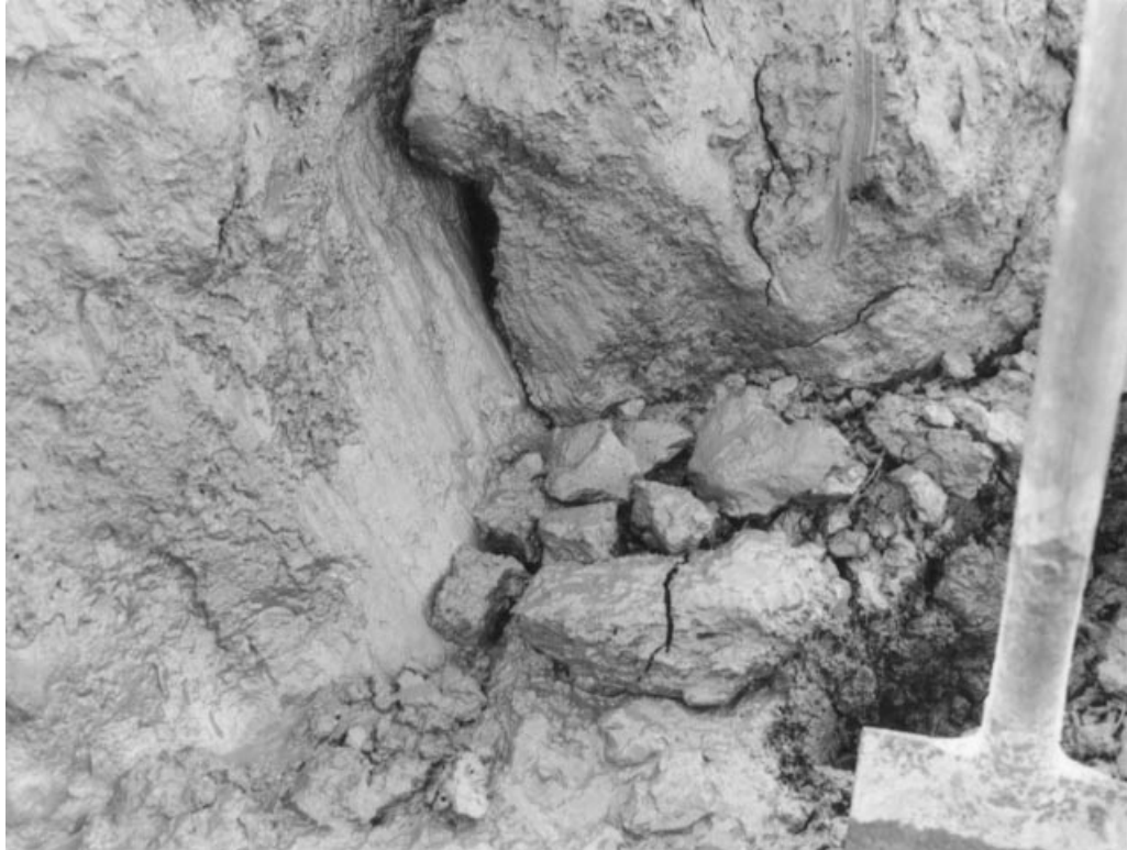
Fig. 10. Vertical striae (slickensides) on fault surfaces associated with rotational slips, Berkeley Pill, Berkeley, Gloucestershire. Spade blade 0.14m across for scale
