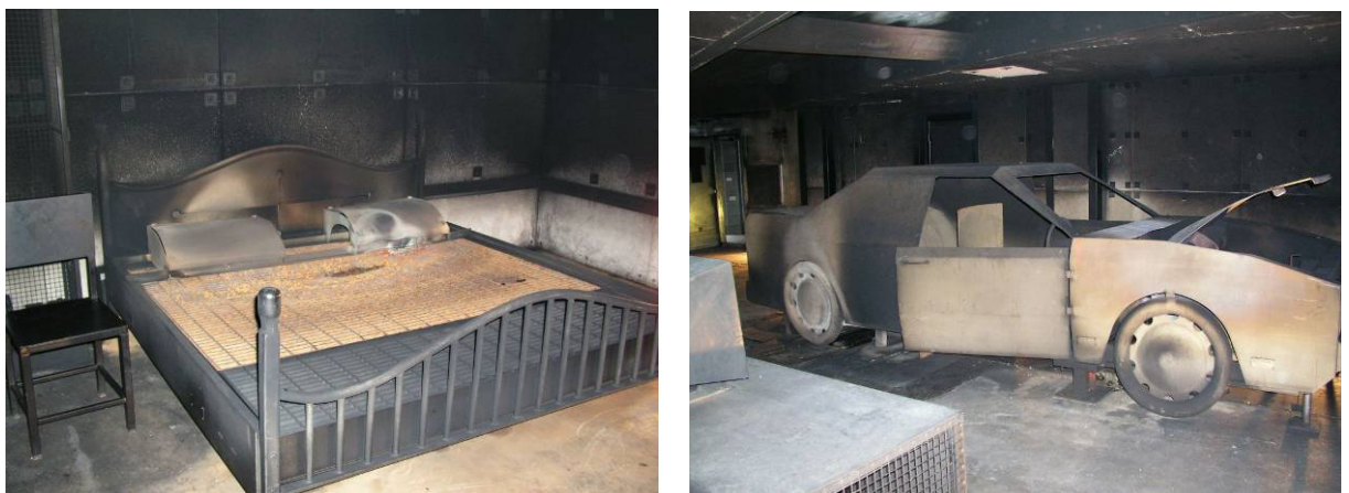
Figure 5.4: (a) 2 nd Floor ‘Bedroom’ (b) 1 st Floor ‘Garage’
