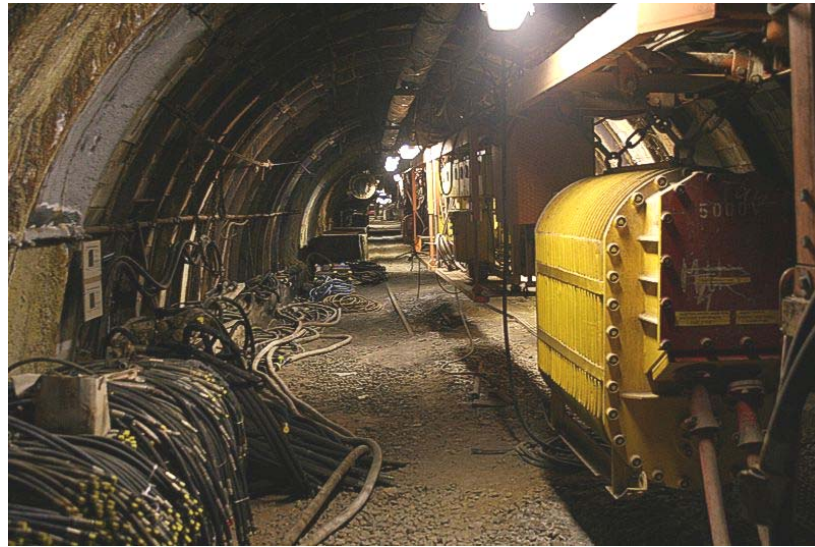
Figure 3.53: MÜZ ‘Main Tunnel’ – View from RX Equipment
