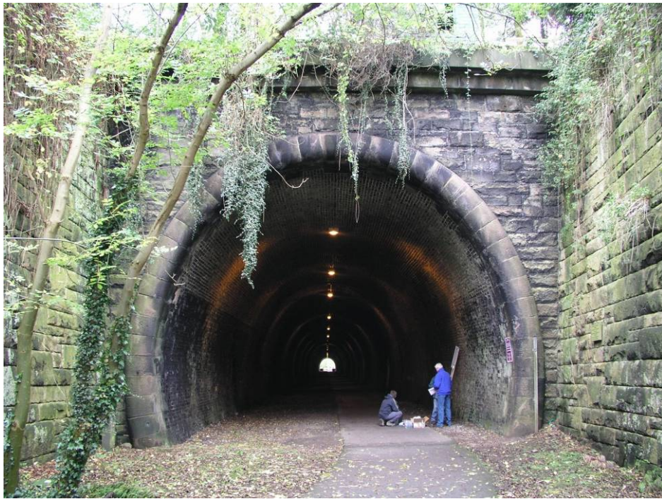
Figure 3.17: Ashbourne Railway Tunnel
