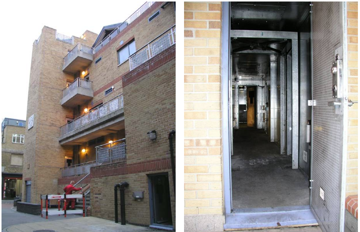
Figure 5.3: (a) LFB Southwark Training Centre (b) Main door
