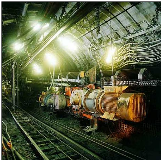
Figure 4.26: Typical Belt Conveyor Drive
