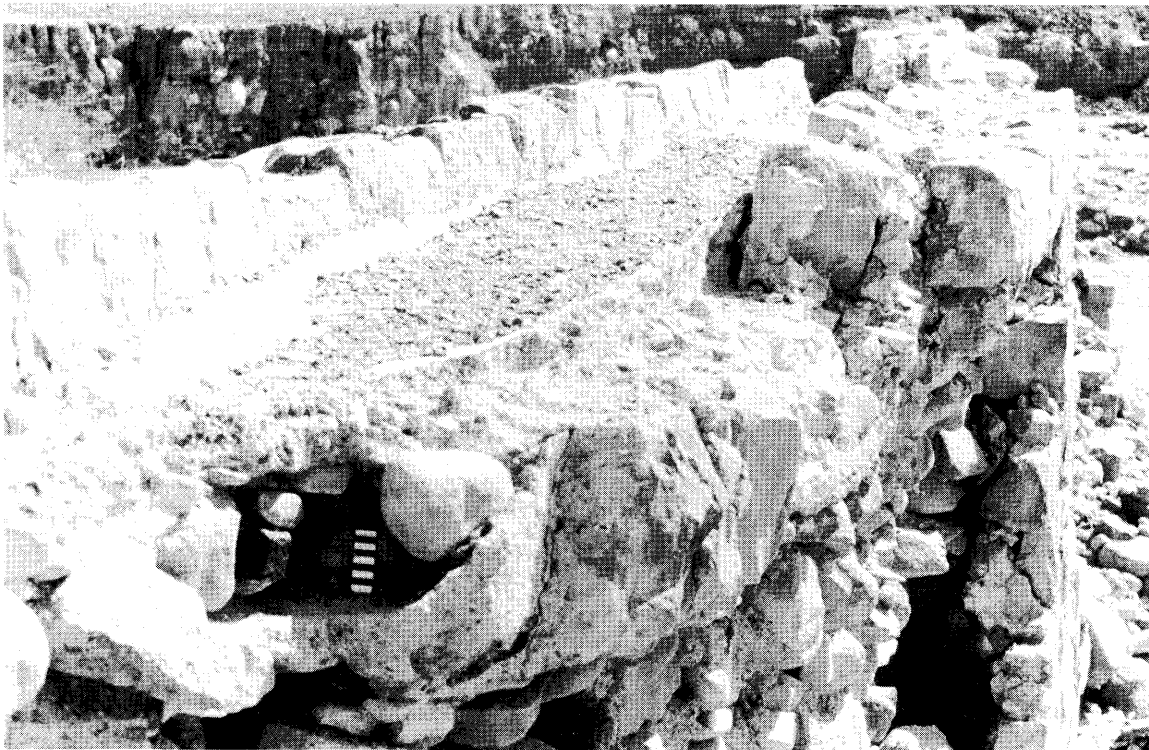
Figure 26. The aqueduct channel, showing clearly the two phases of construction, with the 10 cm. scale on the lower channel. (Photograph: D. Crook).
