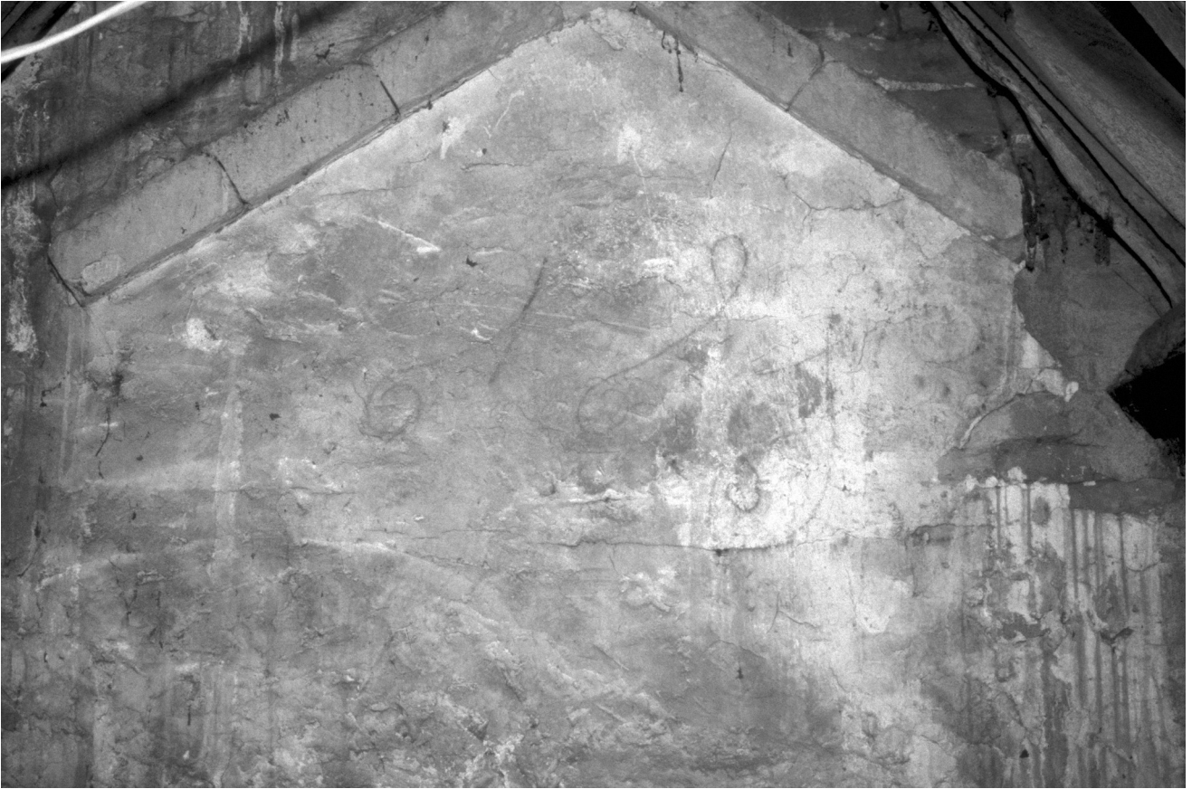
8.9 Early roof line and graffiti on the eastern side of the church tower, now covered by a steeper pitched roof (photo by Richard Parker)
