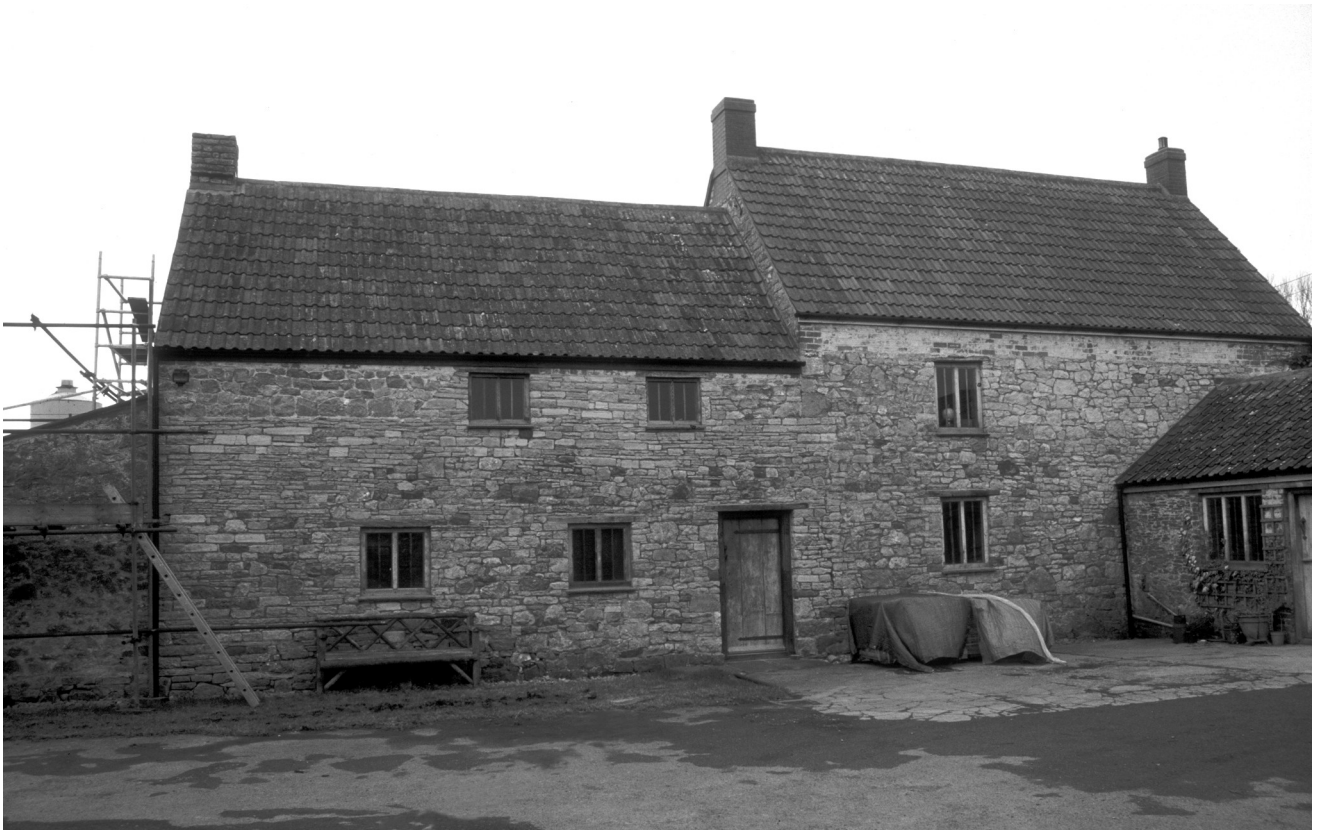
8.4 Hodders Farm: this house is unusual in having had its grey external render removed, revealing a complex structural history starting with a single celled house (centre left), whose walls were raised to accommodate a first floor, and then extended to create a three-roomed cross passage house.
