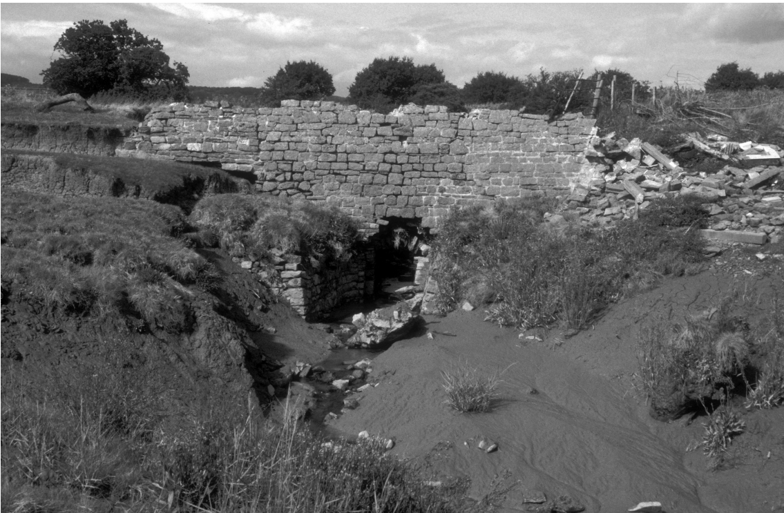
Figure 5.5 The bridge over Grange Pill in the high saltmarshes of Woolaston, Gloucestershire, that may have had its origins as a dam and sluice analogous to those used in the Roman period on reclaimed marshlands such as the North Somerset Levels.
