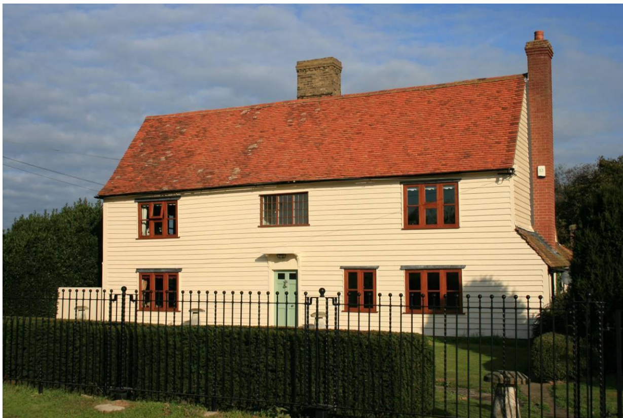
Figure 15: the 16 th or 17 th century Bolts Farm in Barling: an example of a traditional weather-boarded timber framed house.
