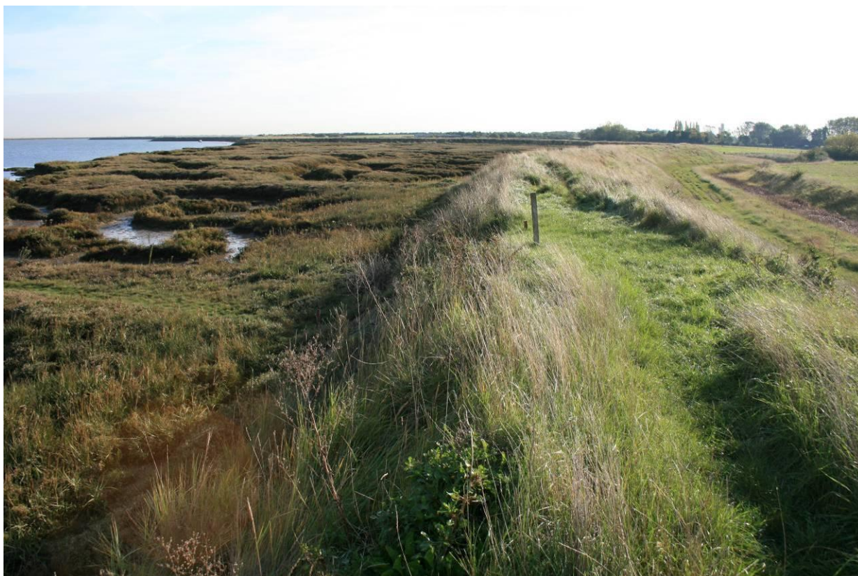
Figure 16: the sea wall north of Bolts Farm in Barling
