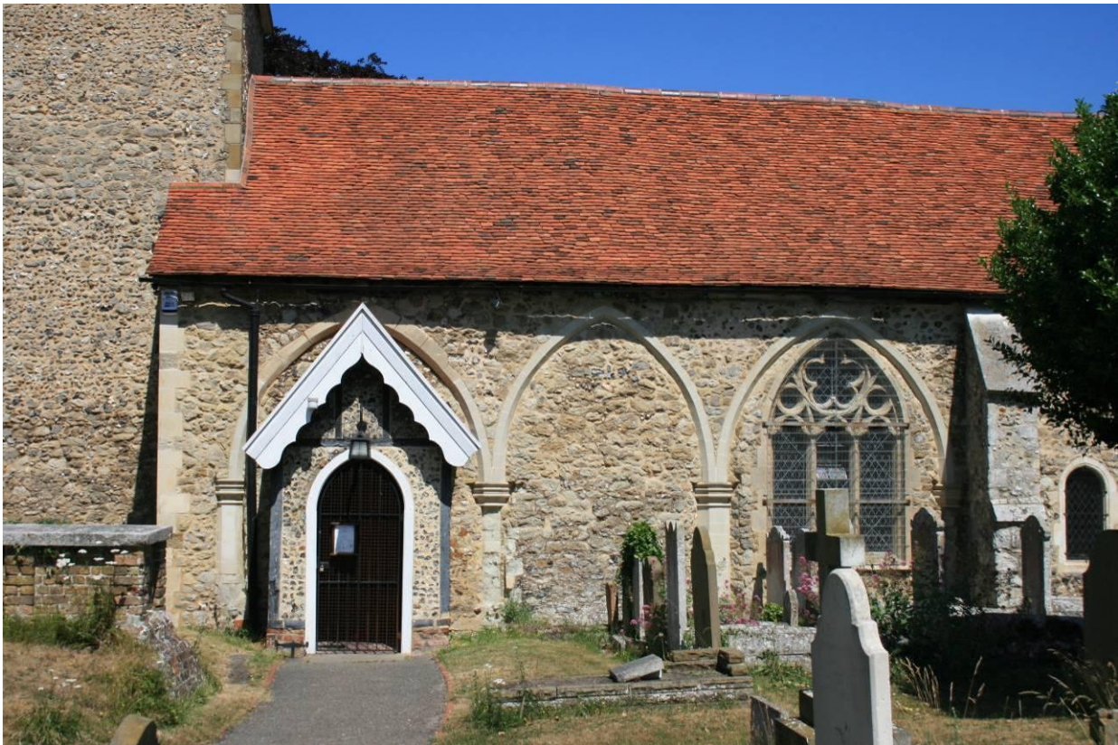
Figure 14: the south side of North Shoebury church. The former 13 th century south aisle was demolished (probably in the 15 th century) and the new south wall of the nave was built by blocking the former arches of the arcade.
