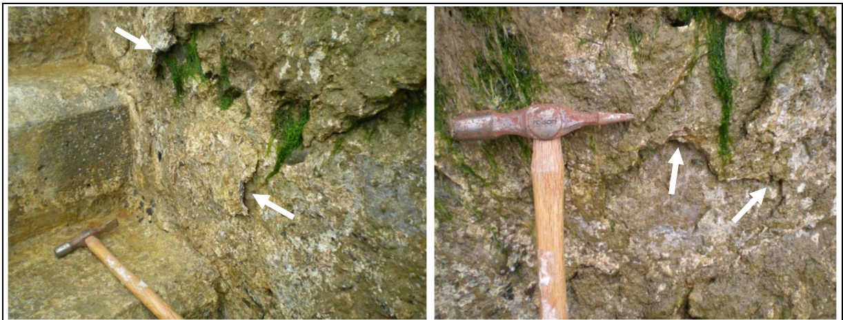
Figure A3 - 7 Surface scaling of concrete (indicated) from vertical walls at Newlyn Harbour, Cornwall (hammer handle width = 2.5 cm for scale).
