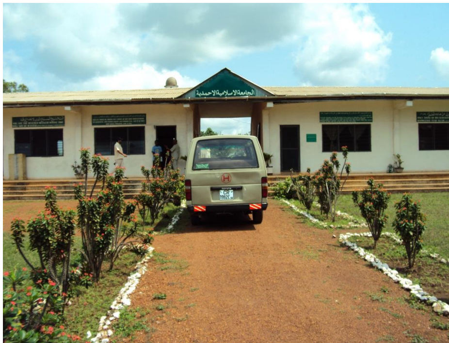
Fig. 4.4.5. The front view of the Administration block, Ahmadiyya Missionary training college at Ekrawfo
