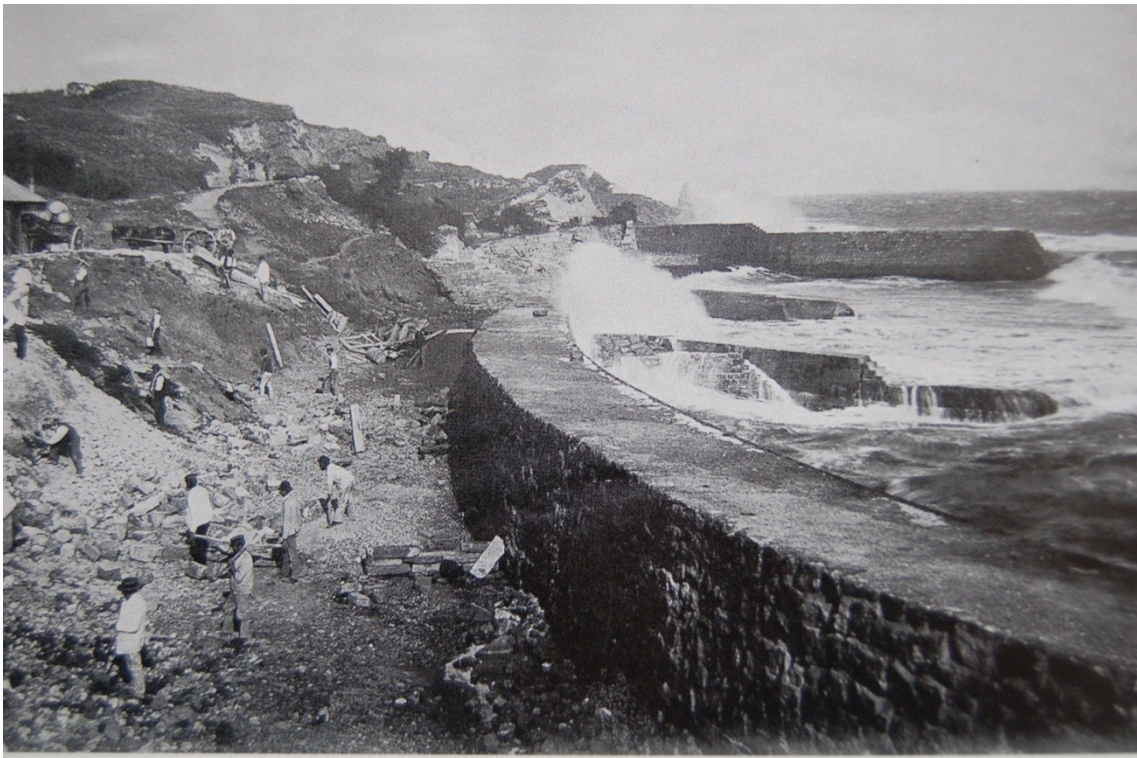
Figure 6.19 The construction of 'Spindler's Harbour' at Binnel Bay (from McInnes 2006)
