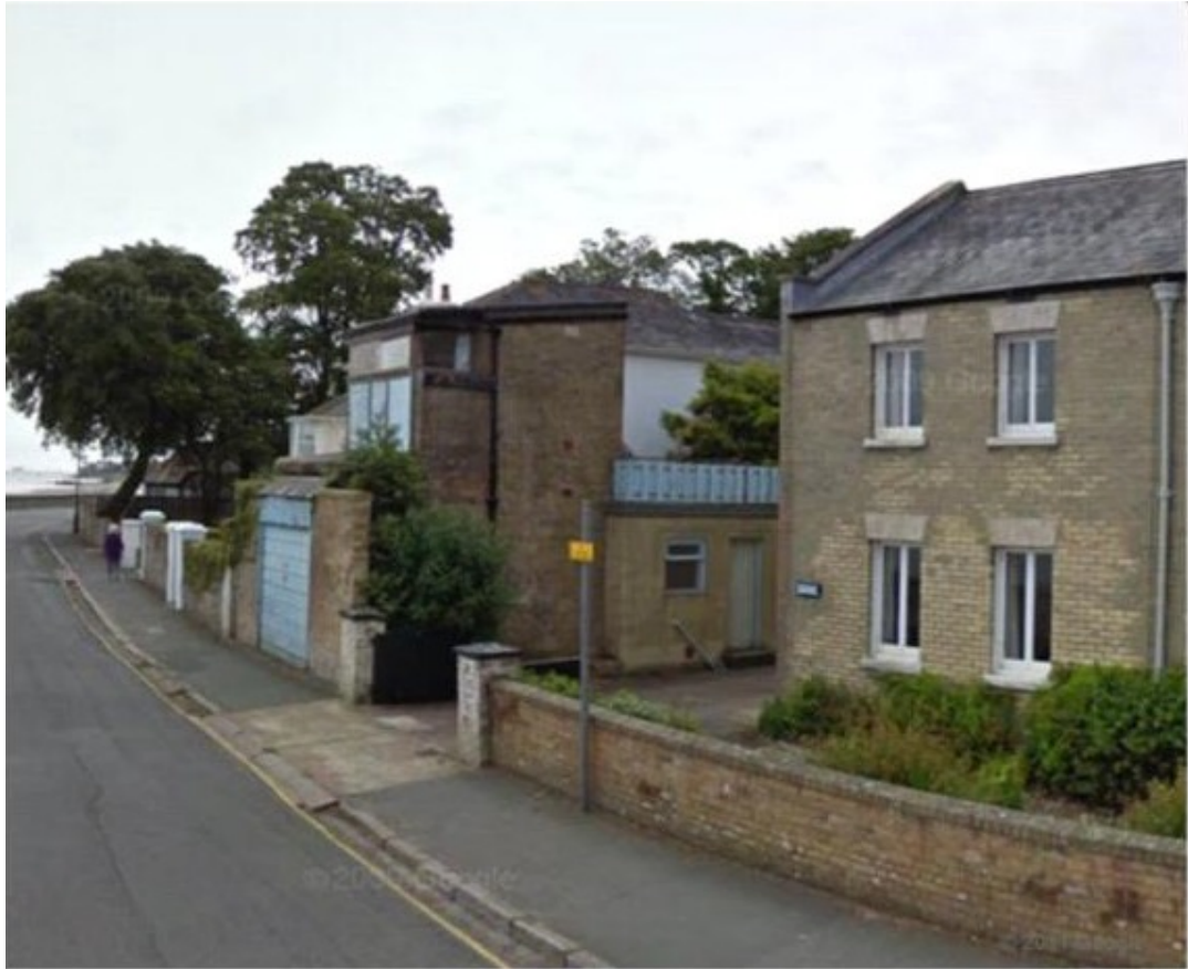
Figure 9.7 Google maps image of the position finding cell adjacent to the Coastguard Cottages at Springvale. The structure has now been demolished
