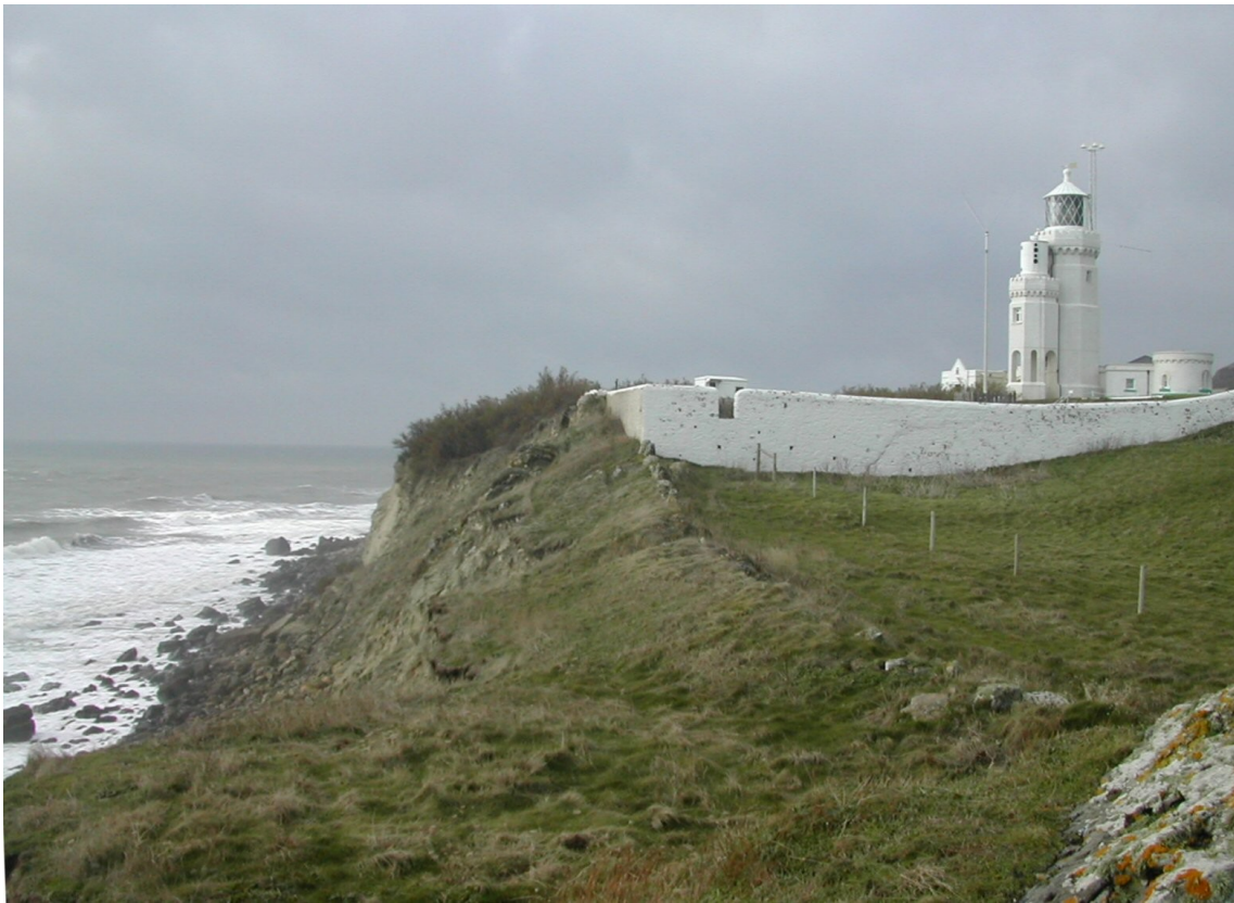
Figure 6.17 The eroding cliff adjacent to St. Catherine's Lighthouse
