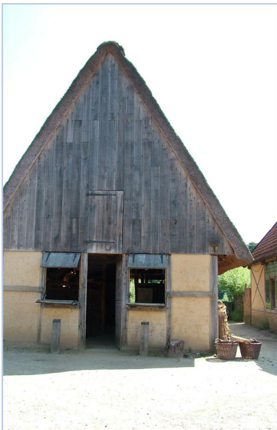
Figure 5.16: Exterior of the Craftsmen house at HOME.
