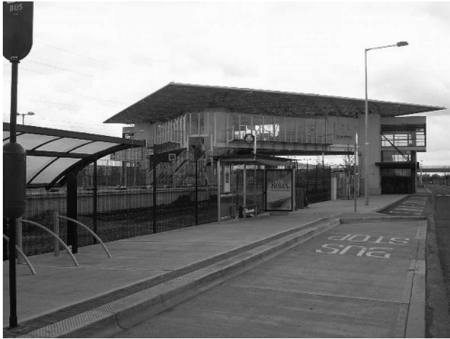
Figure 5. Adamstown central rail station (A in Figure 4)
