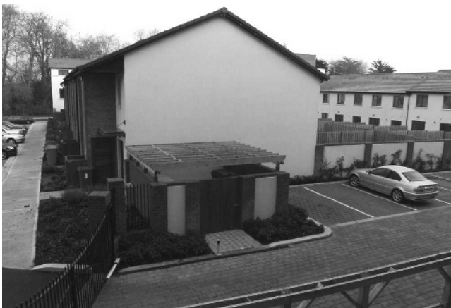
Figure 8. Waste collection points and gated private parking spaces for apartments (front) with adjoining low density housing (rear) within Adamstown Castle (C in Figure 4)
