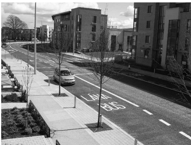
Figure 6. Quality bus corridor (QBC) in Adamstown Castle (B in Figure 4)
