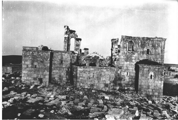
El-Adra, general view of exterior from E (Bell, S_178)
