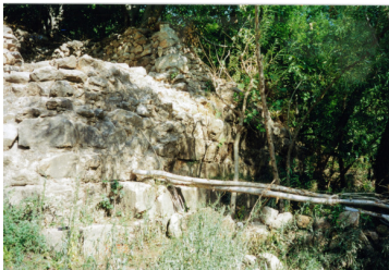
Piers of Roman bridge
