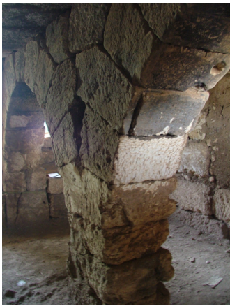
Interior of tower at Yoğunburç
