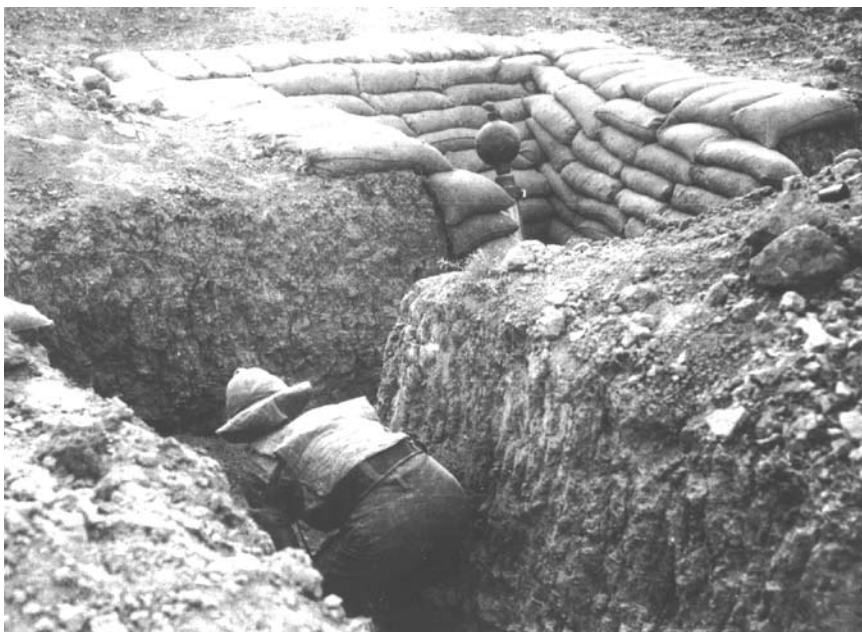
Fig. 68 (left) A 2-inch mortar emplacement in the Middle East. See Fig. 69. Note the shape and the sandbags. The No. 1 is about to pull a lanyard to fire the mortar. He is wearing body armour (IWM)
