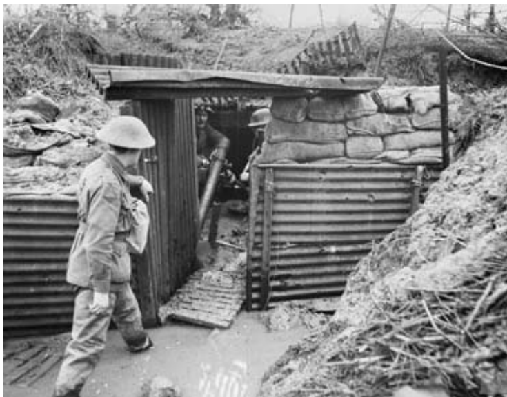
Fig. 71 Stokes mortar emplacement, June 1918. There are three men in the picture, two with the mortar. Note the sandbags and corrugated iron and the wet conditions (Australian War Memorial)
