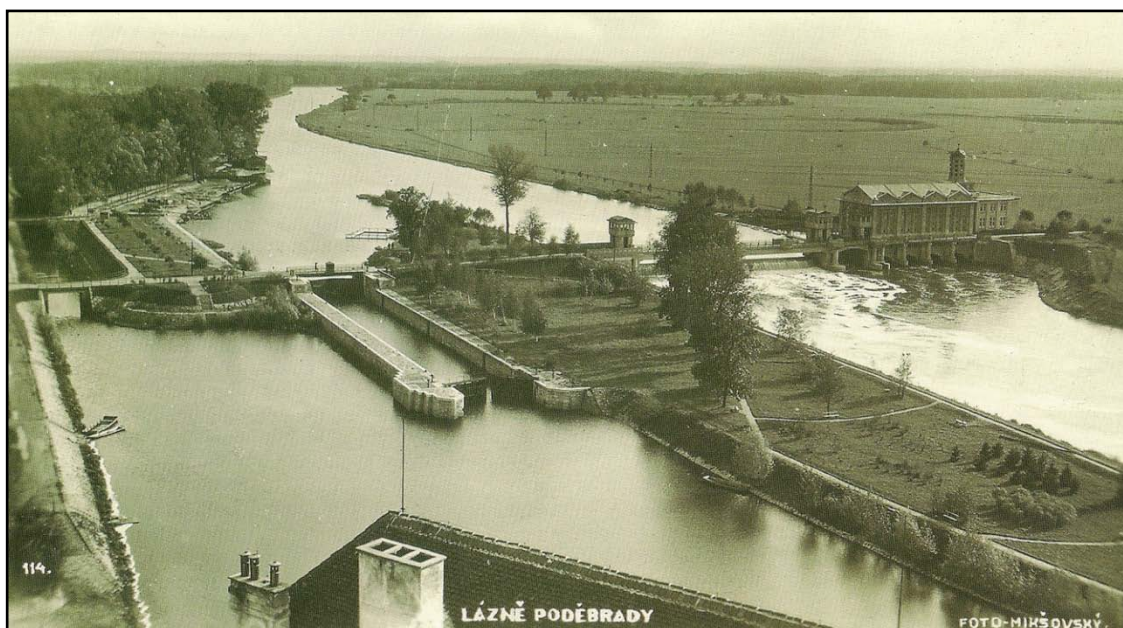
Figure 4.29 The Poděbrady 3 logboat was found during construction work at the town's hydroelectric station in 1964 (far right). The dam, power station sluiceway and locks for boat traffic were originally built from 1913 – 1918 (photograph from the 1930s, published in Vácha and Stegbauer 2006:130).
