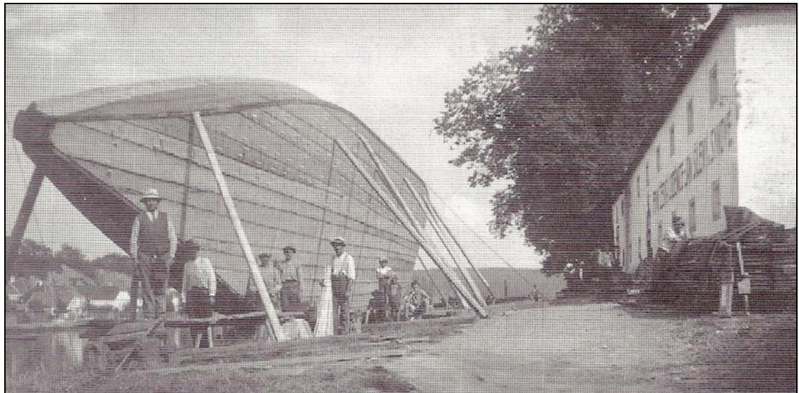
Figure 3.16 Boat construction in front of the salt house at Týn nad Vltavou, late 19 th century (photograph from Hubert 2008:85). In contrast to the vessel in the previous figure, this boat has a pointed bow. Both vessel types would be towed by horse from the riverbank.
