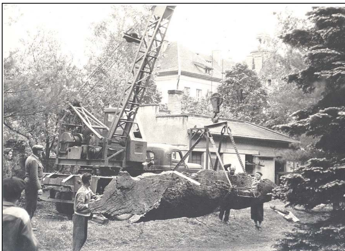
Figure 4.33 Unloading the Přerov vessel at the museum yard in Český Brod (photograph courtesy of the Kolín Regional Museum).
