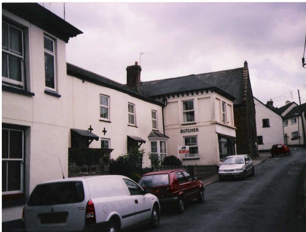
Figure 4.18 4 Conduit Street, still a Butcher's Premises in 2009
