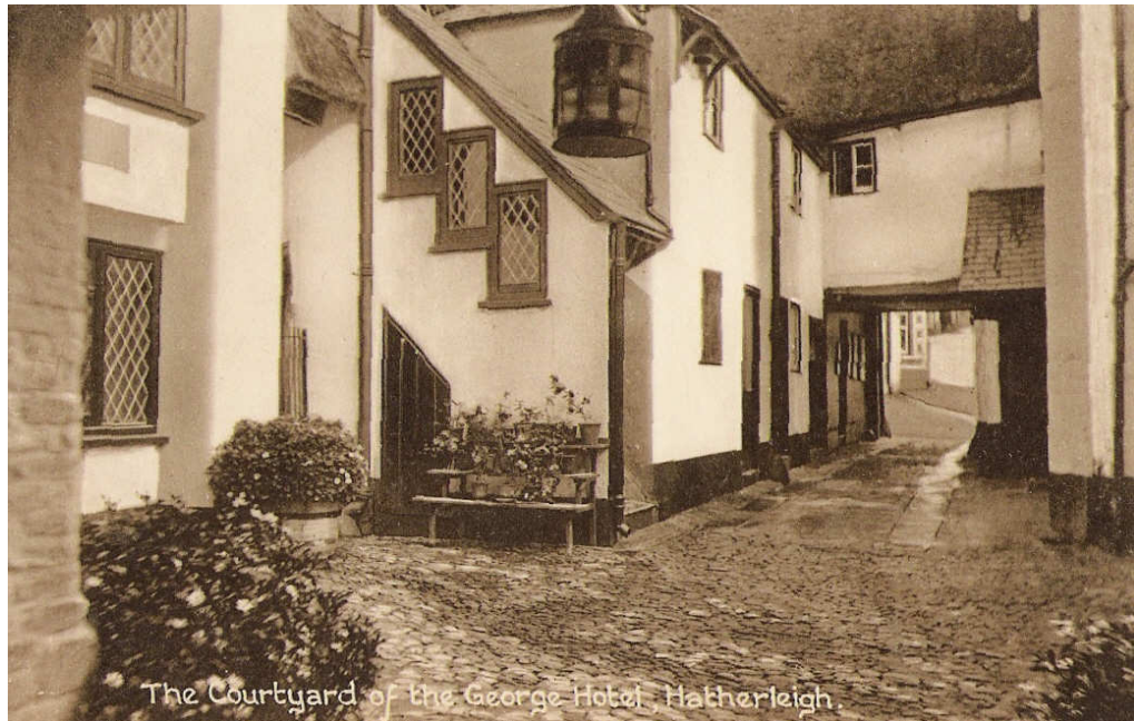
Figure 2.12 The Courtyard of The George Hotel
