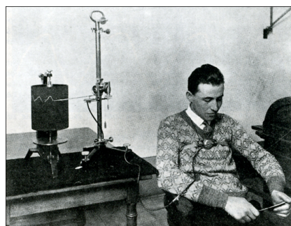
Fig. 4.7a: Mosso plethysmograph detected changes in blood pulsations attributed to an untruthful state of mind. Fig. 4.7b: Marey pneumograph used by Musatti measured the changing in breathing during an interrogation. (Musatti 1989)
