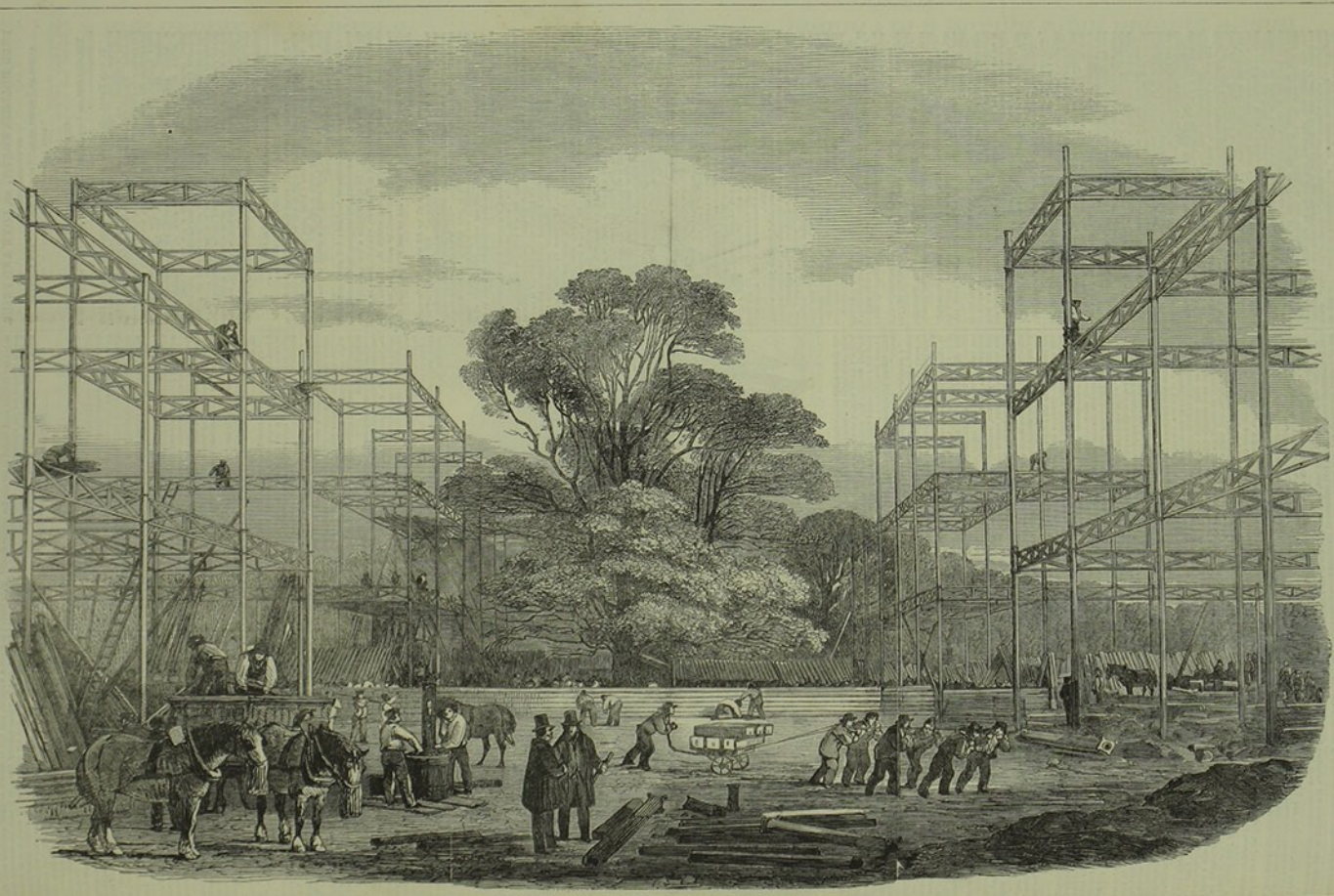
THE BUILDING IN HYDE PARK FOR THE GREAT EXHIBITION OF 1851.—THE TRANSEPT.—(COOKING WORKS)
