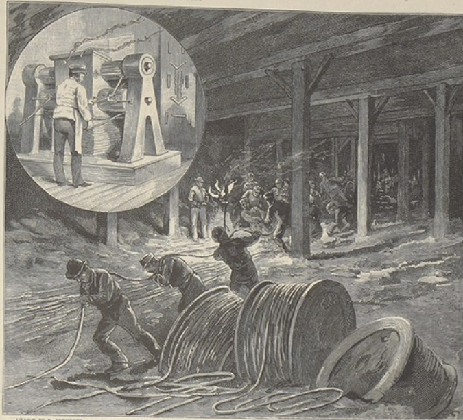
DRAWN BY J. FRENCH LAYING THE WIRES UNDER THE FLOOR OF THE MAIN AISLE, CRYSTAL PALACE
