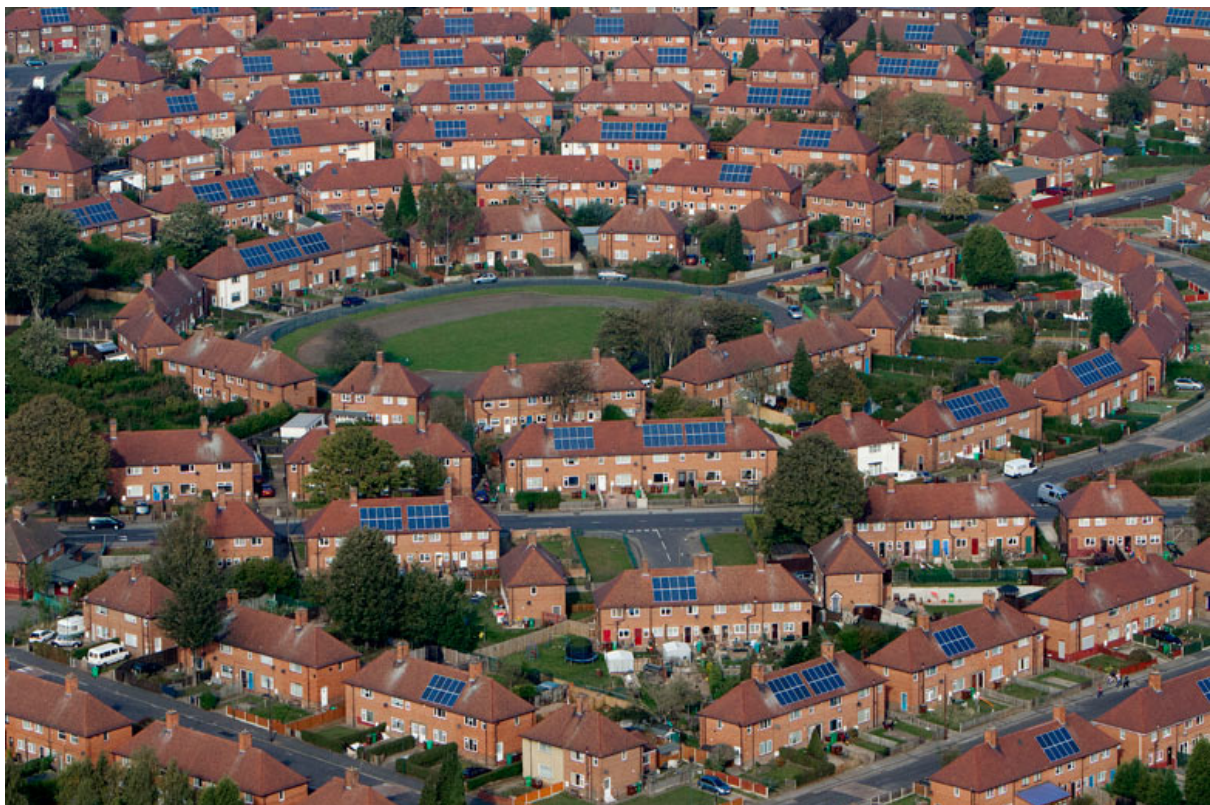
FIGURE 6.3 SOLAR PV ARRAYS ON SOCIAL HOUSING IN ASPLEY, NOTTINGHAM
