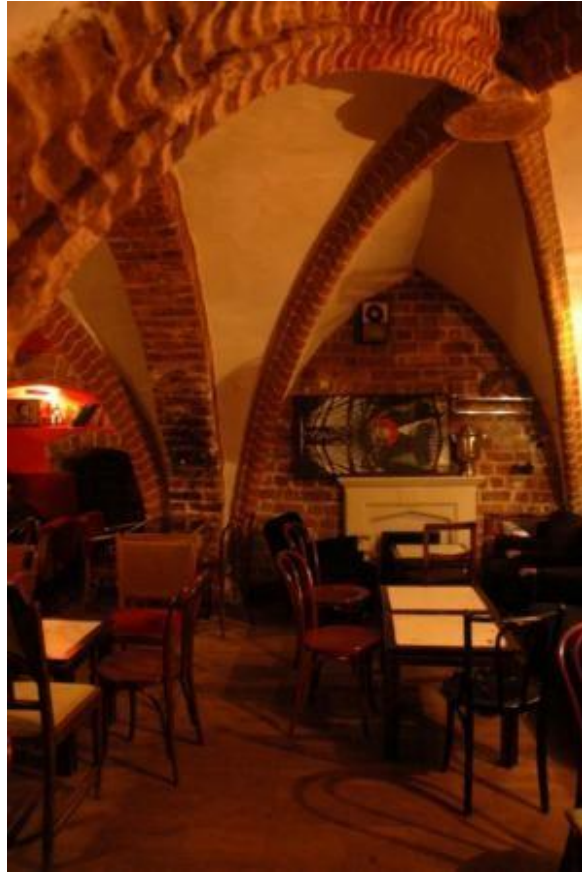
Figure 18: Więzienna Prison, Wrocław – one of the cell rooms with its original ceiling and walls.
