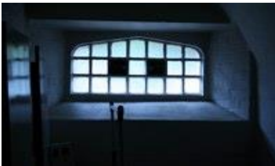
Figure 23: One of the windows in the Exeter Guildhall cell.
