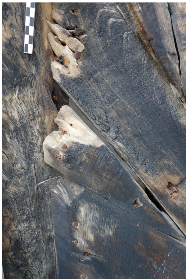
Figure 25. The nailed and screwed hood-ends above the fourth strake of kettuvallam B. (Image: Chiara Zazzaro).
