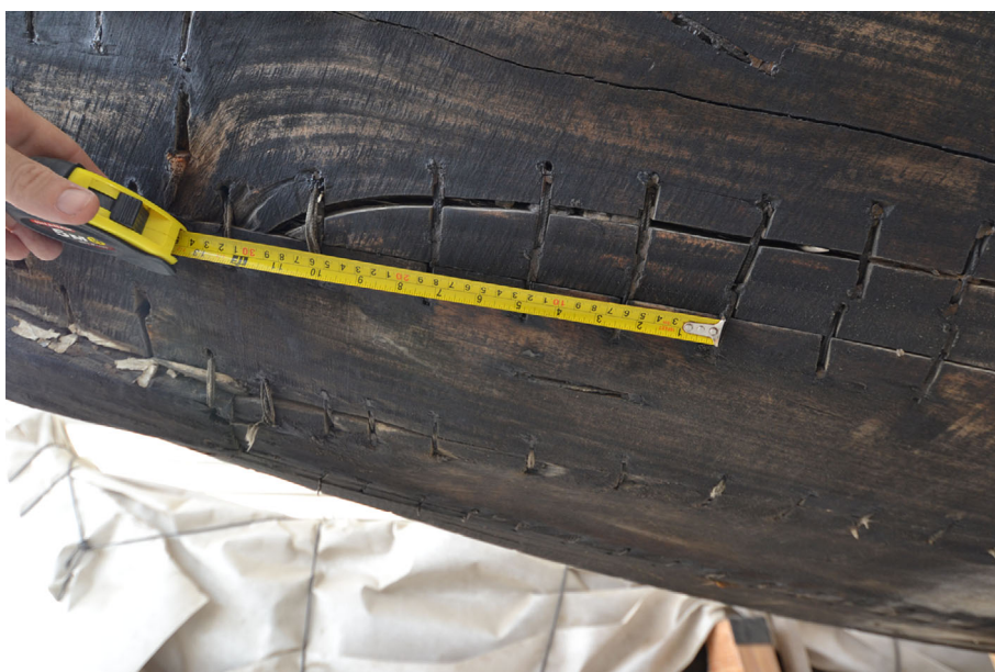
Figure 27. Stitched repair of a crack on kettuvallam B (Image: Alessandro Ghidoni).
