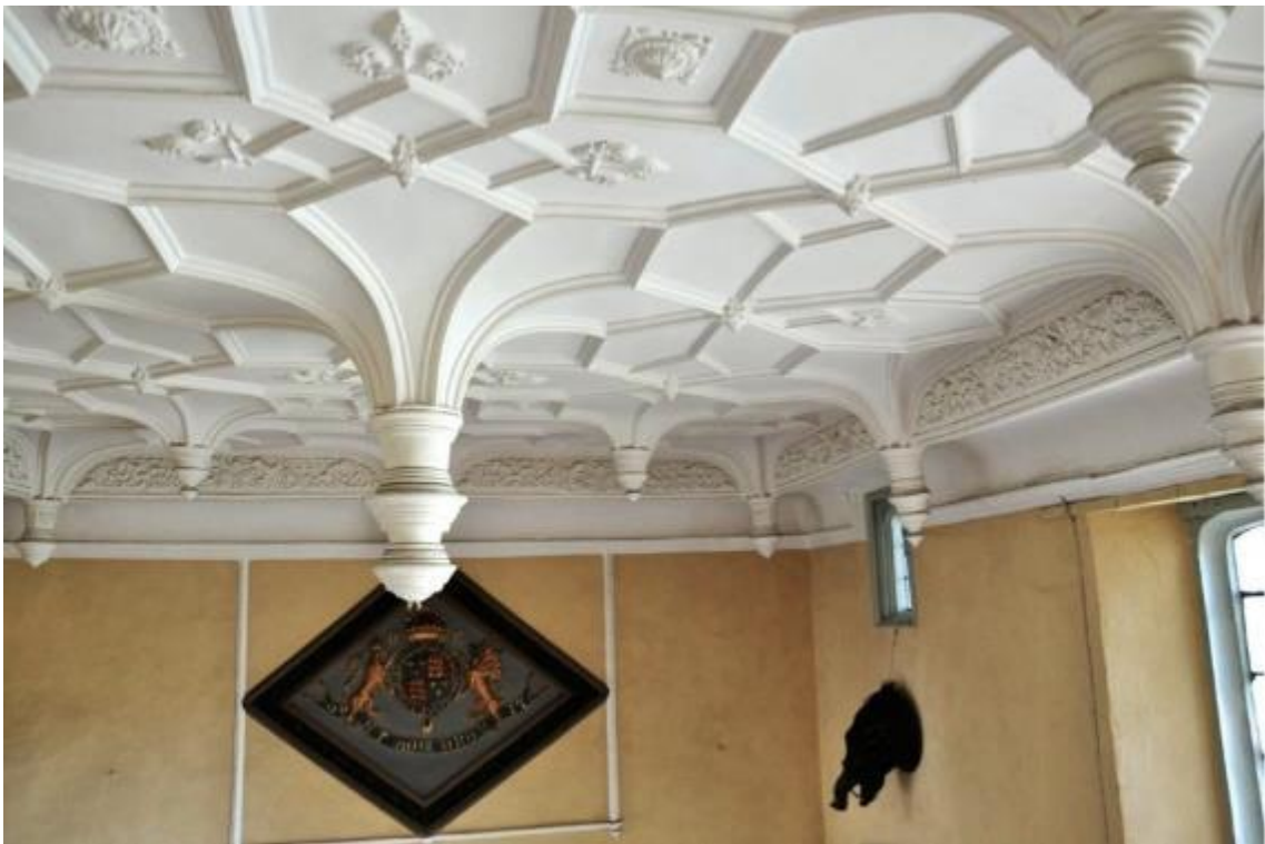
3.34 Ceiling, hall, Poundisford Park, Somerset (TA24).
