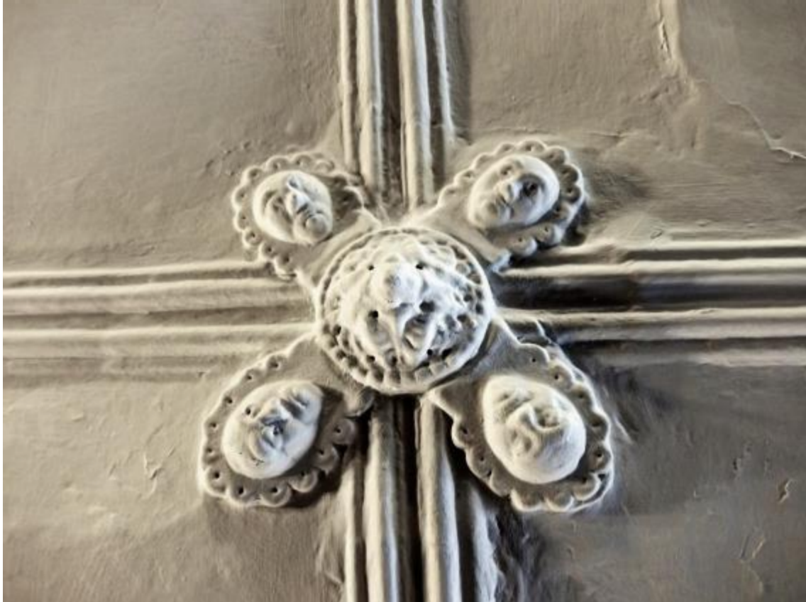
3.76 Boss, ceiling, 10 Duke Street, Dartmouth (SH8).
