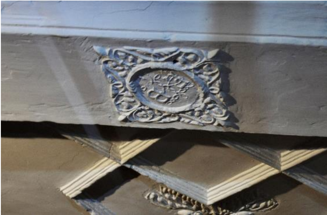
3.57 Ceiling beam, Bogan House, 43 High Street, Totnes (SH45).
