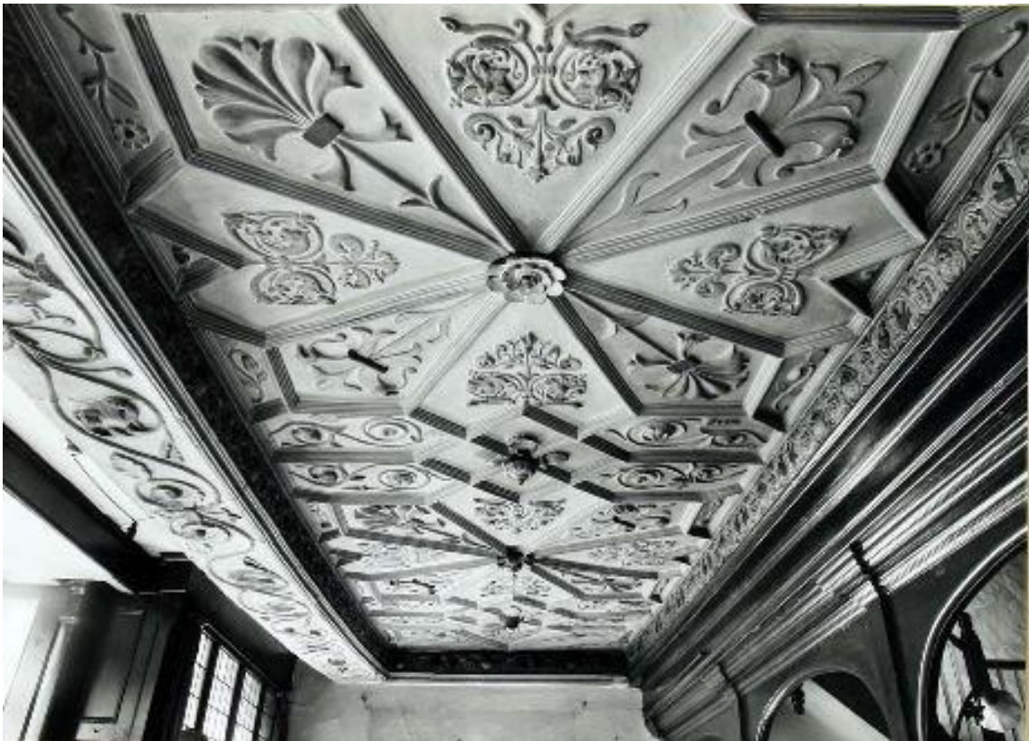
1.06 Ceiling, 38 North Street, Exeter (EX17) in 1971 [© Crown copyright. Historic England Archive, 0962_041].
