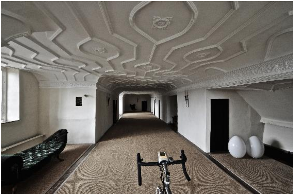
3.22 Ceiling, gallery, Holcombe Court, Devon (MD11).
