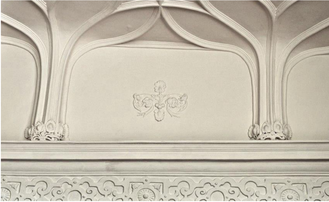
3.23 Ceiling, great chamber, Holcombe Court, Devon (MD11).
