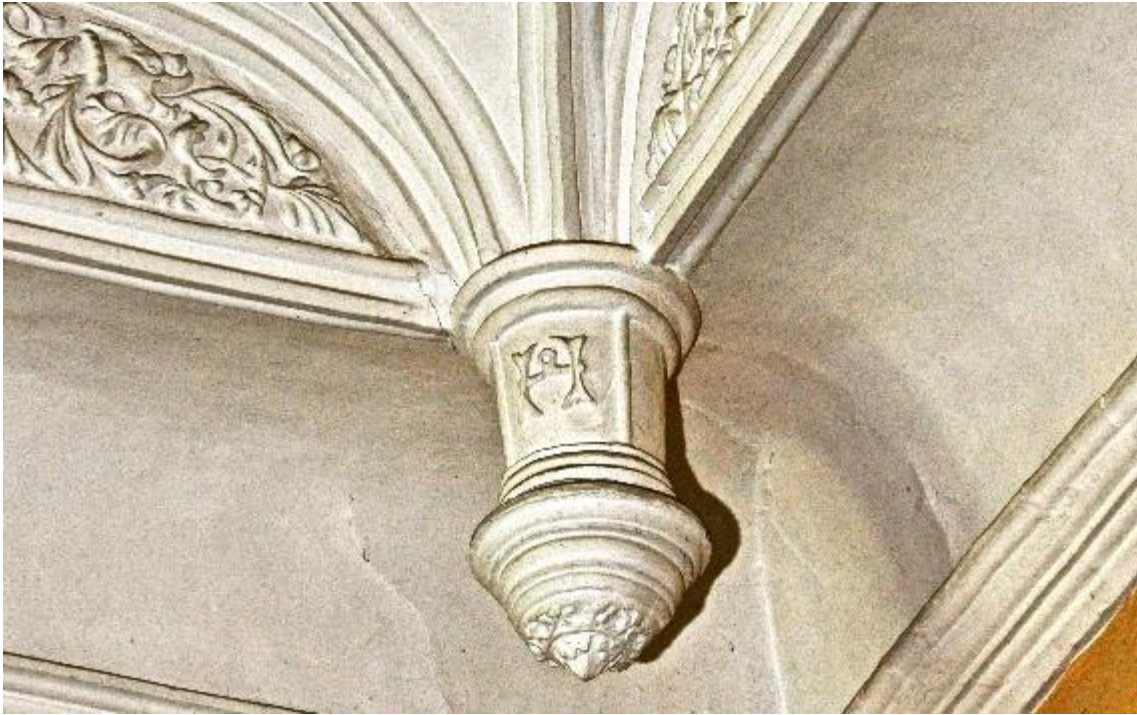
6.13 Pendant, hall, Poundisford Park, Somerset (TA24).
