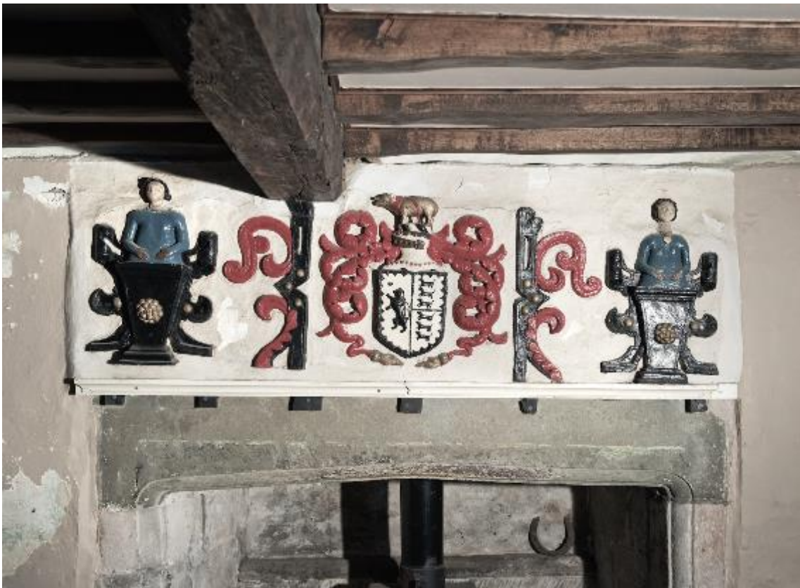
6.06 Overmantel, Beara Farm, Ilfracombe, Devon (ND40). [© Crown copyright. Historic England Archive, DP113817].
