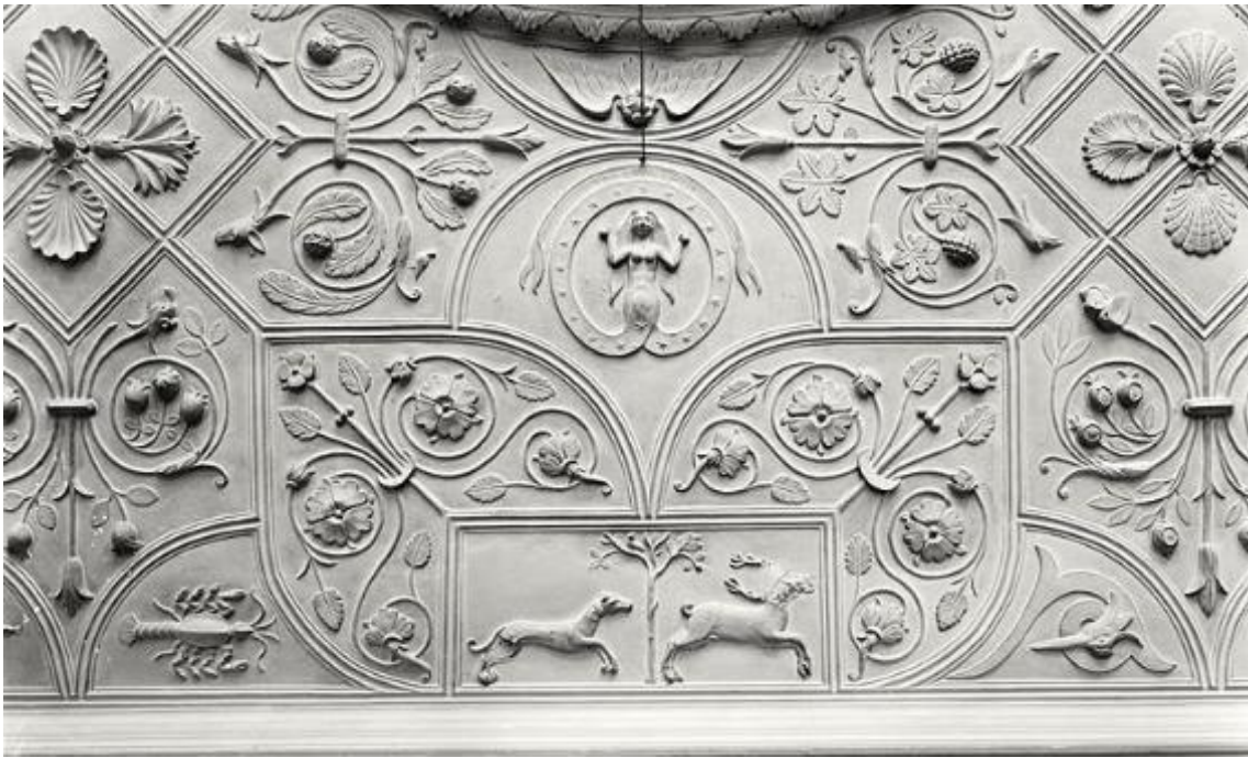
3.73 Ceiling, Hinton House, Somerset (SS10) [© Crown copyright. Historic England Archive BB68/06325. Reproduced under licence].
