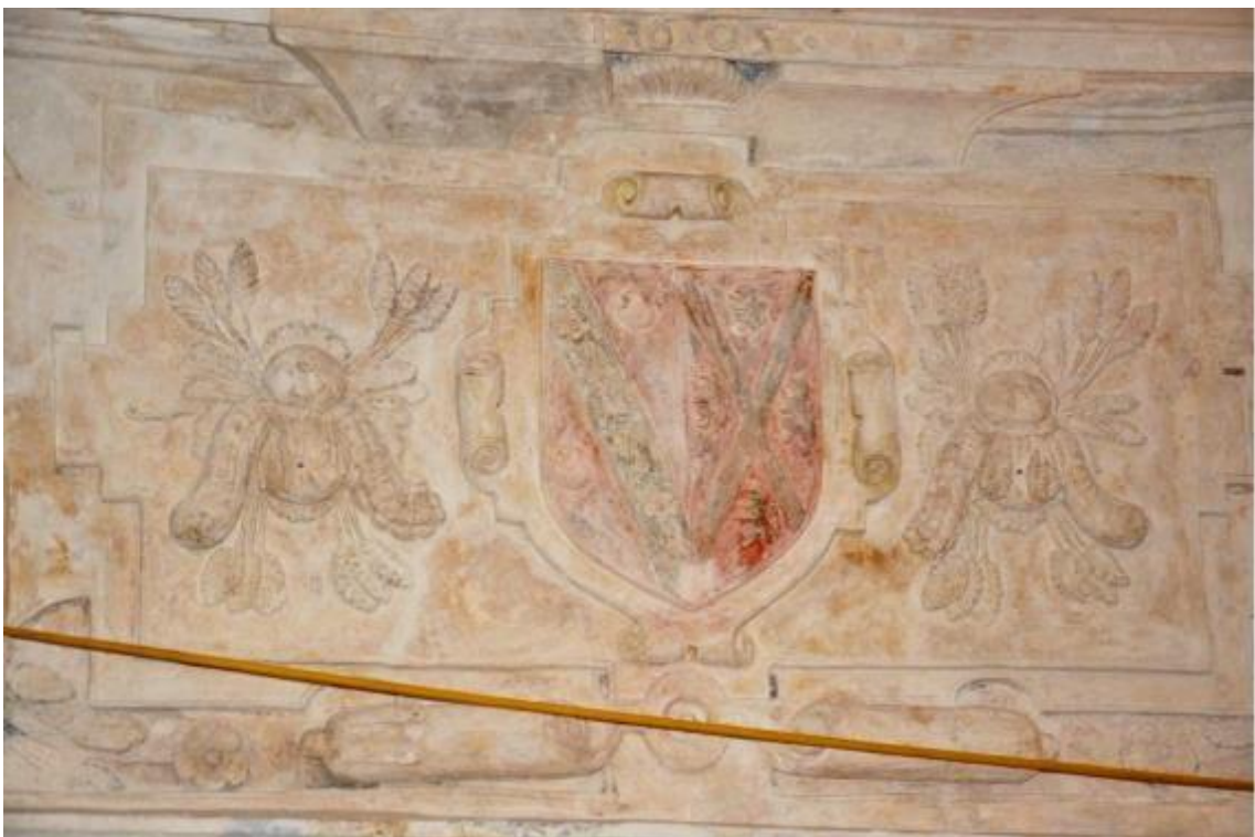
3.04 Overmantel prior to repainting (2013), hall, Walronds, Cullompton (MD6).
