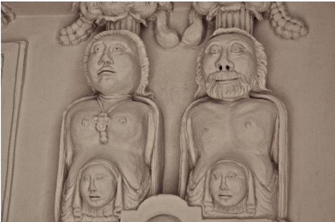
5.12 Caryatids, overmantel, Parlour Chamber, Holcombe Court, Devon (MD11).
