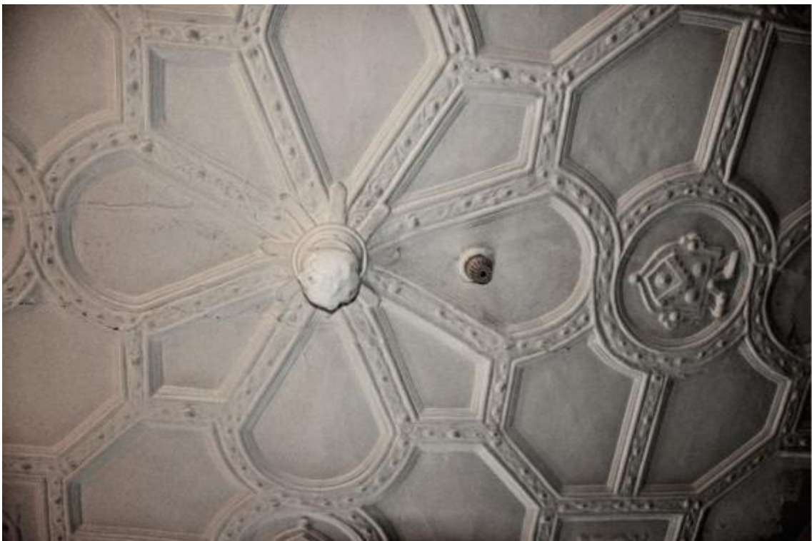
3.26 Ceiling, rear first floor chamber, 18 Fore Street, Taunton (TA33).
