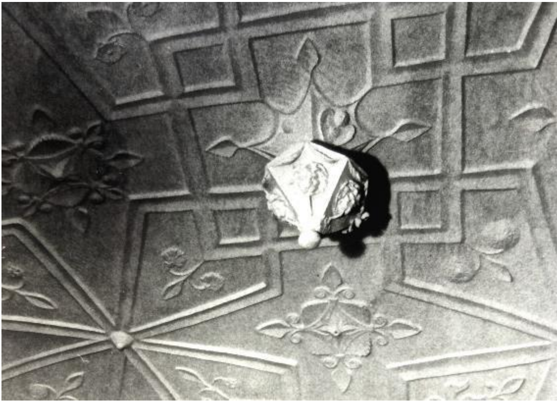
3.25 Ceiling, Court House, Chard, Somerset (SS6) [Reproduced with the kind permission of Somerset Archives and Local Studies Service, A\ECU/1].
