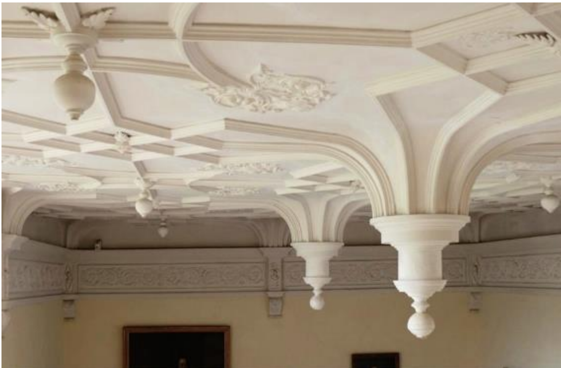
3.32 Ceiling, hall, Trecice, Cornwall (CO29).
