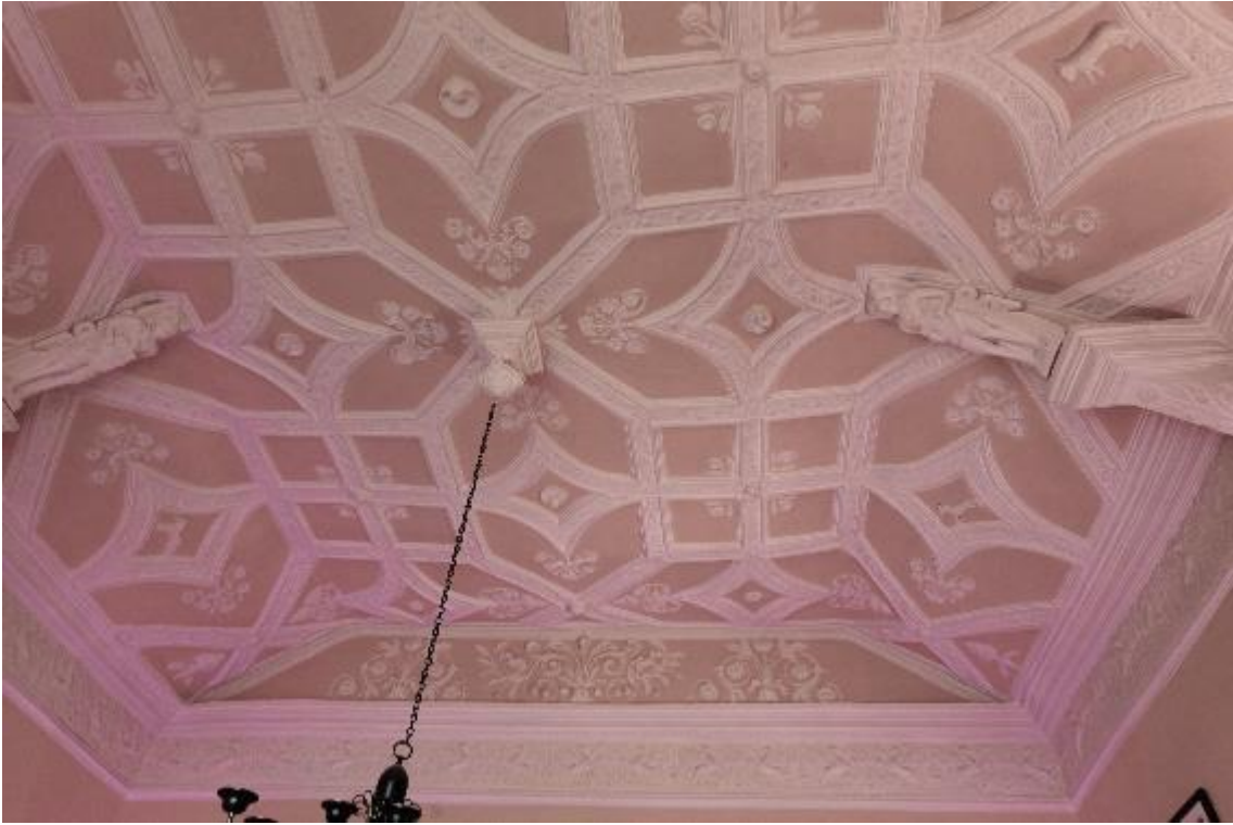
5.27 Rear ceiling, 62 Boutport Street, Barnstaple (ND3).
