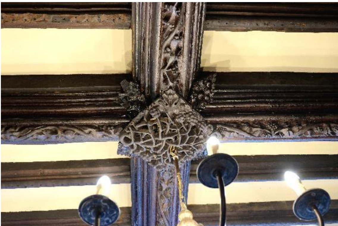
2.06 Ceiling, hall, Godolphin, Cornwall (CO4).
