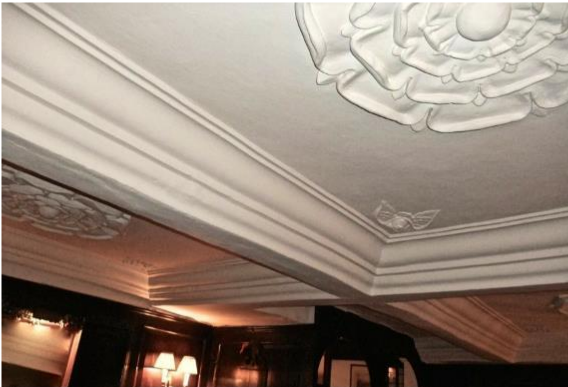
3.70 Ceiling, hall, Old Manor, Combe Florey, Somerset (TA6).
