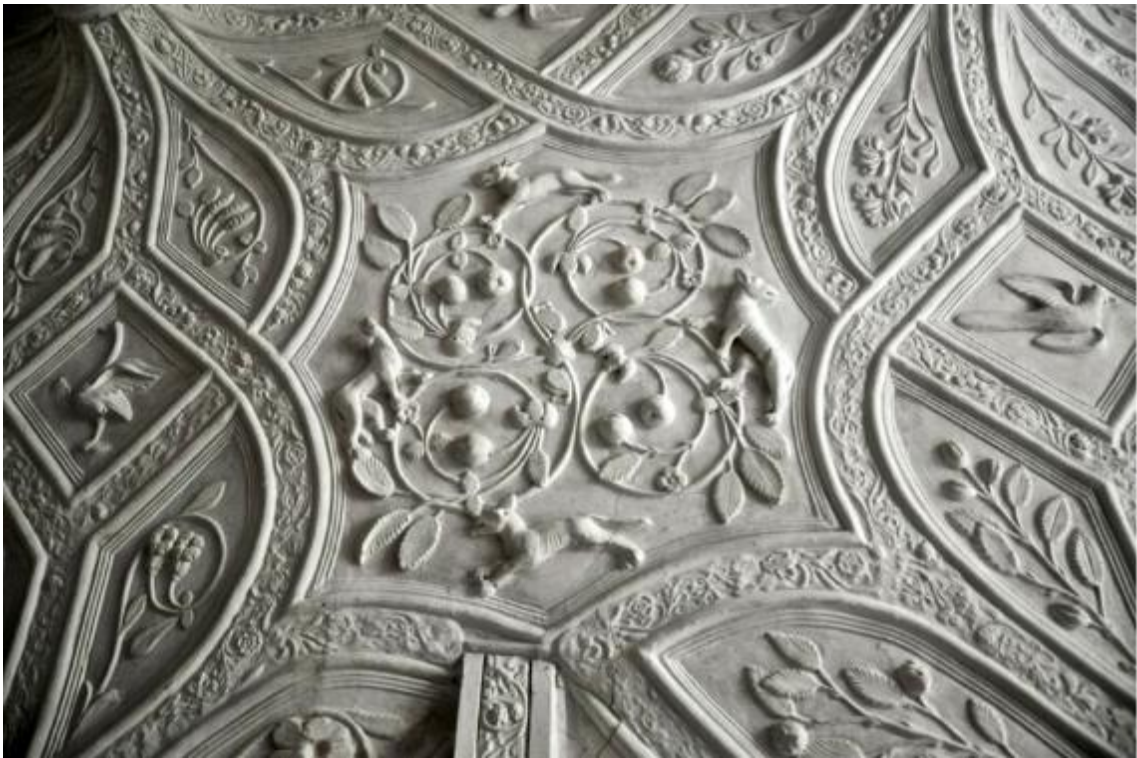
3.77 Ceiling, master chamber, Rashleigh Barton, Devon (MD24).
