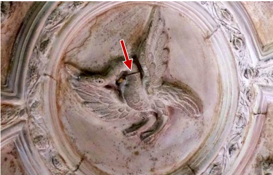
3.12 Wired-in cast, ceiling, gallery, Lanhydrock, Cornwall (CO9).
