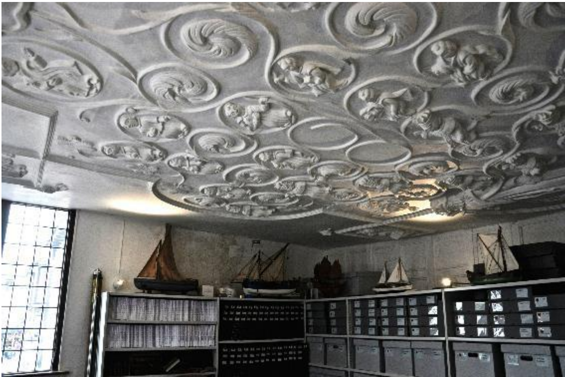
7.41 Ceiling, 12 Duke Street, Dartmouth, Devon (SH9).
