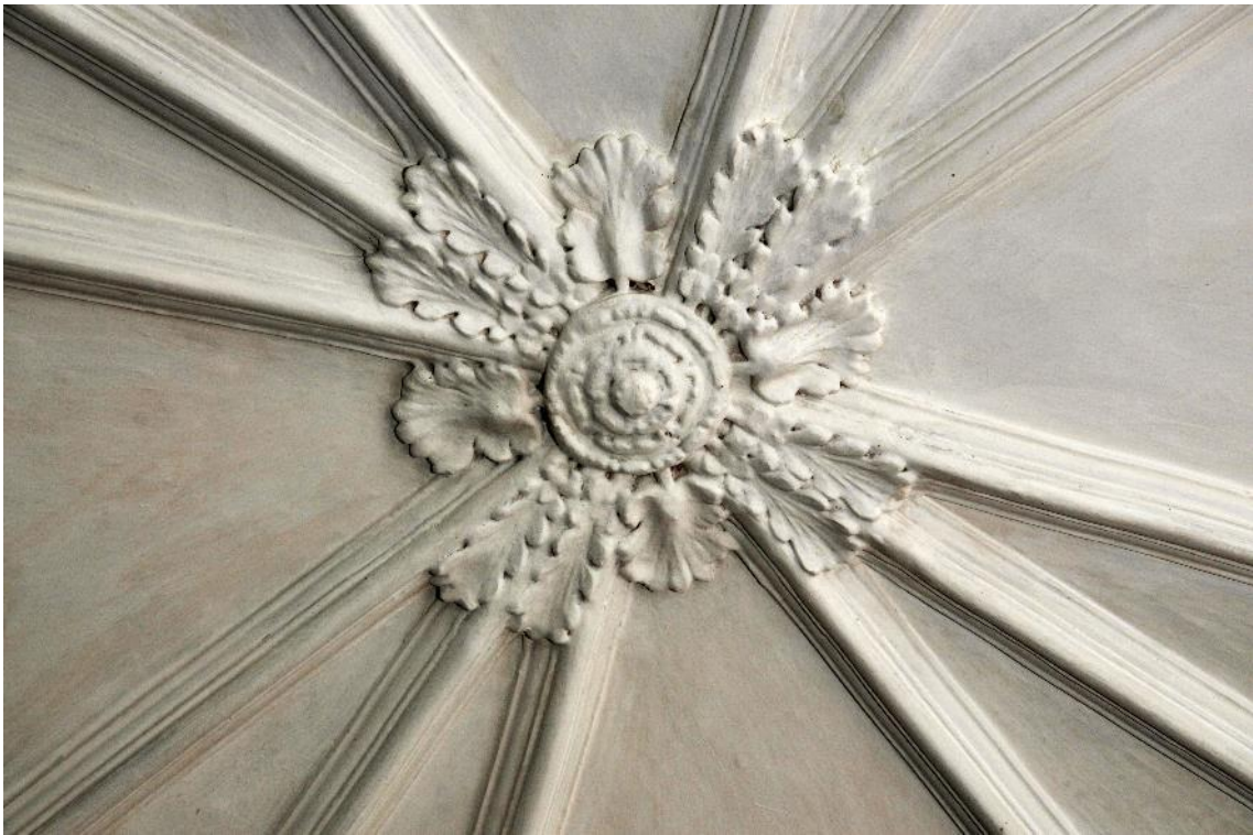
3.15 Ceiling boss, Oak Room Poundisford Lodge (TA23).
