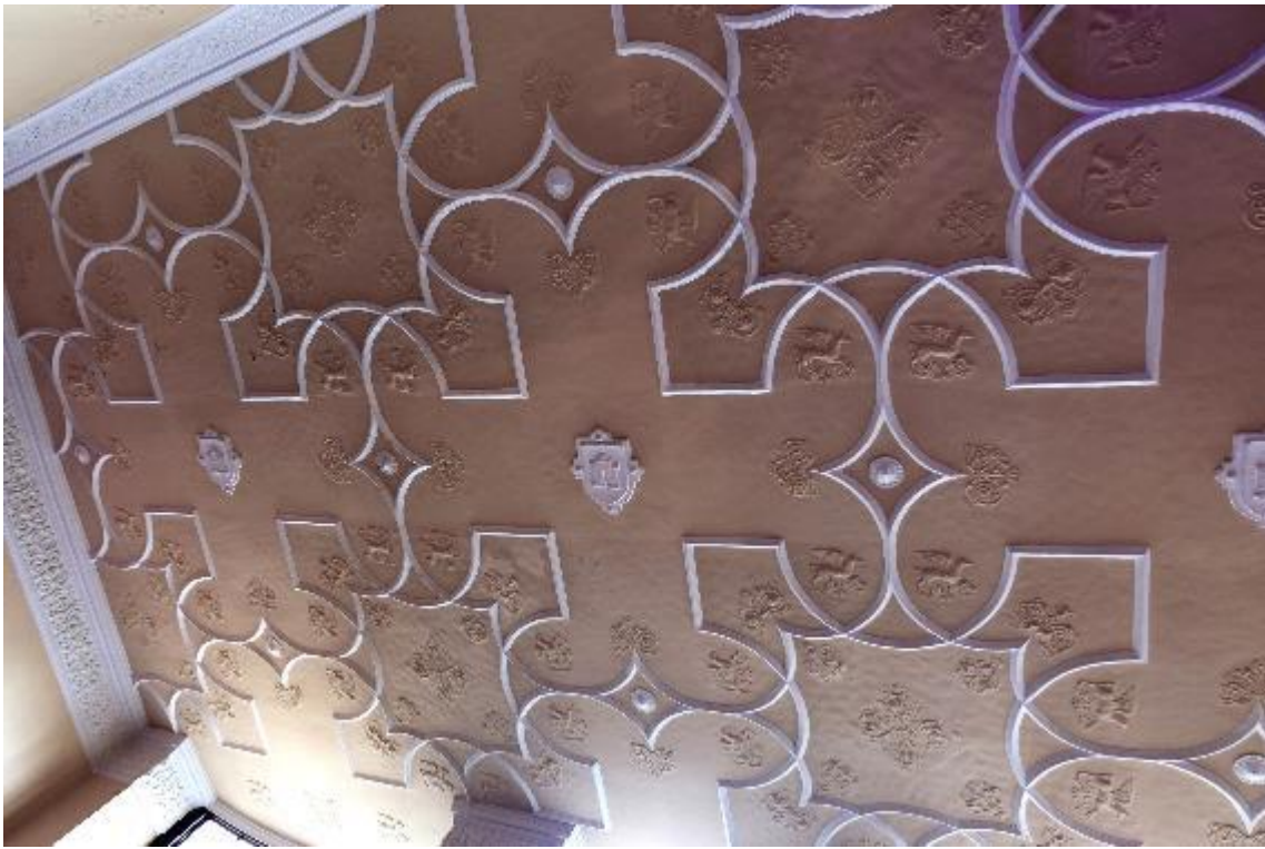
5.25 Front ceiling, 62 Boutport Street, Barnstaple (ND3).
