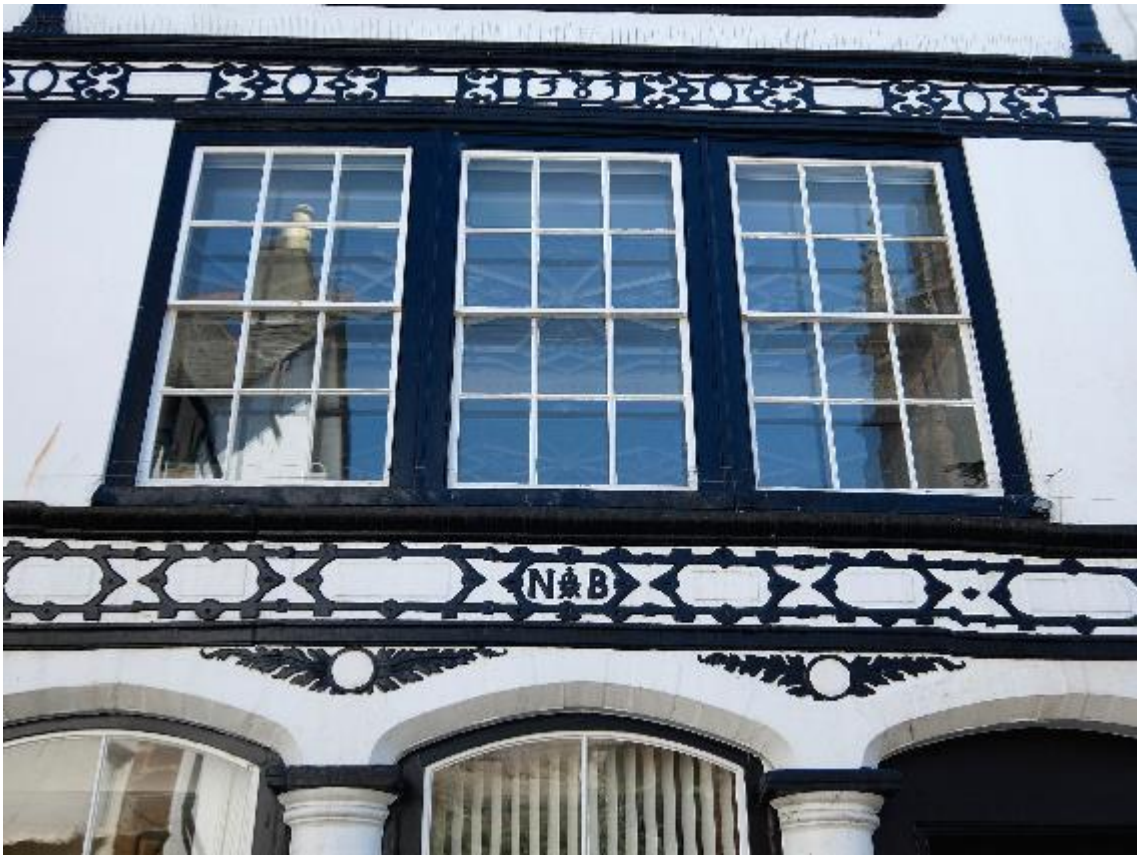
7.37 View from street level, 16 High Street, Totnes, Devon (SH40).
