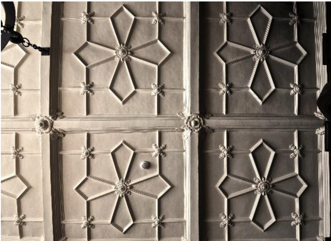
3.18 Ceiling, parlour, Holcombe Court, Devon (MD11).
