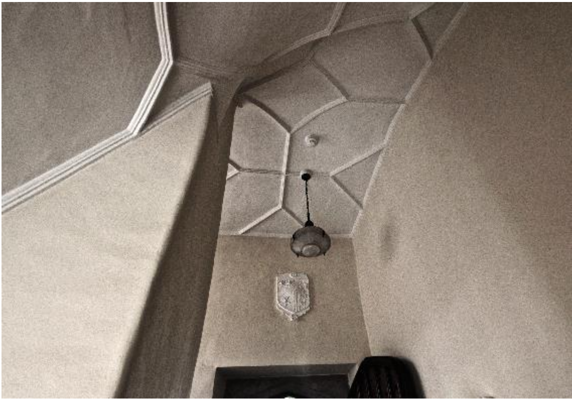
7.29 Stairwell, Holcombe Court, Devon (MD11).
