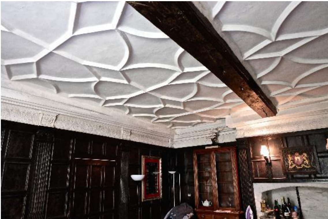
7.13 Ground floor, 10 High Street, Totnes, Devon (SH37).
