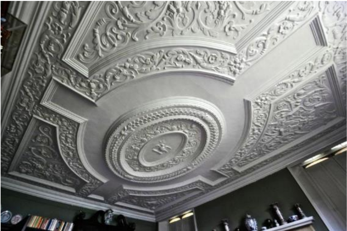
3.30 Ceiling, parlour, Poundisford Park, Somerset (TA24).
