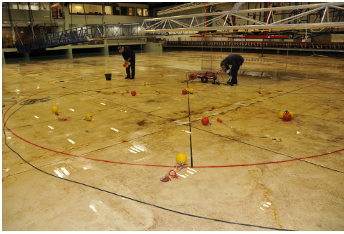
(a) Welding anchor points to tank floor
