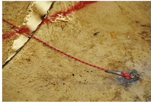
(c) Welded anchor point
