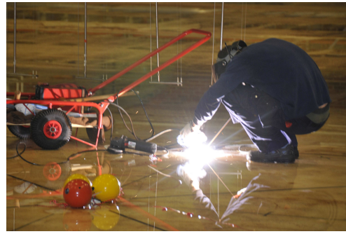
(b) Welding anchor points to tank floor
