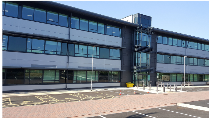
(a) Overview of the building.
