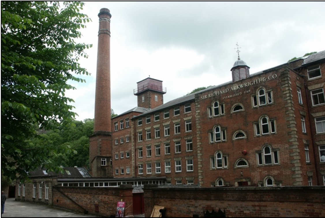
Figure 4.16 Masson Mill front elevation, the central part is the original mill with its venetian windows and a service bay to each end with a cupola above the central bay, the waterwheel was at the rear on the river. The mill was later extended, and the steam engine installed. Photo © Author, 2013.
