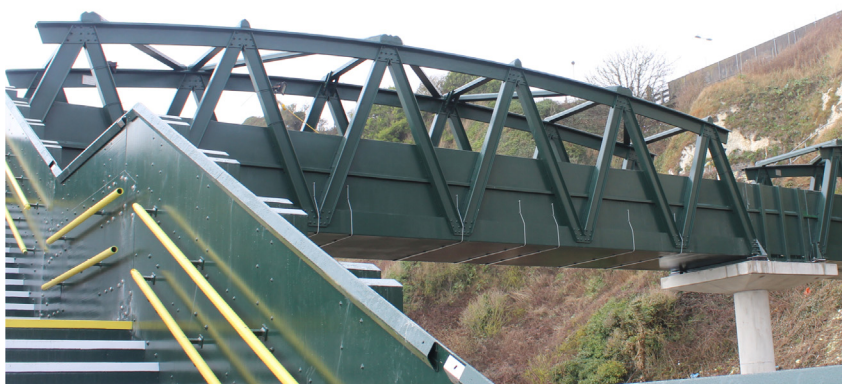
(a) Photograph of the bridge
