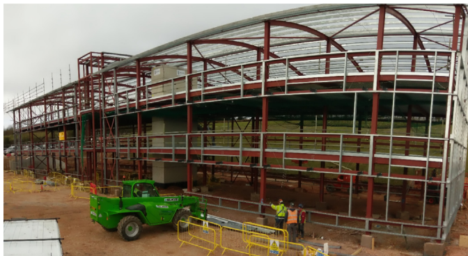
Fig. 8. Panoramic view of the building containing Floor B (The far half of the first floor).
