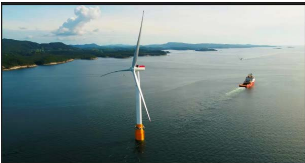
Figure 2 Hywind Towout (courtesy Equinor)
