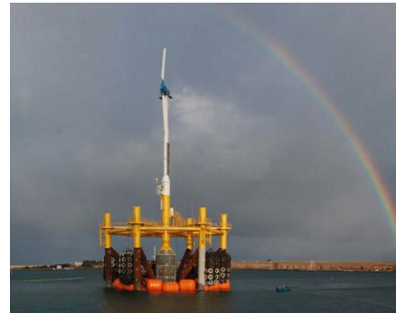
Figure 10 0.08MW TLP (courtesy Blue H)
