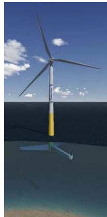
Figure 5 TLP (courtesy Bluewater)
