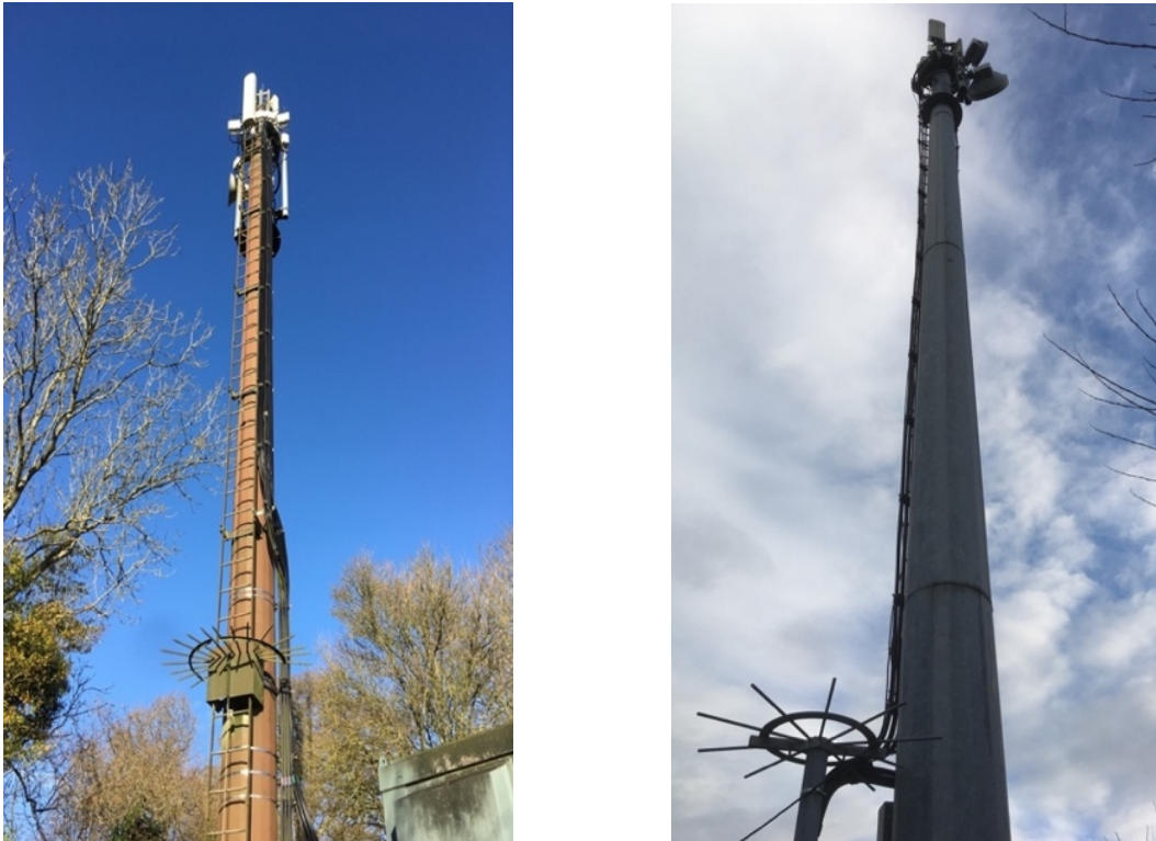
Figure 4-1 Left. F&Li monopole. Right. Portasilo monopole.
