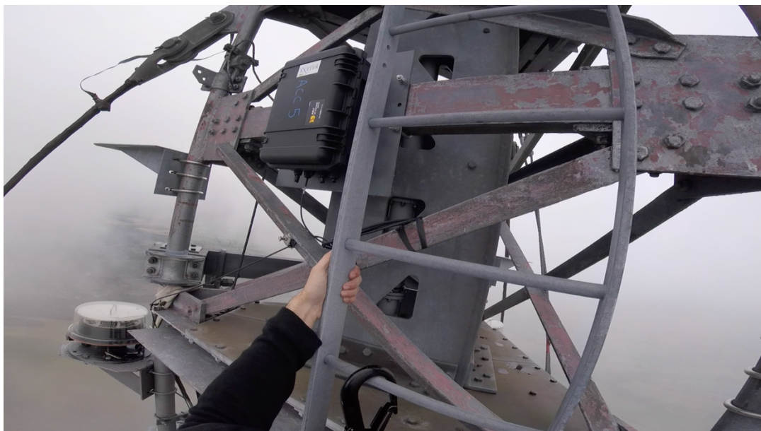
Figure 9-5 Installed position of accelerometer box (ACC5) and anemometer. Picture of accelerometer box (ACC5).
