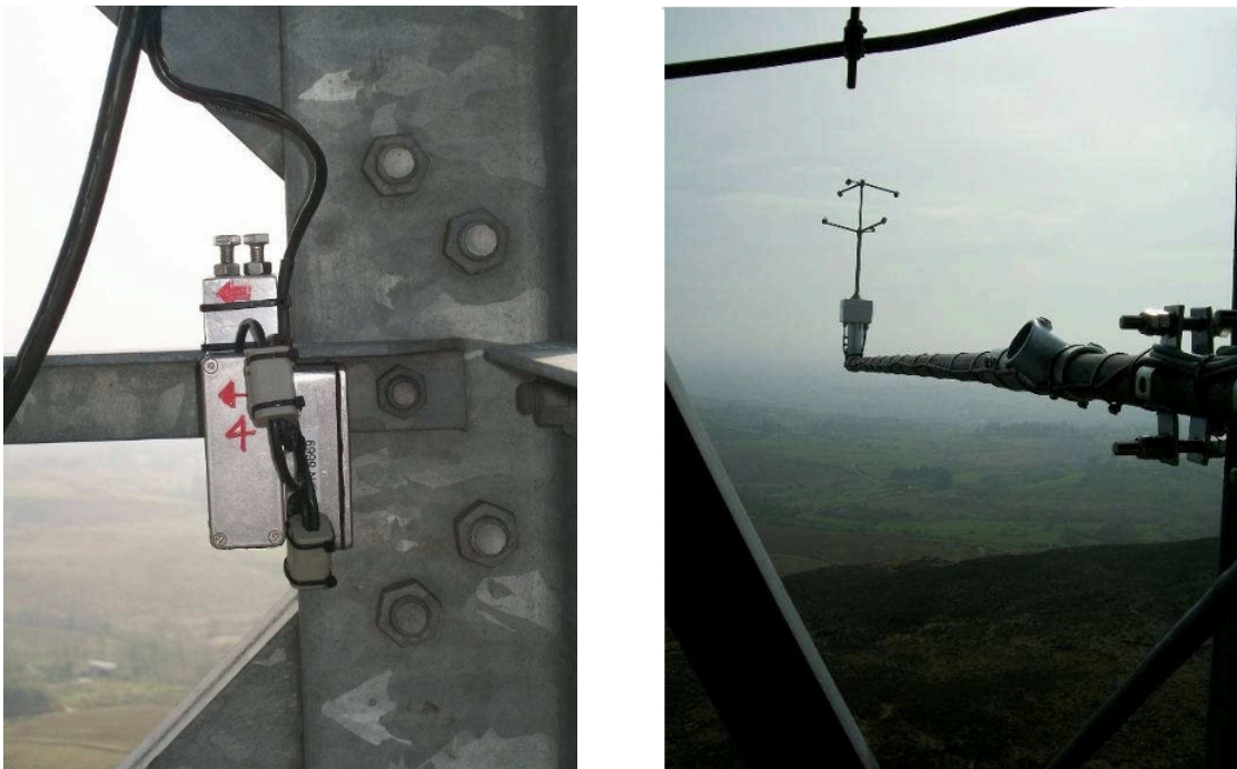
Figure 8-18. Monitoring instrumentation in Brougher Mountain, courtesy of the Strainstall report.
