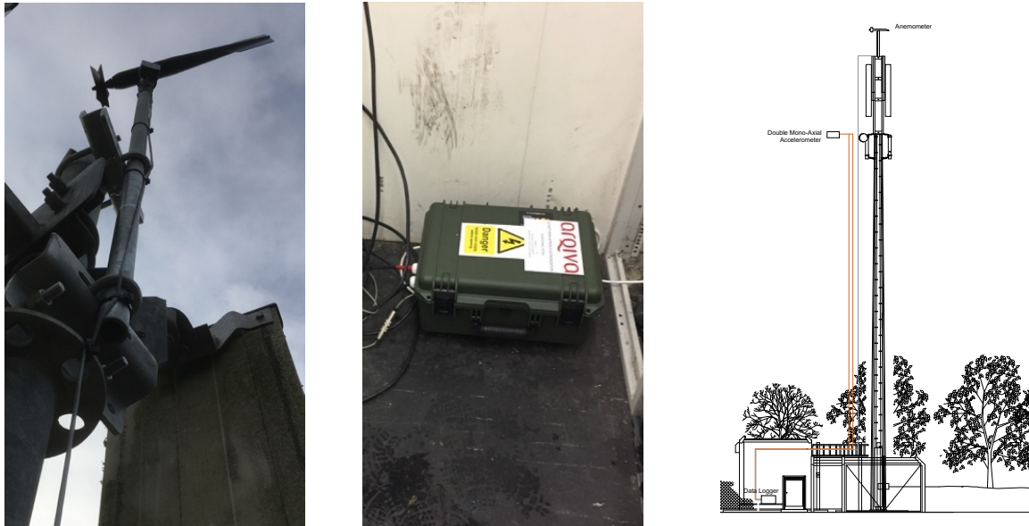
Figure 7-6. Aerodynamic monitoring system. Left: Anemometer installation & Steelwork. Centre: Data logger in Cabin. Right: Monitoring Sketch for St Ives FC.
