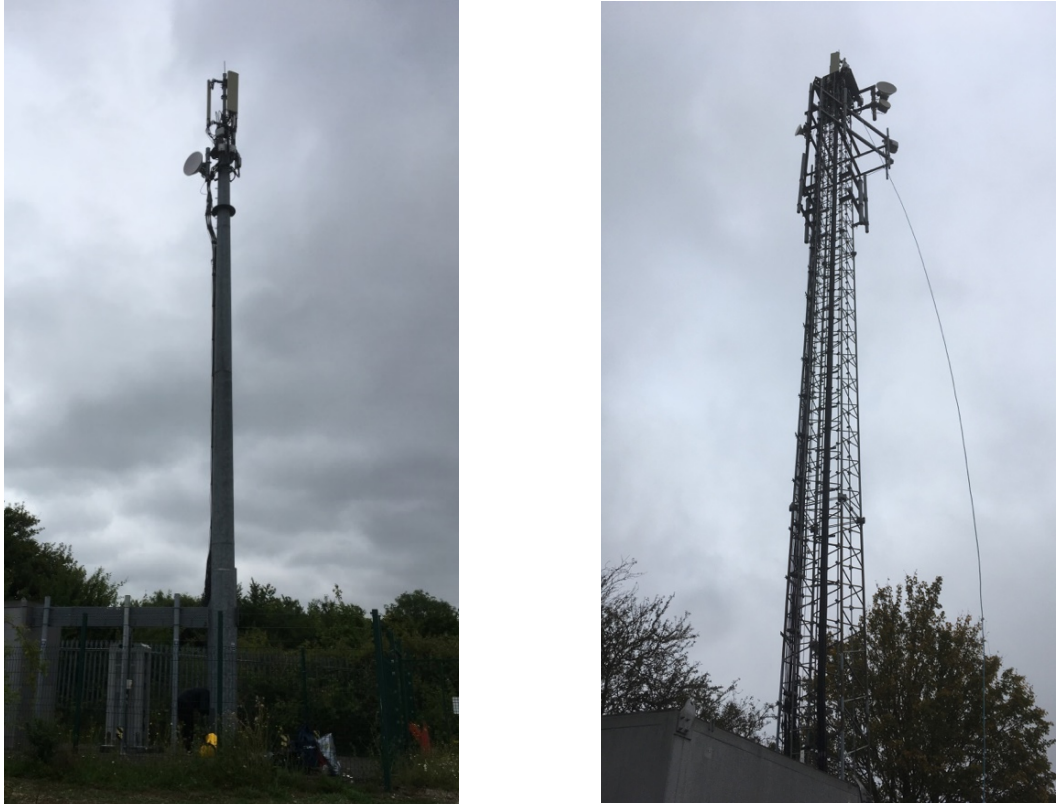
Figure 3-1 Left. Example of a monopole. Right. Example of a short lattice tower.
