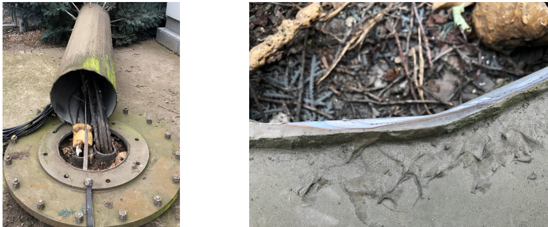
Figure 7-1 Pictures of failed tree monopole in the UK in 2019. Provided by MBNL.
