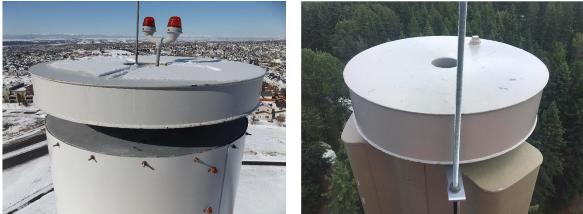
Figure 2-19. Typical TLD in monopoles. Canada [70].
