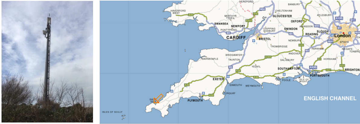
Figure 6-1 (Left) Picture of St Ives FC Portasil monopole. SHM system install. Arqiva. (Right) Location of St Ives in South-West of the UK.
