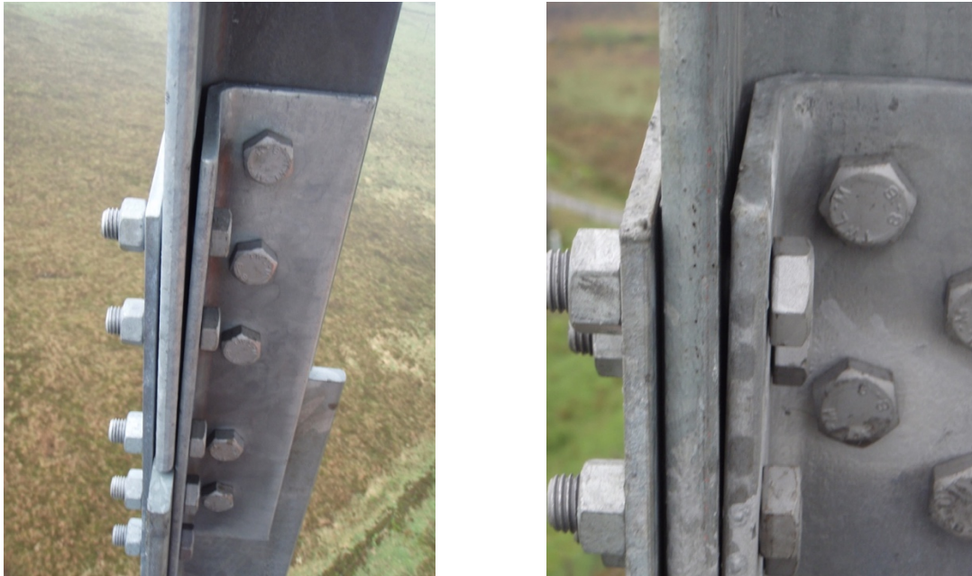
Figure 8-15. Pictures of inspection of leg joints at Brougher Mountain after VS events.
