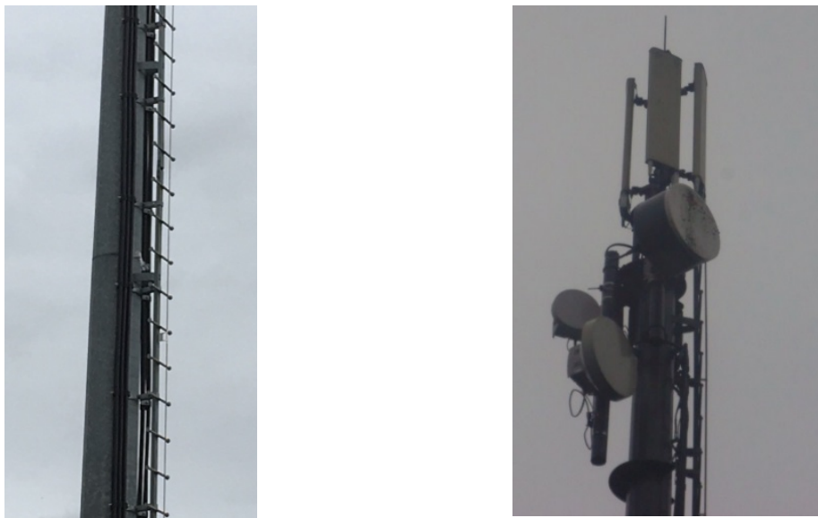
Figure 6-11 Main bending cantilevered modes in St Ives monopole during monitoring. Picture of External cabling and ladder installation.
