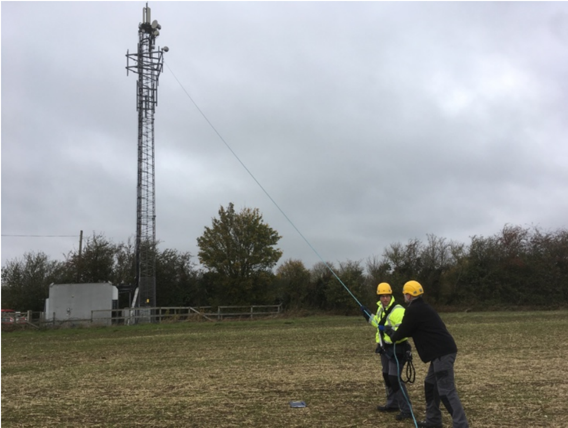
Figure 3-4 Picture of pull application on lattice towers during modal test.
