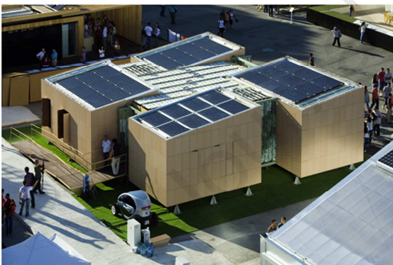
(e) BIPV roof application
