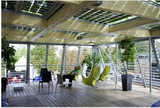
(a) BIPV daylighting application
