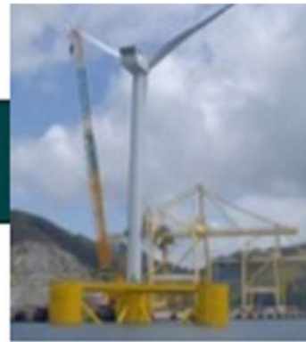
WTG Integration at Quayside
