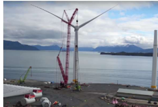
Onshore topside construction
