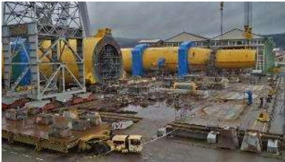
Onshore Construction Of the Substructure
