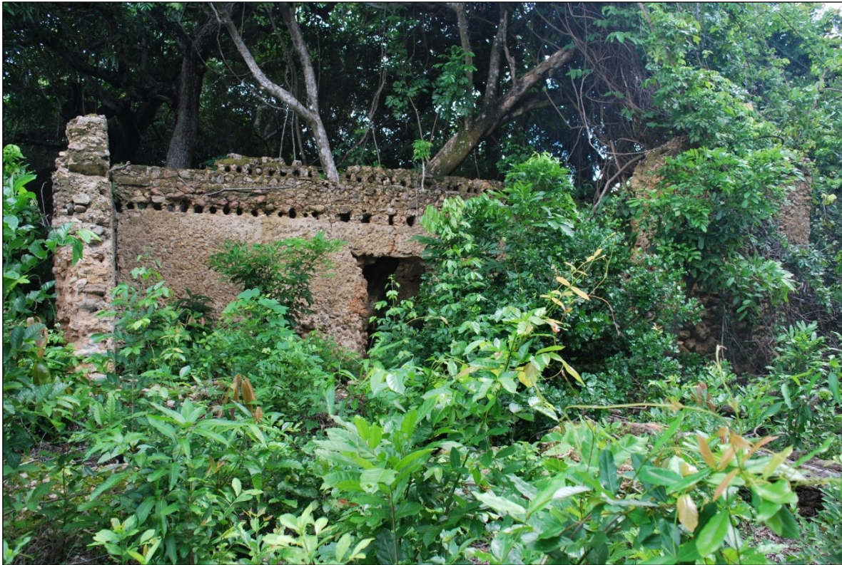
Figure 3.12: Tungi palace facing northwest.
