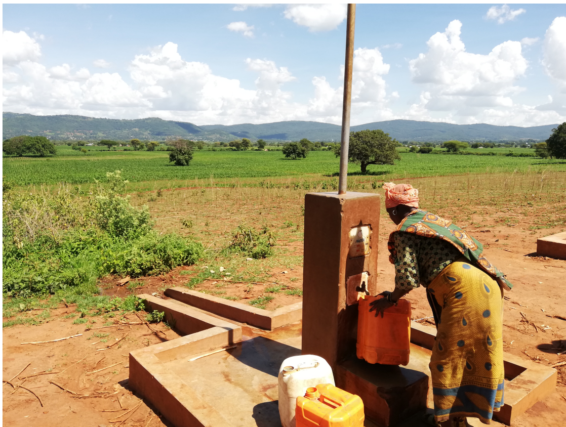
Figure 3.2 eWater tap in use in Tanzania, with solar panel and antennae at the top of the pole. The tag is held on to the top module with a magnet.
