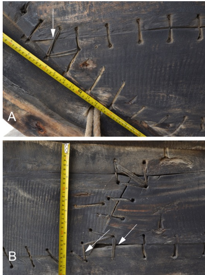
Figure 6.8: Holes without rebates at the corners of hood ends (A) and scarf joints (B) of the QM kettuvallam . (Photo: Author).
