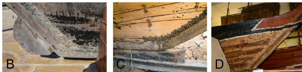
Figure 6.7: Timber Wo98B with a series of holes without rebates (A) suggesting the presence of sections of wadding outside the hull as observed in an Omani kambāri (B) and battil (C) (Photos: Author). The mtepe model at the Science Museum, London (D). (Photo courtesy of Norbert Weismann)
