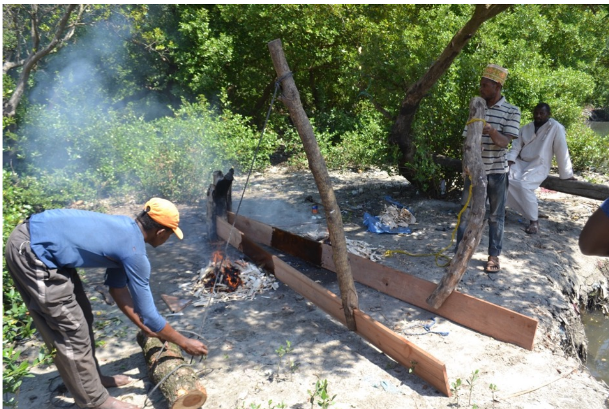
Figure 5.4: Boatbuilders in Zanzibar use controlled fire to bend and twist planks. (Photo: Author)
