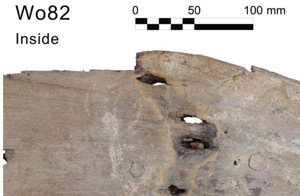
Figure 3.51: Traces of oxidation on the inner surface of plank Wo82, revealing the presence of nails. (Photo: Author).
