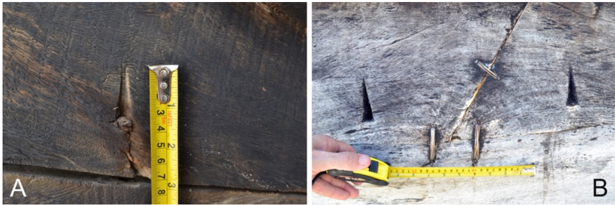
Figure 6.32: Oblique nails recessed in triangular rebates on the hull of QM kettuvallam (A). Zanzibari boatbuilders have combined this fastening technique with discrete lashings on a vernacular ngalawa (B). (Photos: Author).
