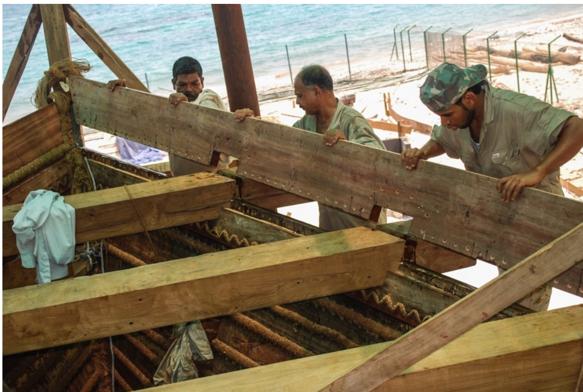
Figure 5.10: Fitting the plank above the through-beams on Jewel of Muscat . The top and bottom strakes, and the beams are notched to accommodate each other. (Photo: Author)
