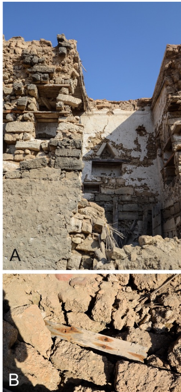
Figure 7.10: Abandoned buildings in Mirbat, southern Oman (A). Most of the timber used for shelves and beams was recycled from boats (B). (Photos: Author)
