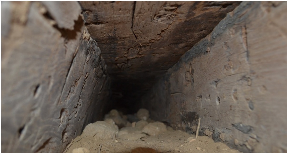
Figure 6.30: The edges of timbers Wo98C (left plank) and Wo98A (right plank) lined with bitumen. (Photo: Author)
