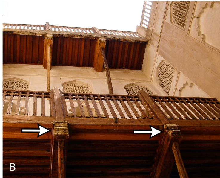
Figure 7.9: A balcony in the internal courtyard at Jabrin castle, supported by beams with decorated ends. (Photo: Author)
