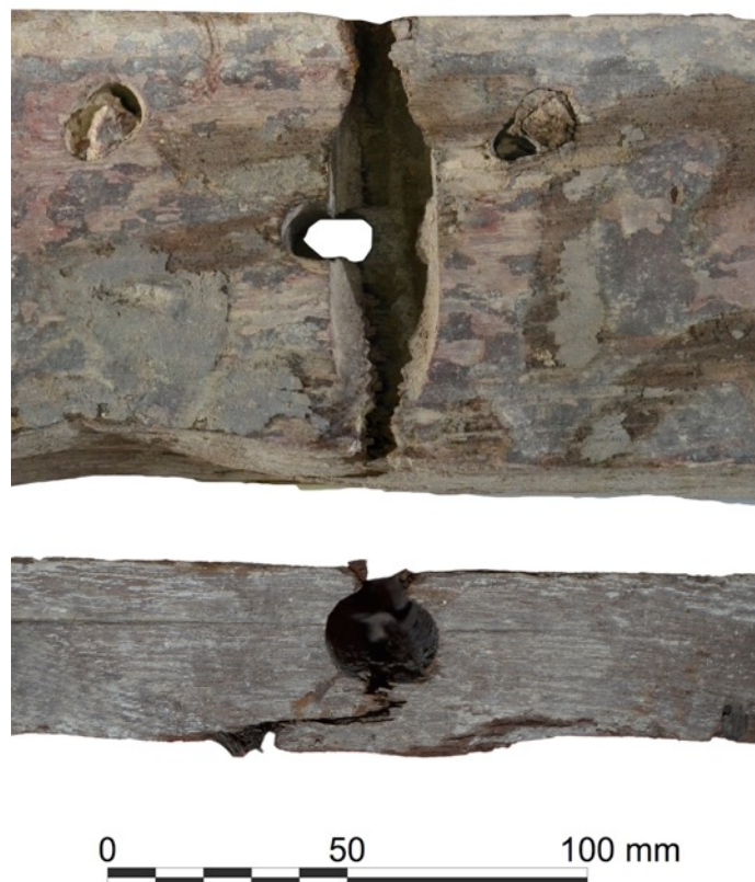
Figure 3.32: A large crack caused by a dowel on Wo56-Wo60. (Photo: Author).
