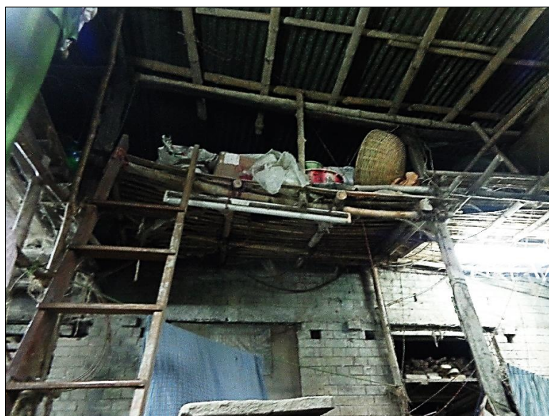
Figure 6.5: A loft in the workshop (source: author)
