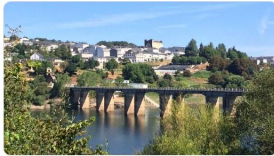
Figure 141: Portomarín, a bridge too far
