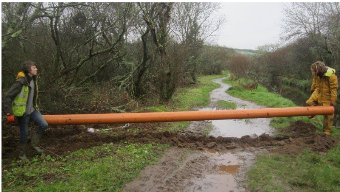
Figure 22: Photograph of pipe laying into the Willow Carr
