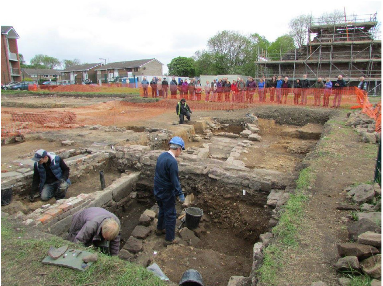
Figure 2: Aside from the volunteers taking part in excavations, the Radcliffe Tower project drew significant interest from the local community
