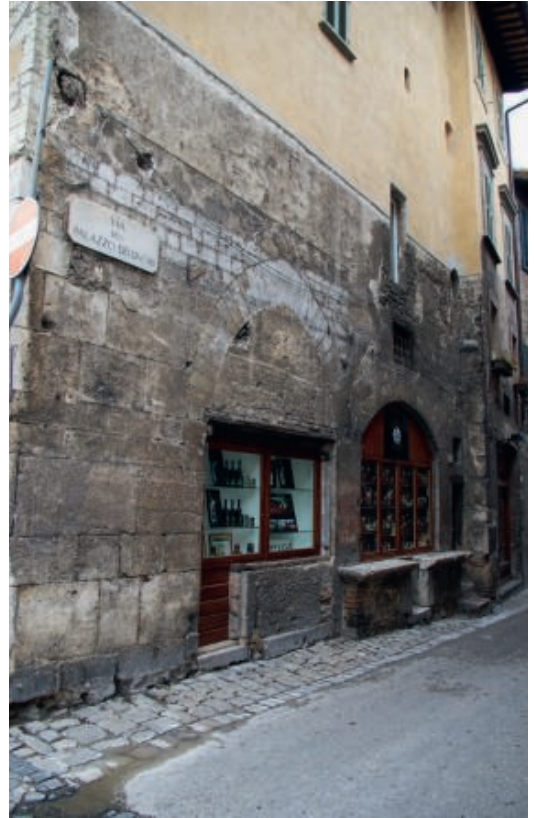
83. Shops on via del Palazzo dei Duchi, Spoleto. They were created from chapels remaining after the demolition of the church of San Donato in the 16th century.
