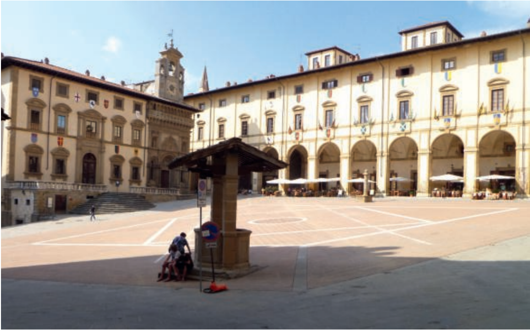
96. The headquarters of the Fraternita dei Laici (left), 1484, and the Loggia Vasari (right), from 1570, piazza Grande, Arezzo.
