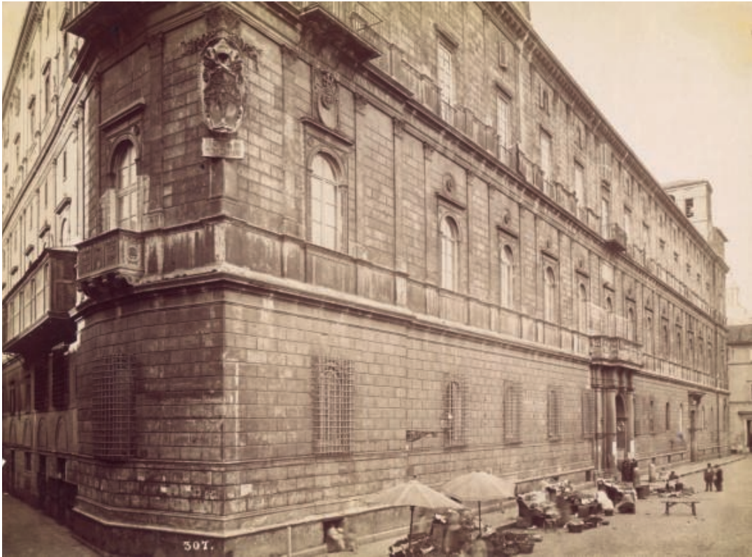
80. Palazzo Cancellaria, from the corner of via dei Pellegrini, Rome. Photograph from the second half of the 19th century.
