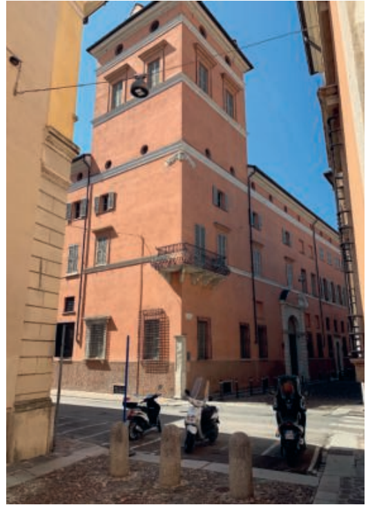
15. Palazzo Arrivabene, Mantua. A candlestick pilaster, dated 1481, adorns the corner of the building, recording its construction.
