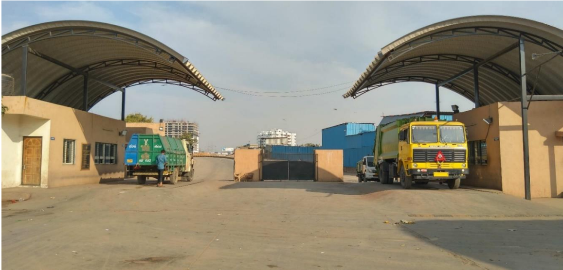
Fig. 22: At the 400 MT-capacity RTS in Wadaj (West Zone), Ahmedabad. Two vehicles stand on weighing scales for digitised measurements conducted at the 'site-offices' on either side. On the left, stands an incoming door-to-door waste collection vehicle – one with the smallest capacity denomination (1 MT), with separate chambers for dry and wet waste. On the right is a larger outgoing vehicle of 20 MT capacity, expected to be filled exclusively with dry materials, headed for the WTE plant. The RTS acts as a key techno-logistical point of localisation and transfer of separate streams of materials toward different processing sites and networks. Courtesy: Author
